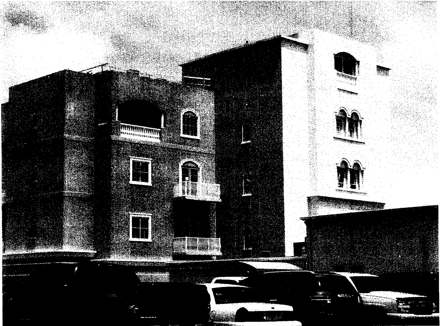
Front View (Looking Southeast) Photo Date 6/24/11
