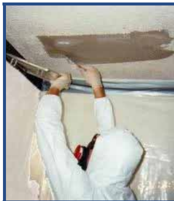
Licensed asbestos abatement worker removing asbestos-containing ceiling
