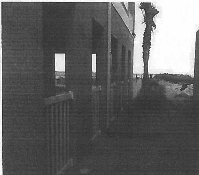
RIGHT SIDE (NORTH) VIEW 8/19/2015
