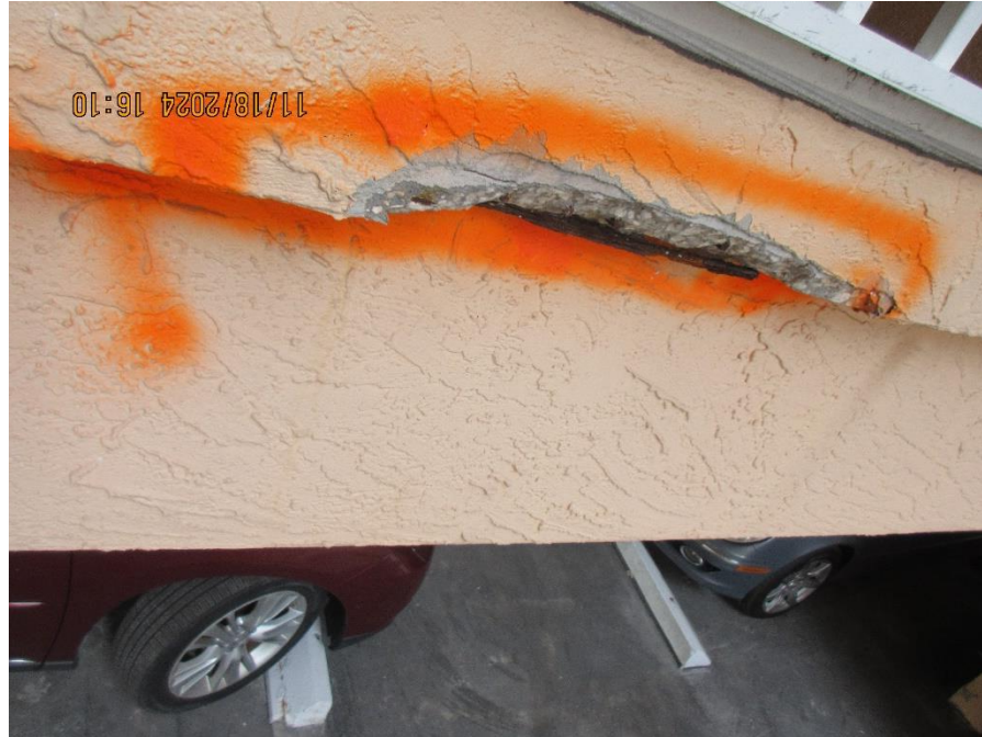
Photo #19 – Concrete Spall with Exposed Reinforcement at Slab Edge of Elevated Balcony, (Building I).
