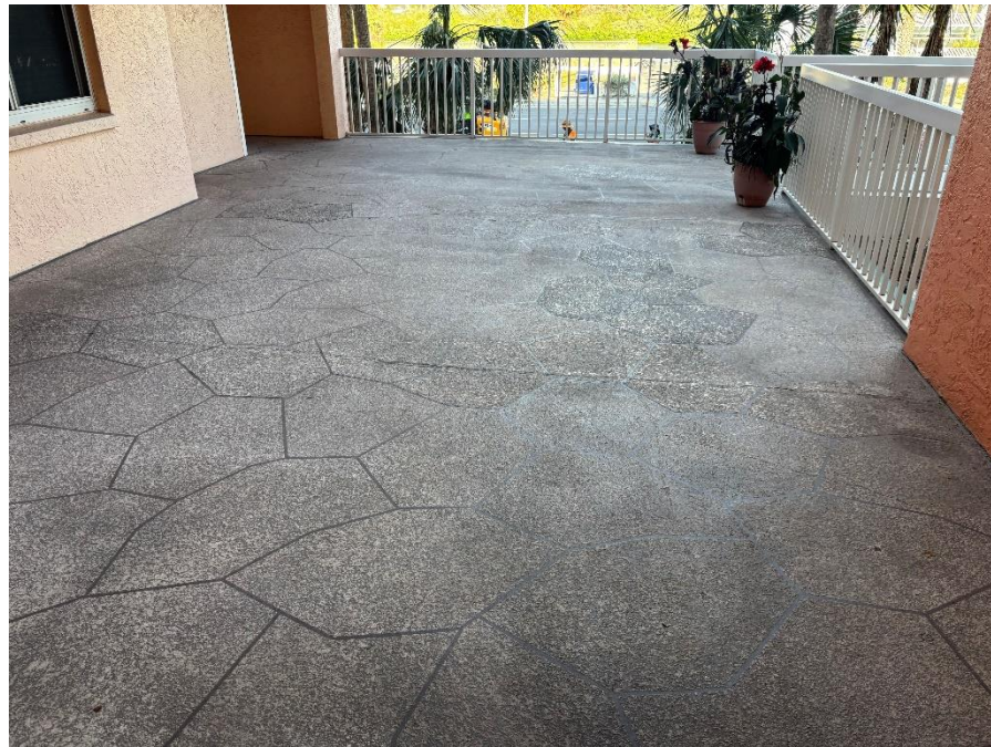
Photo #24 – Stained Deck Coating (1 st Floor - Building II)
