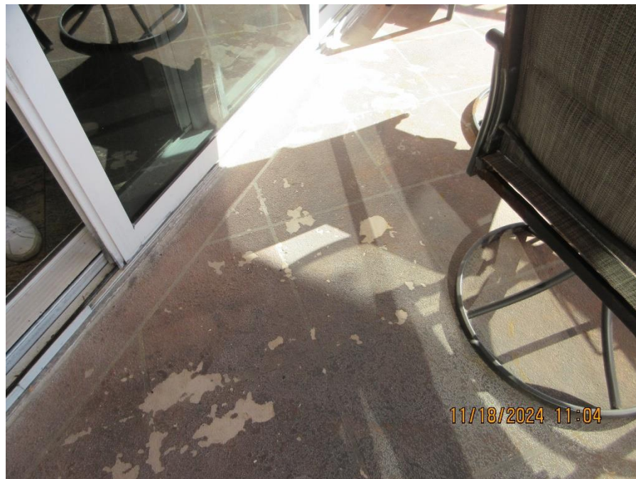
Photo #14 – Deck Coating Finish Peeling at Balcony.
