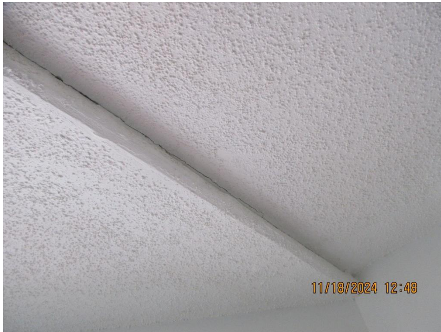
Photo #26 – Typical Transition Between Precast Panels at Unit Interior - Beach Cottage II.
