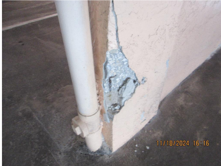
Photo #21 – Typical Concrete Spalls at Columns in Under-building Parking Garage.
