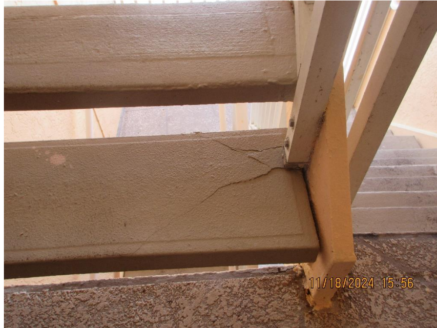
Photo #17 – Cracked Stair Threads (North stair tower 1 st , 2 nd , 3 rd + S stair tower 1 st floor – Building I)
