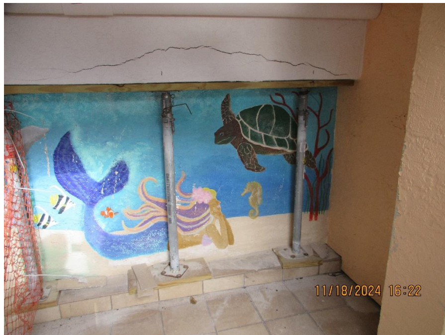
Photo #20 – Concrete Crack at Beam Under Pool Deck Area - Under Repair.
