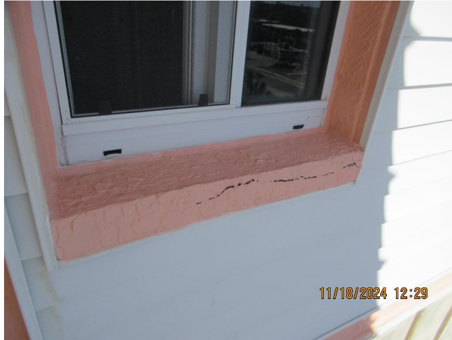
Photo #13 – Crack at Pre-Cast Concrete Window Sill. (TYP.)
