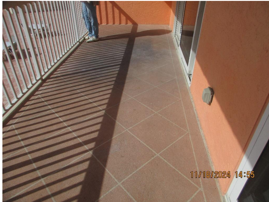
Photo #15 – Typical Stained Balcony Deck w/ Possible Ponding Area.
