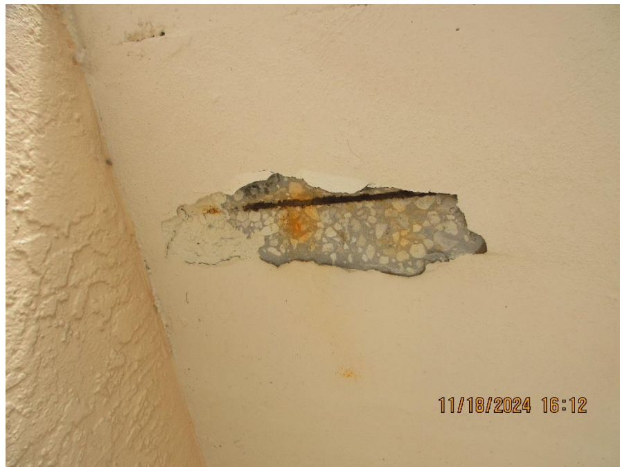
Photo #18 – Typical Concrete Spall w/ Exposed Reinforcement at Building I Under-building Parking.
