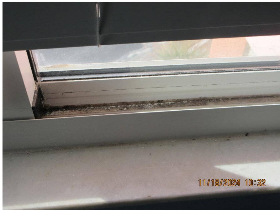
Photo #12 – Possible Sign of Condensation and Suspected Microbial Growth at Windows of Unit #2501.
