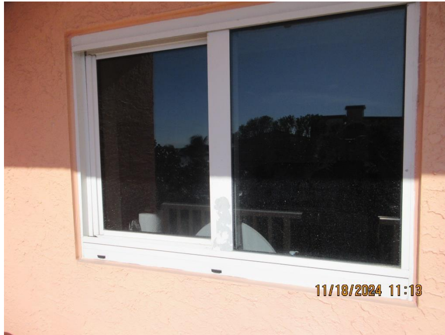
Photo #11 – Sealant Bead Around Exterior Window Perimeter at Elevated Walkways in Good Condition. (TYP)
