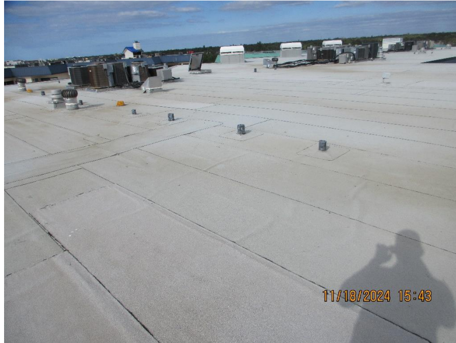
Photo #7 – Typical Overview of Modified Bitumen Roof Systems with HVAC Units @ Beach Cottage I.
