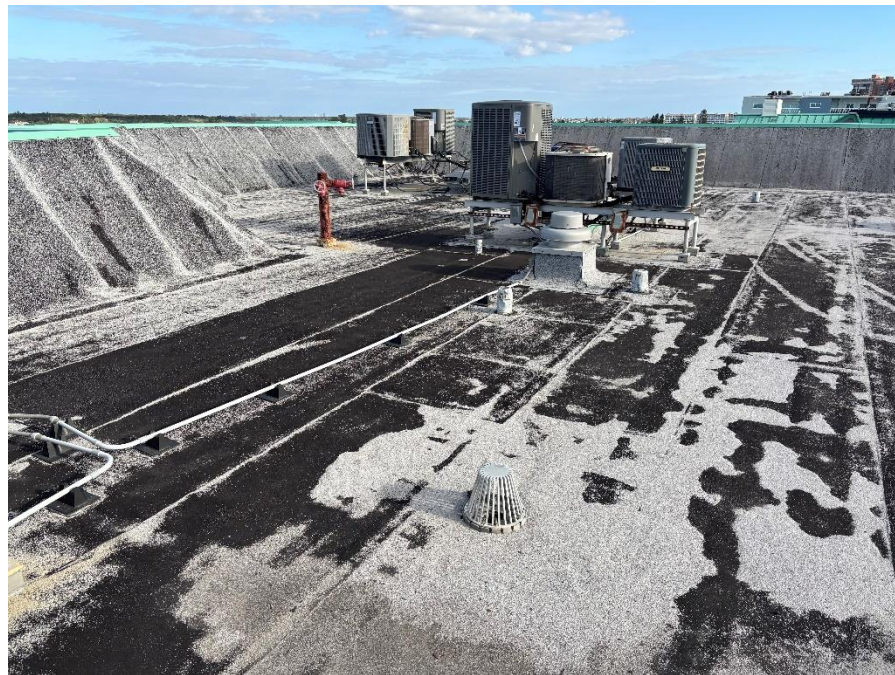
Photo #8 – Typical Overview of Modified Bitumen Roof Systems with HVAC Units at Beach Cottage II.
