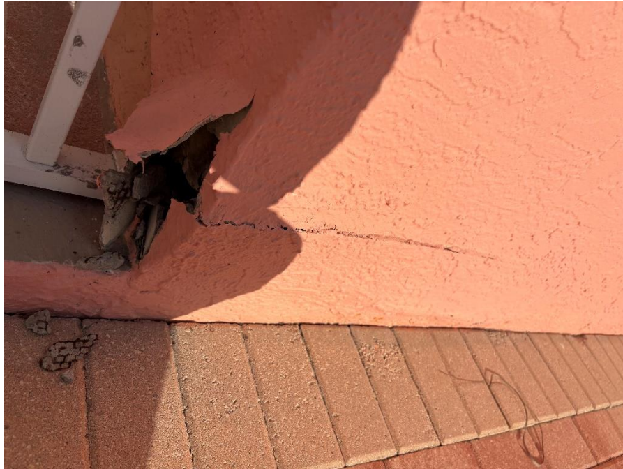
Photo #25 – Delaminated and Cracked Stucco at 1 st Floor at Pool Deck. (W Elevation - Building II)
