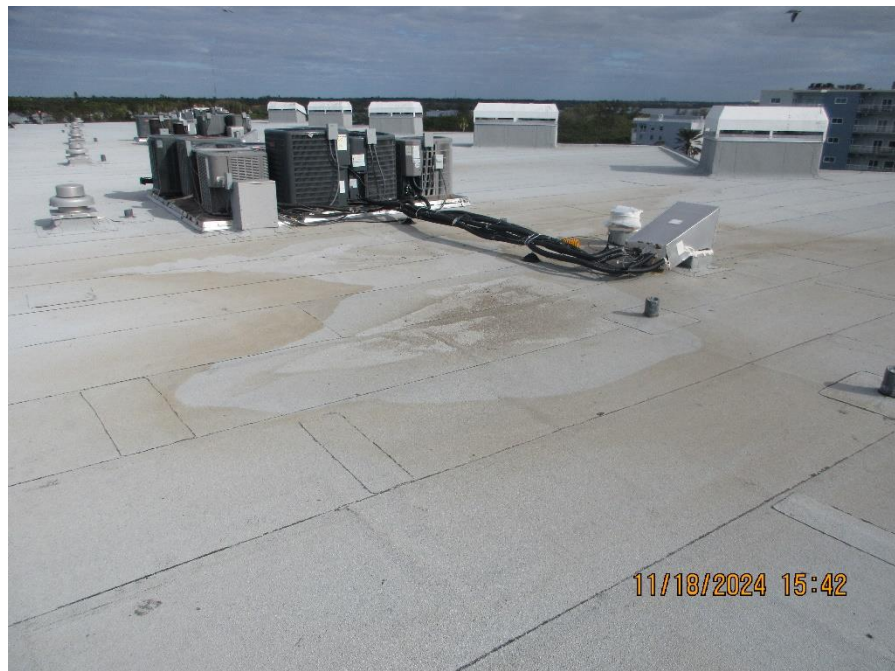
Photo #16 – Sign of Mild Water Ponding on Roof at Building I, Periodic Maintenance Recommended.
