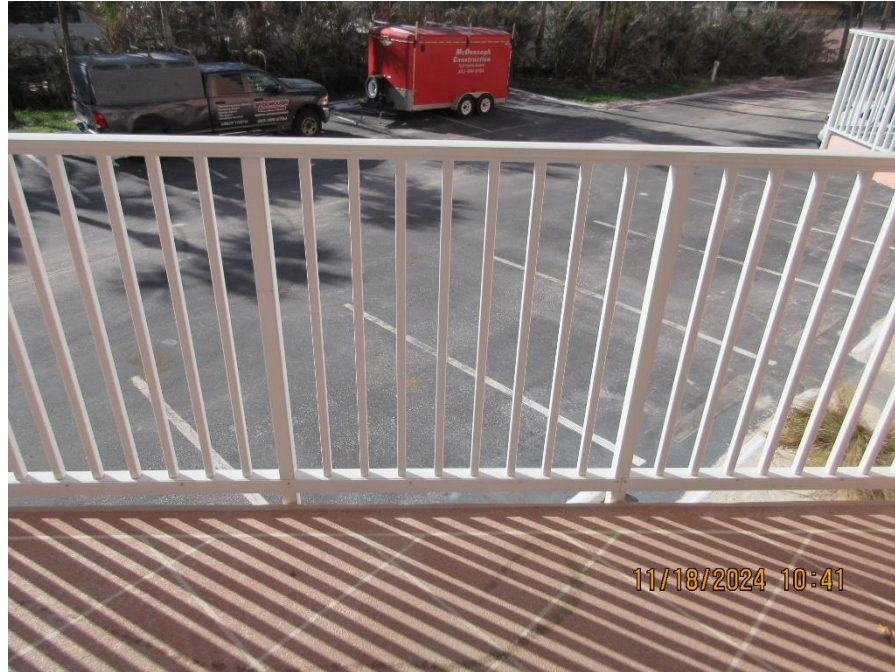
Photo #9 – Typical Code-Compliant Railings at Balconies and Elevated Walkways. (42 ½" in height – 3 ½" in picket's spacing).
