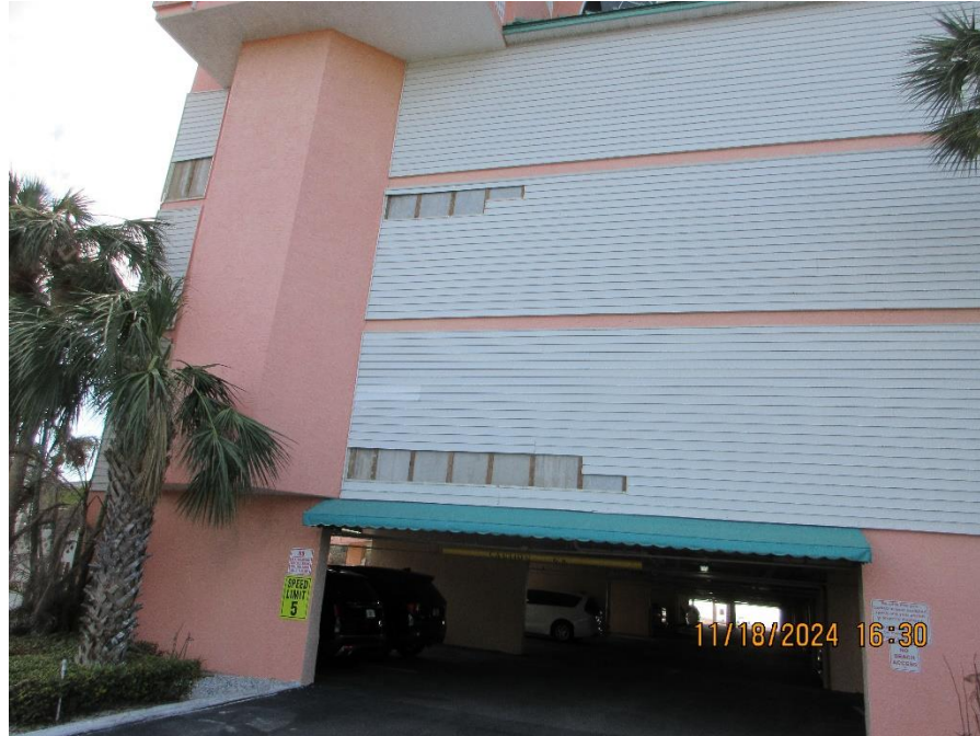
Photo #23 – Typical Missing Vinyl Siding at Both Building's Elevations, from Recent Hurricanes.
