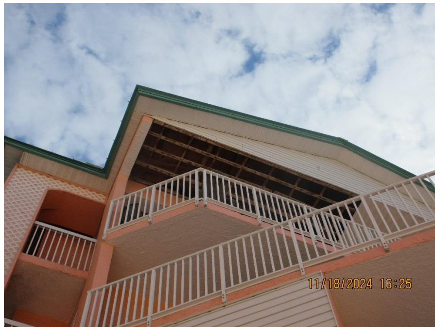
Photo #22 – Typical Missing Soffit at Roofs of Both Buildings, damaged during recent hurricanes.
