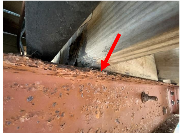
Photo 22 Building 4 – West Elevation – Overall view of corroded exterior steel supports.
