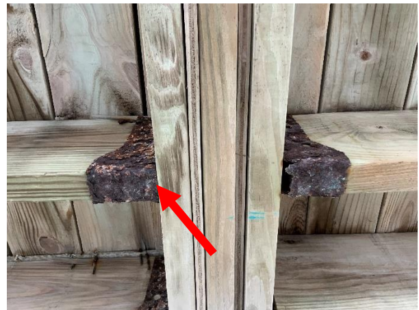
Photo 11 Building 4 – West Elevation – Overall view of corroded joist hangers.
