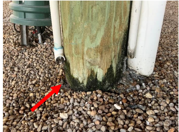
Photo 40 Building 6/7 – North Elevation – Overall view of staining and microbial growth at piling base.
