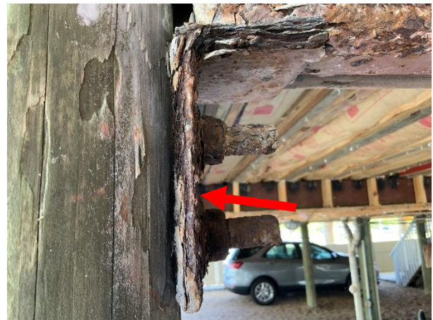
Photo 17 Building 6/7 – South Elevation – Overall view of corroded L brackets.
