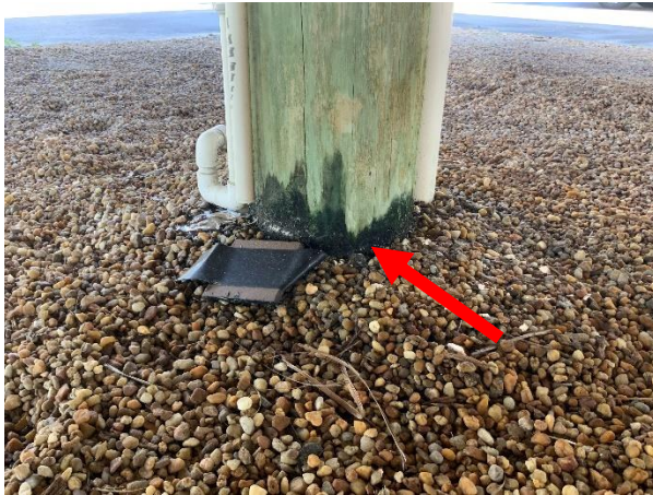
Photo 37 Building 4 – North Elevation – Overall view of staining and microbial growth at piling base.
