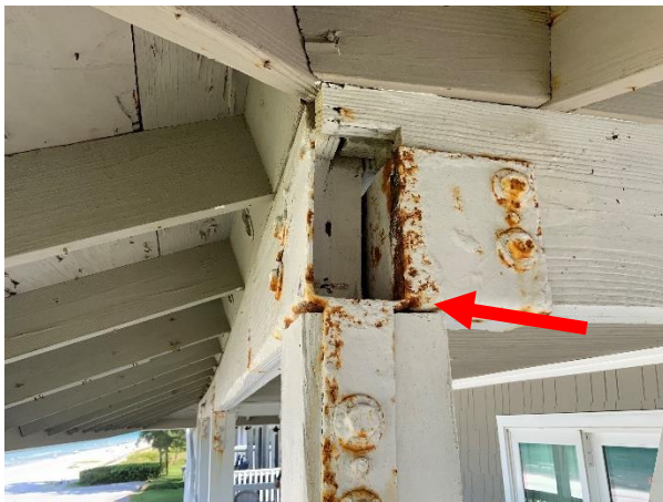
Photo 50 Building 1 – West Elevation – Overall view of corroded metal balcony brackets.
