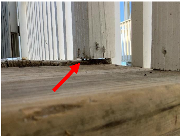
Photo 2 Building 1 – North Elevation – Overall view of unsecured balcony railing post.
