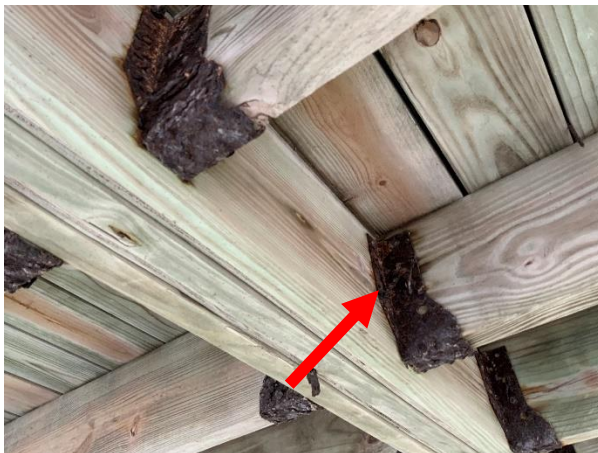
Photo 9 Building 5 – West Elevation – Overall view of corroded joist hangers.
