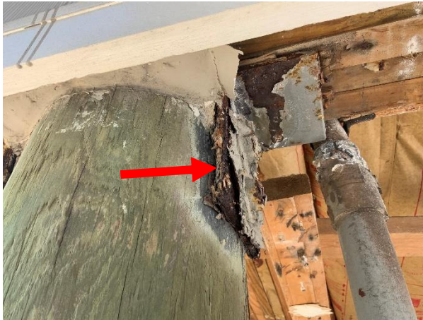
Photo 13 Building 2 – South Elevation – Overall view of corroded L brackets.
