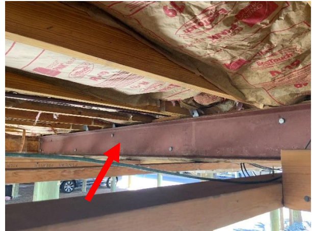
Photo 28 Building 5 – South Elevation – Overall view of corroded interior steel supports.
