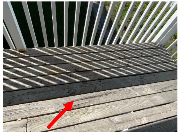
Photo 5 Building 1 – South Elevation – Overall view of deteriorated decking.
