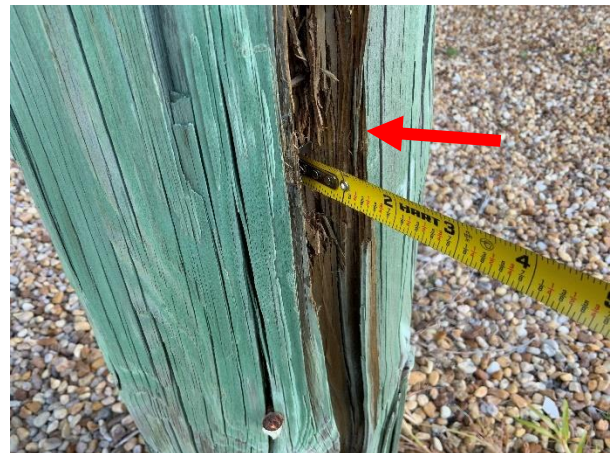
Photo 35 Building 3 – West Elevation – Overall view of approximately 1" of compromised wood.
