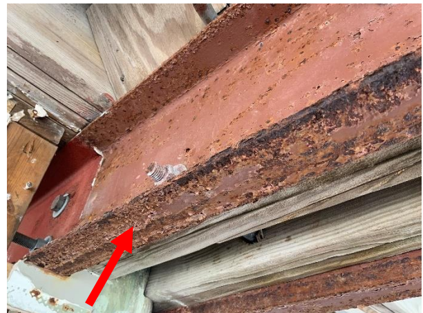
Photo 23 Building 5 – West Elevation – Overall view of corroded exterior steel supports.
