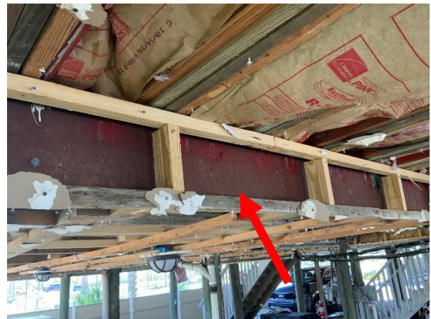
Photo 30 Building 8/9 – North Elevation – Overall view of corroded interior steel supports.
