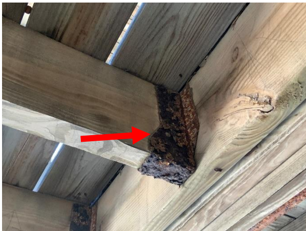
Photo 8 Building 1 – West Elevation – Overall view of corroded joist hangers.
