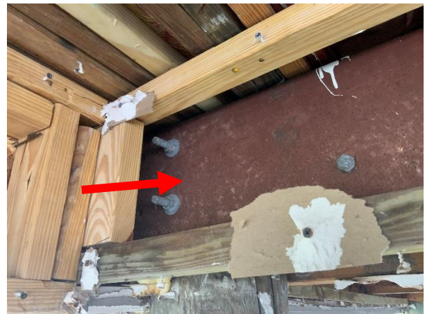
Photo 29 Building 8/9 – North Elevation – Overall view of corroded interior steel supports.
