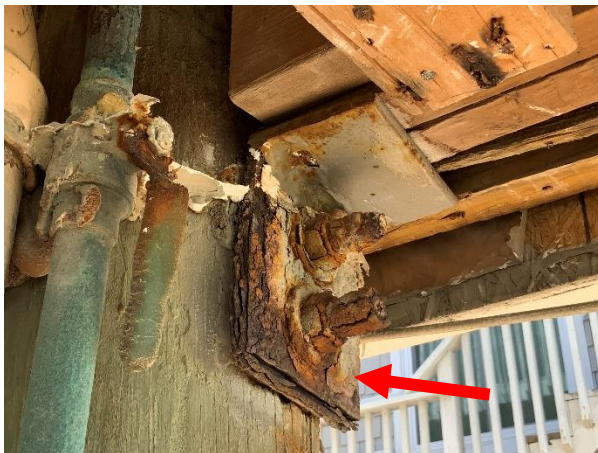
Photo 14 Building 3 – South Elevation – Overall view of corroded L brackets.
