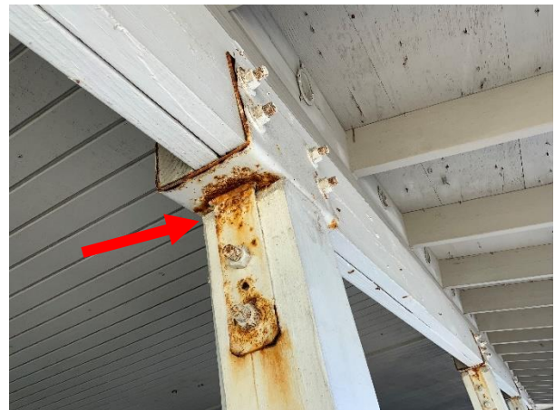
Photo 53 Building 1 – West Elevation – Overall view of corroded metal balcony brackets.
