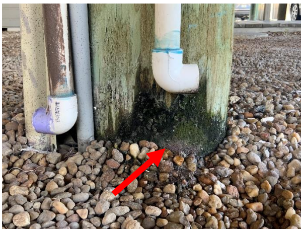
Photo 39 Building 6/7 – North Elevation – Overall view of air conditioning condensation lines at the piling base.
