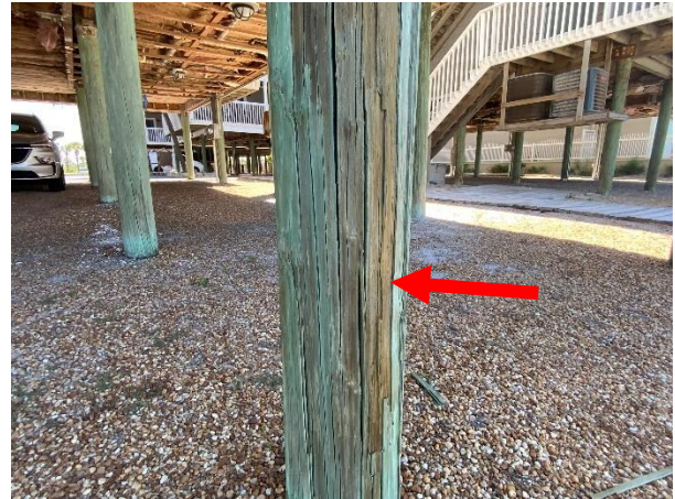
Photo 34 Building 2 – West Elevation – Overall view of splitting piling.
