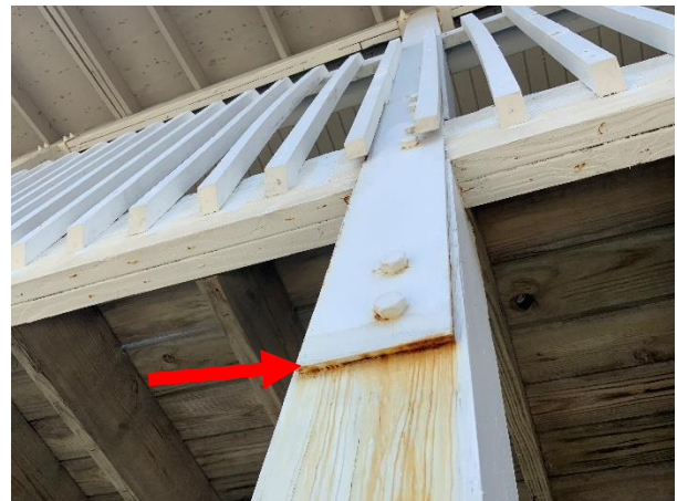
Photo 54 Building 7/8 – West Elevation – Overall view of corroded metal balcony brackets.
