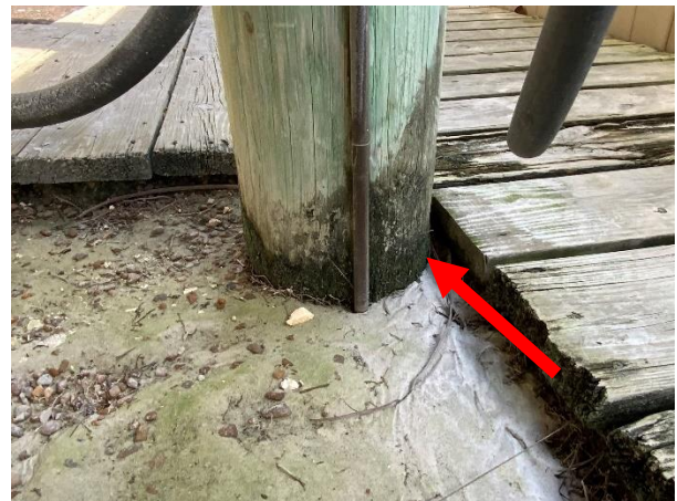
Photo 41 Building 6/7 – East Elevation – Overall view of staining and microbial growth at piling base.
