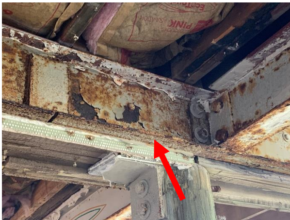
Photo 21 Building 3 – West Elevation – Overall view of corroded exterior steel supports.
