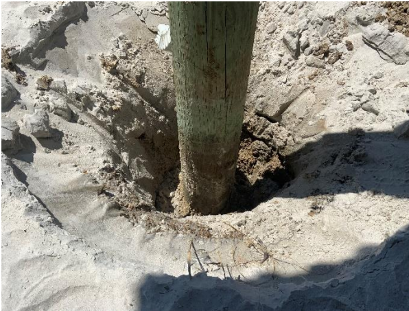
Photo 43 Building 3 – West Elevation – Overall view of excavation at piling base.
