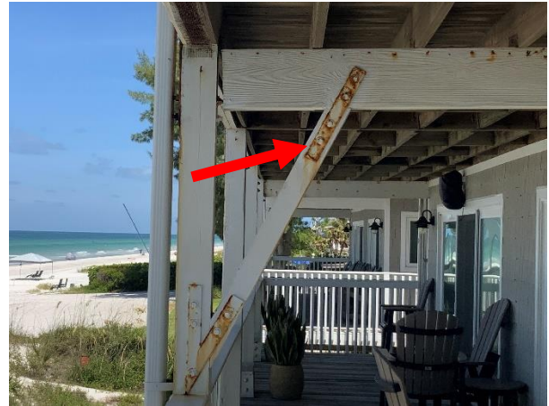
Photo 52 Building 2 – South Elevation – Overall view of corroded metal balcony brackets.
