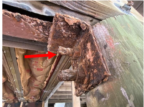
Photo 16 Building 6/7 – West Elevation – Overall view of corroded L brackets.
