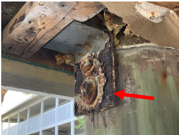
Photo 15 Building 4 – West Elevation – Overall view of corroded L brackets.
