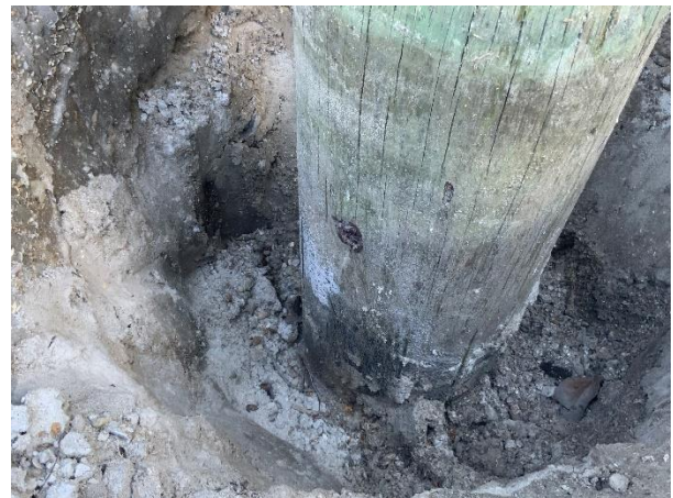
Photo 47 Building 4 – West Elevation – Overall view of sealant applied to piling core sample.
