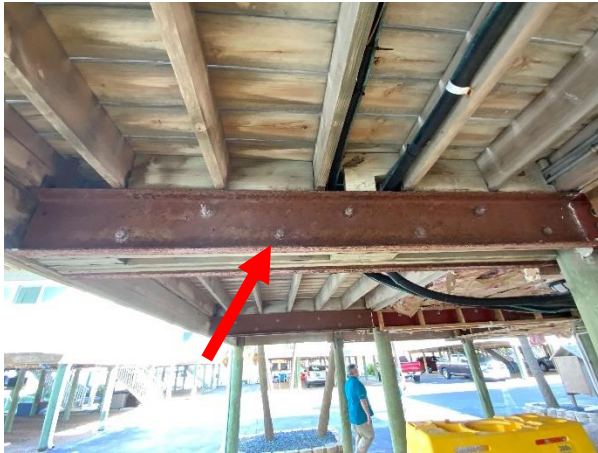
Photo 19 Building 4 – West Elevation – Overall view of corroded exterior steel supports.
