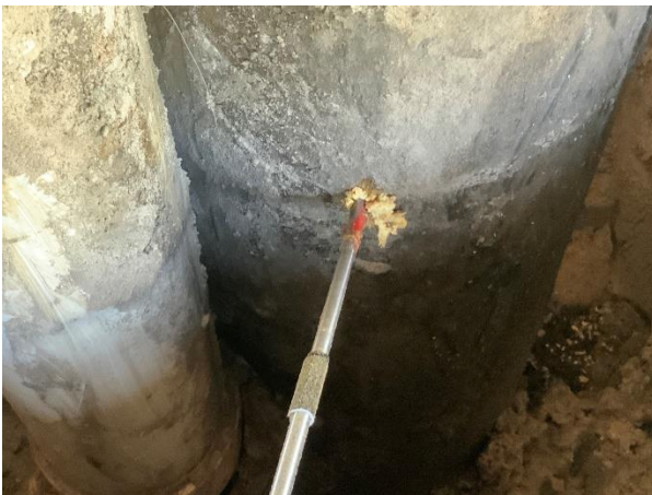
Photo 44 Building 1 – West Elevation – Overall view of core sample of piling base.
