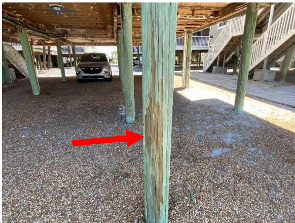
Photo 32 Building 2 – West Elevation – Overall view of splitting piling.
