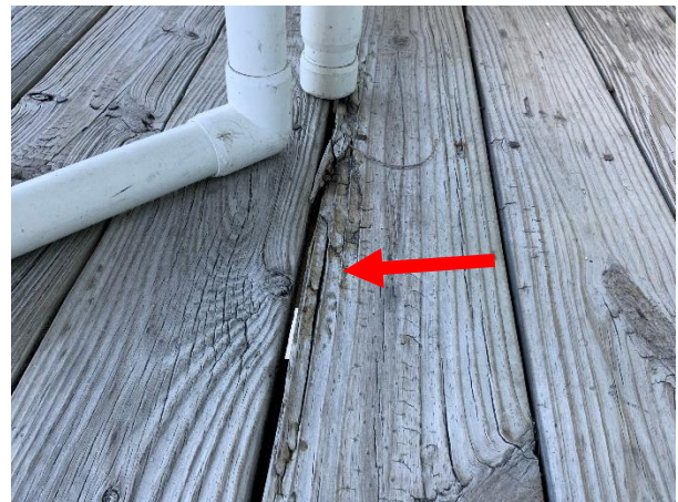
Photo 6 Building 6/7 – West Elevation – Overall view of deteriorated decking.
