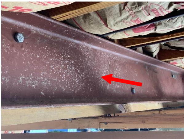
Photo 26 Building 4 – North Elevation – Overall view of corroded interior steel supports.
