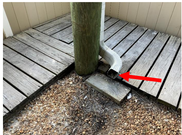
Photo 42 Building 6/7 – South Elevation – Overall view of gutter downspout at piling base.
