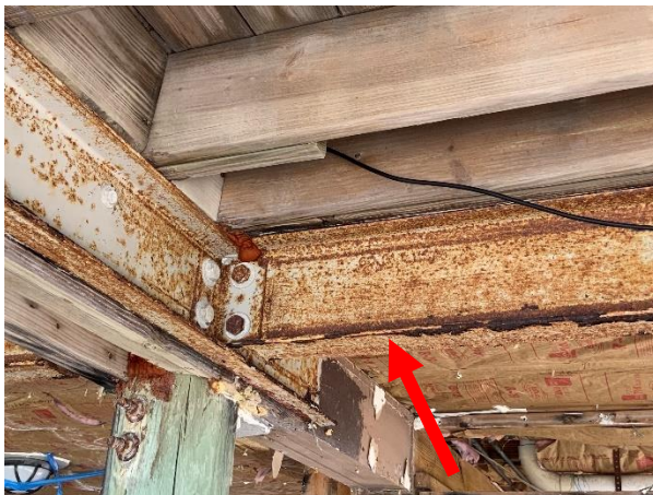
Photo 20 Building 2 – West Elevation – Overall view of corroded exterior steel supports.
