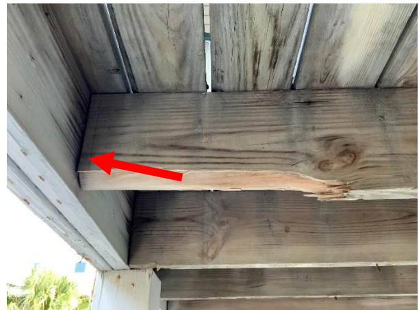
Photo 12 Building 6/7 – West Elevation – Overall view of hangers not installed at joists.
