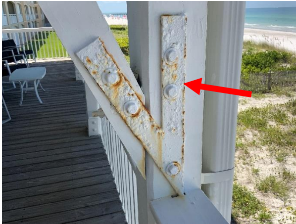
Photo 49 Building 1 – West Elevation – Overall view of corroded metal balcony brackets.
