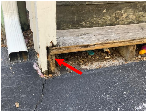
Photo 3 Building 5 – East Elevation – Overall view of deteriorated wood staircase.
