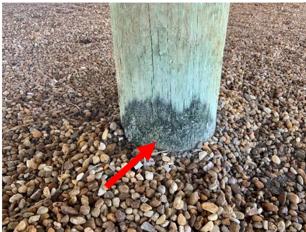
Photo 38 Building 4 – North Elevation – Overall view of staining and microbial growth at piling base.
