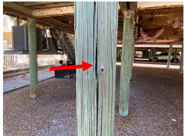
Photo 36 Building 3 – West Elevation – Overall view of splitting piling.
