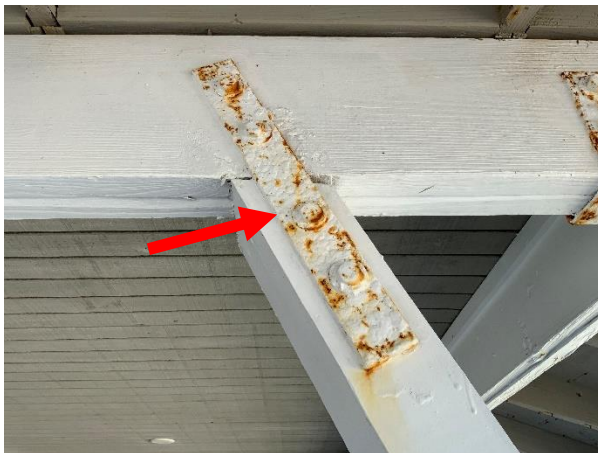
Photo 51 Building 1 – West Elevation – Overall view of corroded metal balcony brackets.
