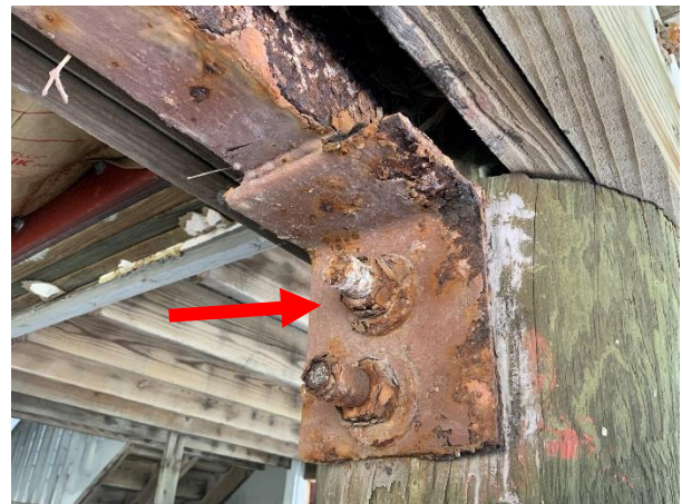
Photo 18 Building 8/9 – West Elevation – Overall view of corroded L brackets.
