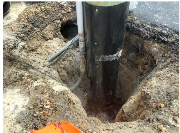
Photo 48 Building 1 – East Elevation – Overall view of Vinyl wrap installation at piling.
