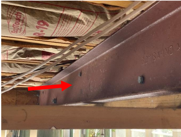
Photo 25 Building 4 – South Elevation – Overall view of corroded interior steel supports.
