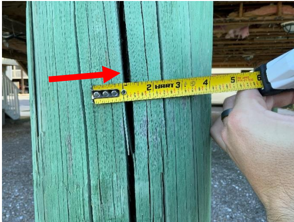
Photo 31 Building 1 – West Elevation – Overall view of splitting piling.
