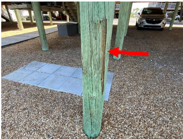
Photo 33 Building 2 – West Elevation – Overall view of splitting piling.
