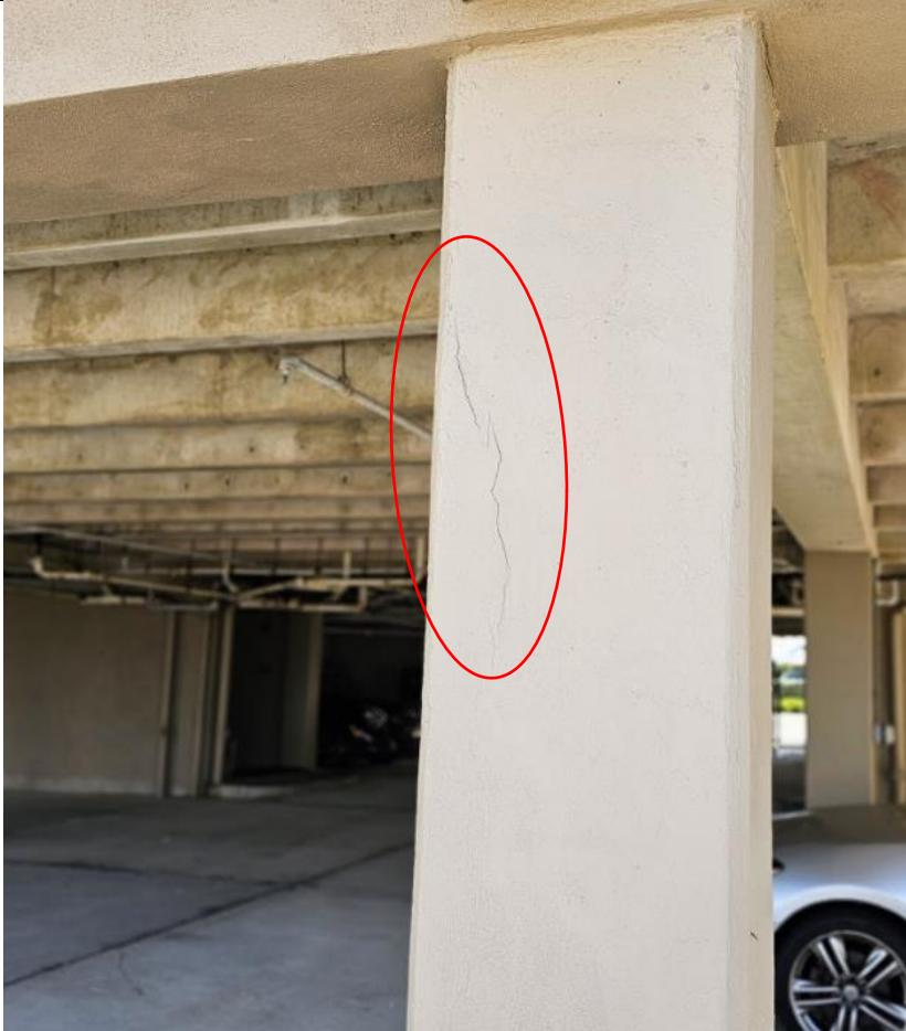
8. Observed cracking on concrete columns in garage.
