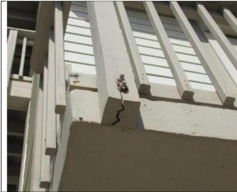
20. Observed wood cracking on guardrails.
