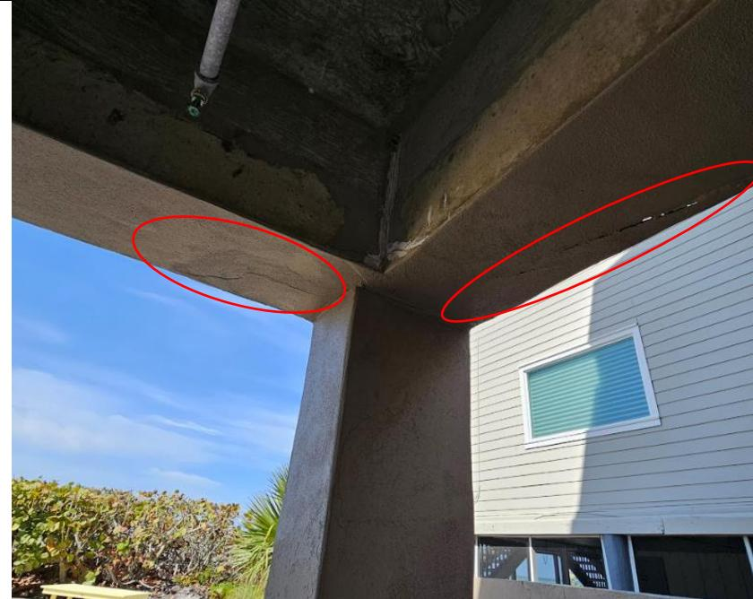
11. Observed cracking on concrete support beams in garage.
