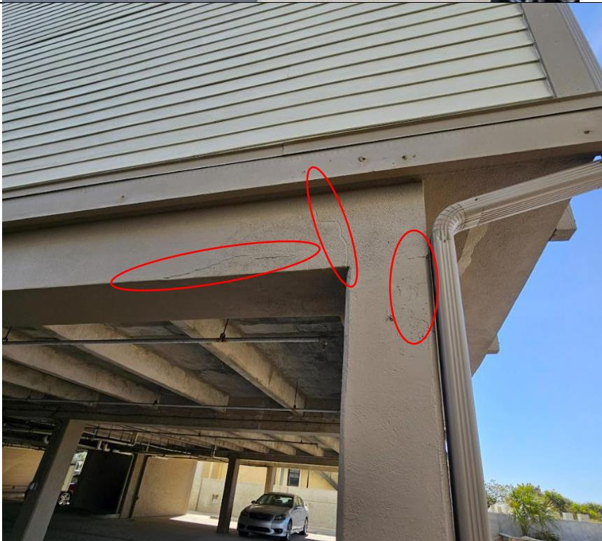
9. Observed cracking on concrete columns in garage.
