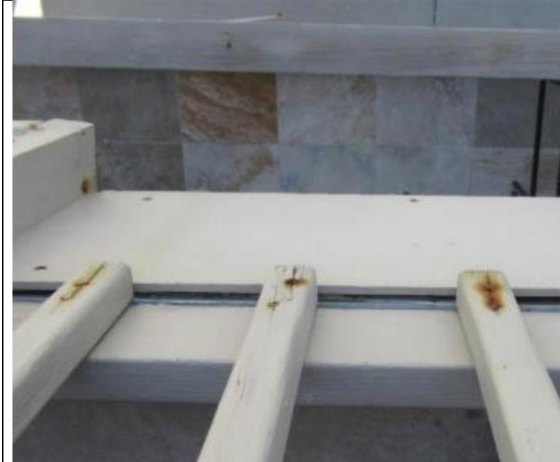
21. Observed rusted fasters on balcony guardrails.
