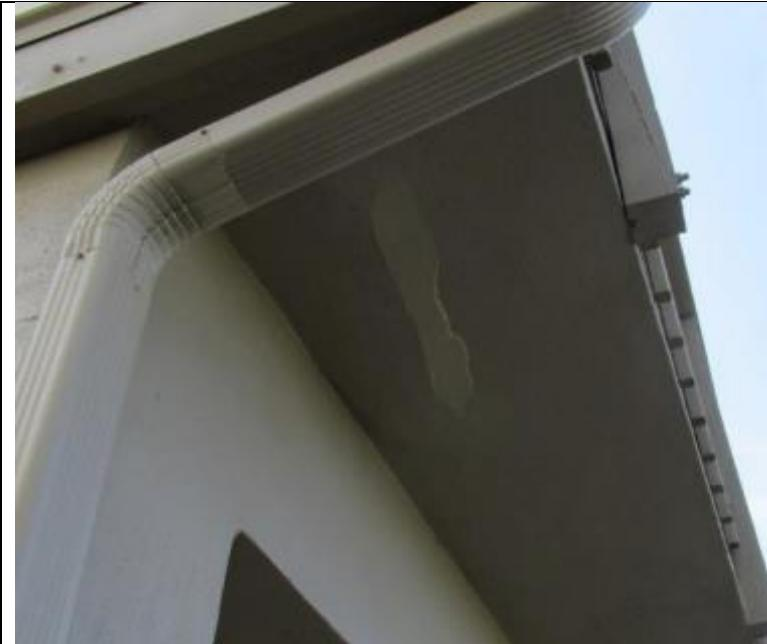
14. Observed loose stucco area on the NW corner of the parking garage (during initial inspection, PRE Hurricane Milton)
