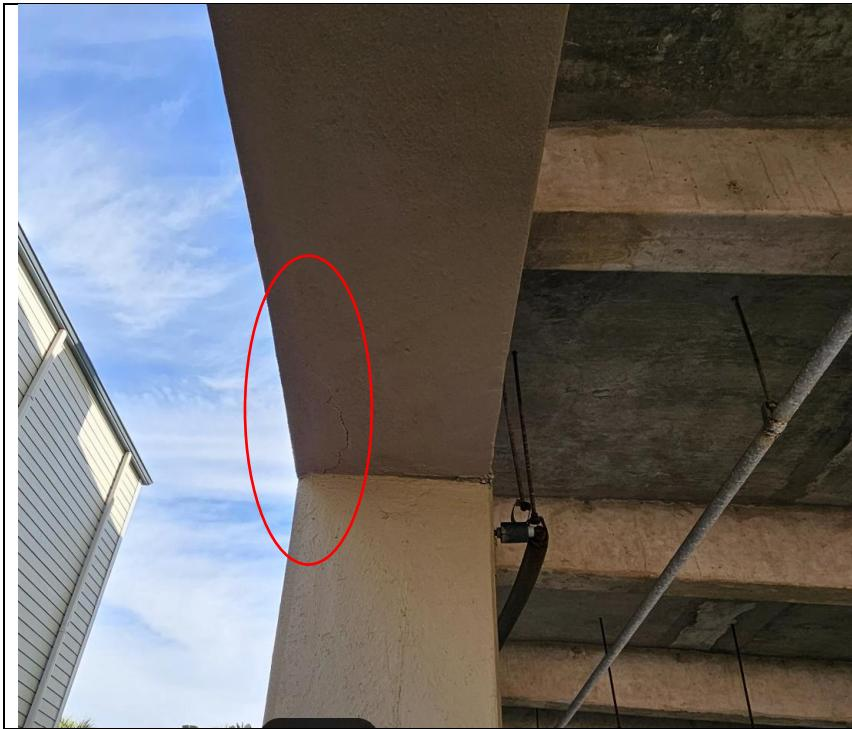
12. Observed cracking on concrete support beams in garage.
