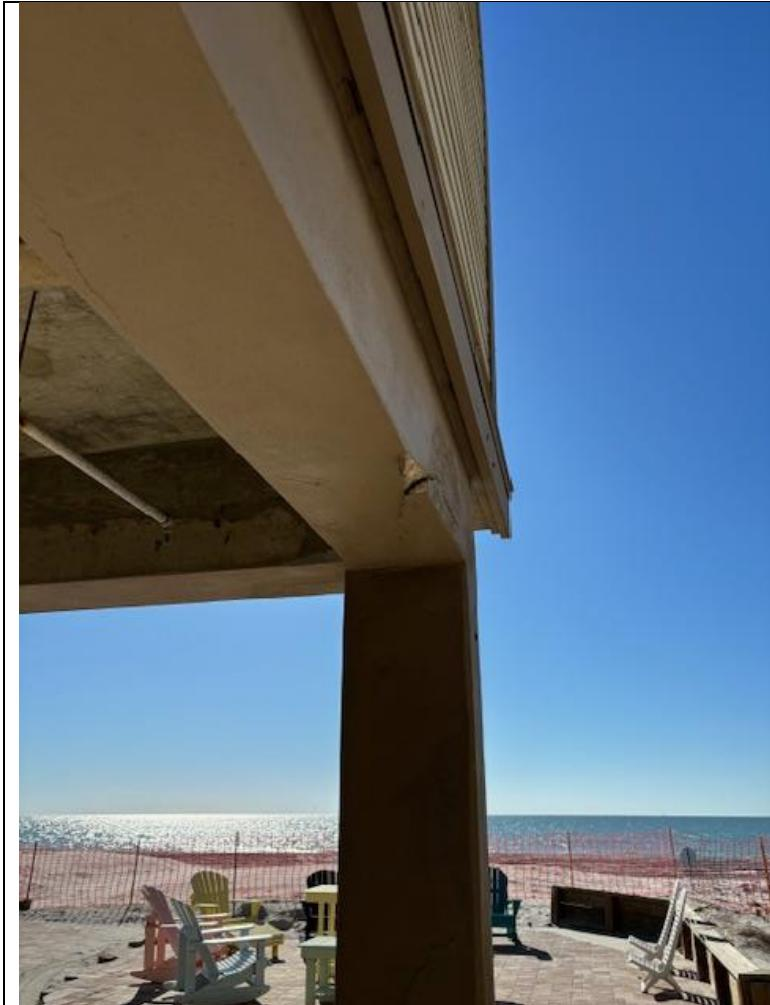
16. Damage observed to concrete column (post hurricane Milton)
