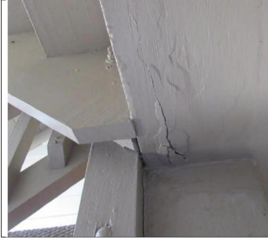
13. Observed spalling and cracking on the south center stairwell in the parking garage.
