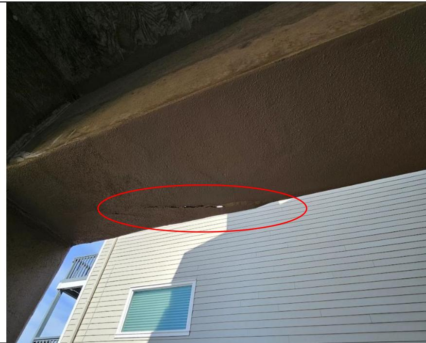
10. Observed cracking on concrete support beams in garage.
