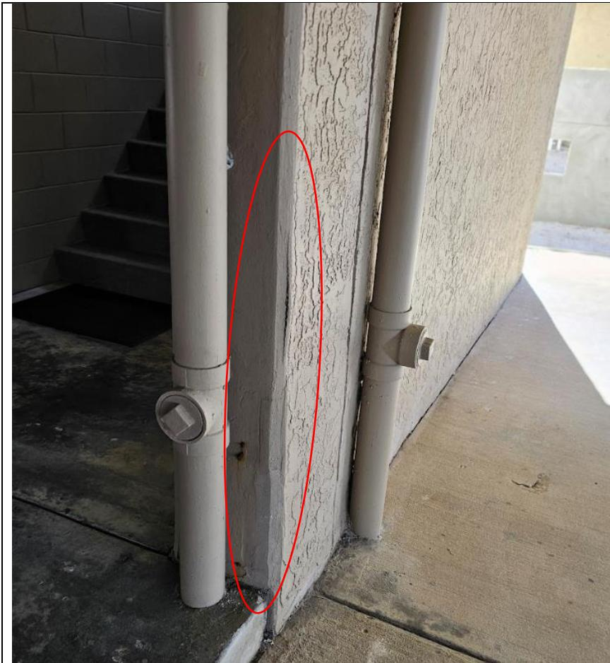
7. Observed efflorescence, separation, and cracking on stucco in garage.
