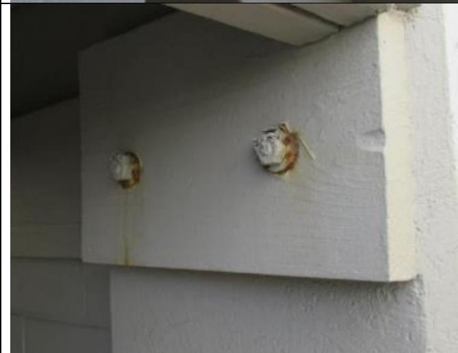
15. Observed rusted anchor support bolts on south center stairwell in the parking garage (Pre-Hurricane Milton)
