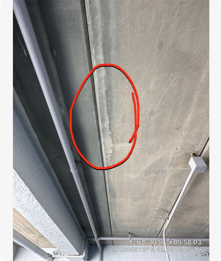
Minor ceiling slab spalling adjacent to elevator in garage. Repair is recommended, although this does not qualify as substantial structural deterioration.
