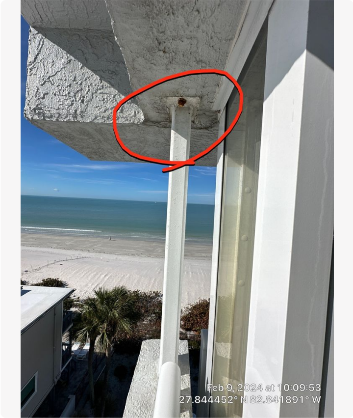
Unit 501. Early-onset corrosion on nut and bolt for balcony support post. This condition is typical throughout the building. As a preventative maintenance item, these fasteners should be cleaned and coated or replaced.
