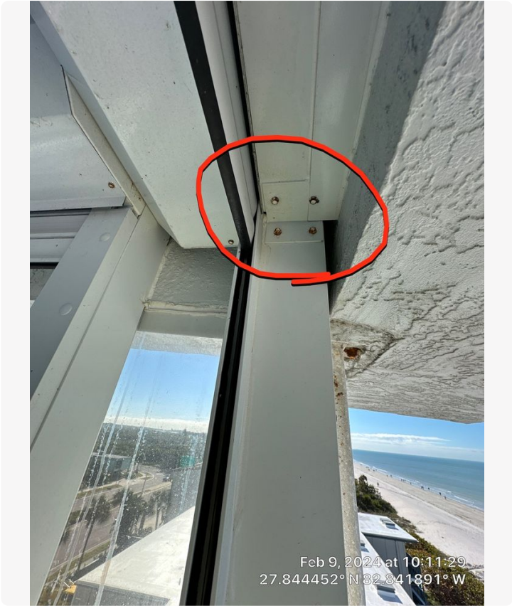
Unit 501. Corrosion of fasteners for storm shutter bracket. This corrosion is fairly minor and typical for the building, although the fasteners should be periodically observed to make sure that they remain in serviceable condition.
