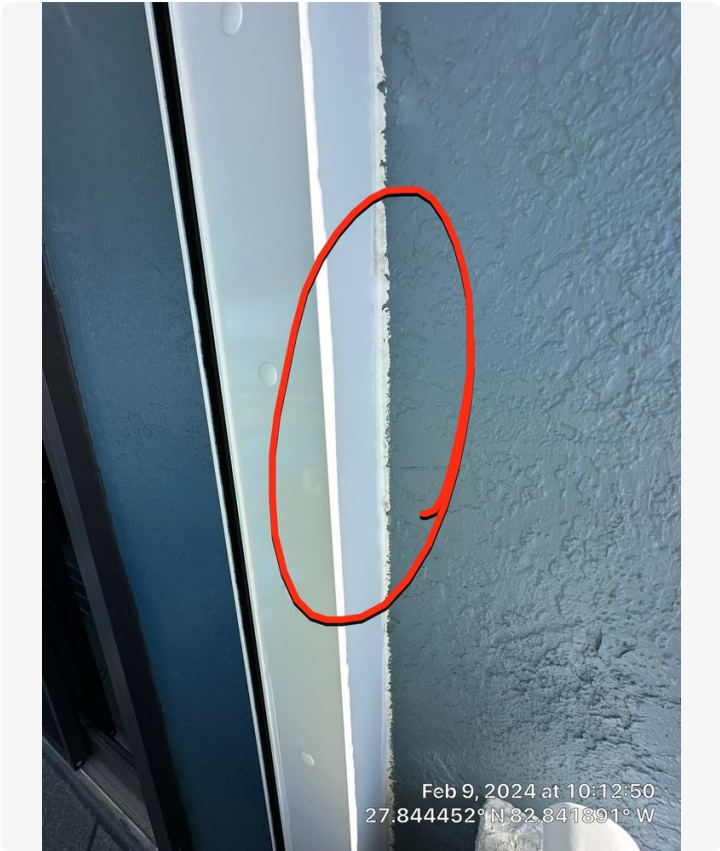
Unit 501. Sealant at storm shutter perimeter is in good condition and pliable.
