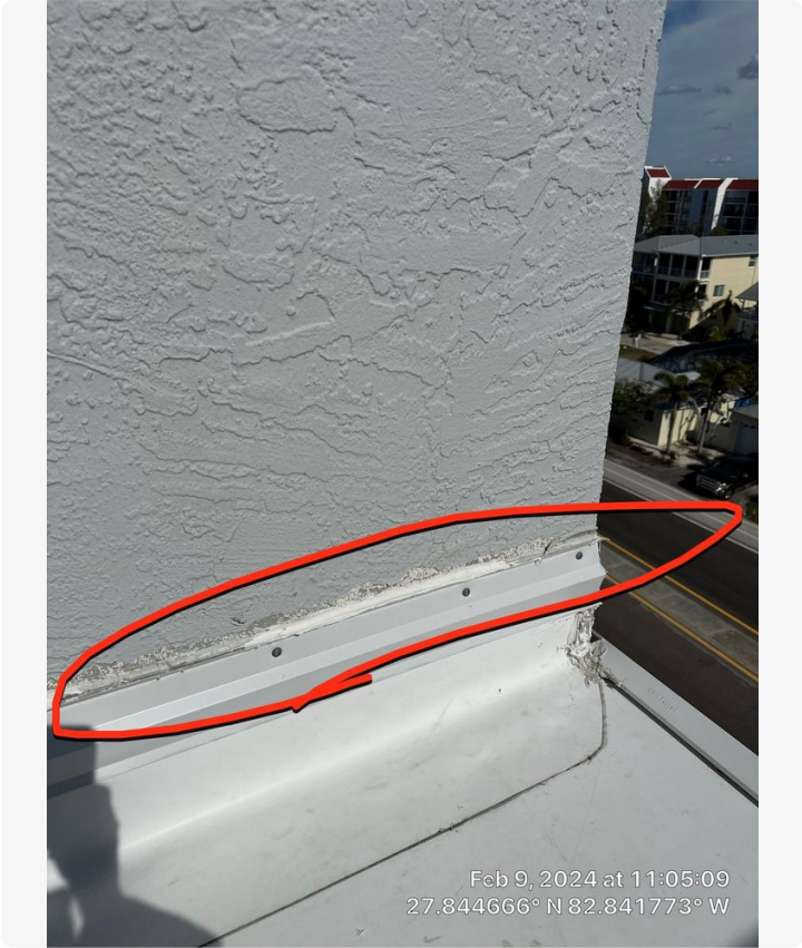
Bare stucco and missing sealant observed at roof counter flashing in several locations on flat roof. Recommend caulking replacement and repainting.
