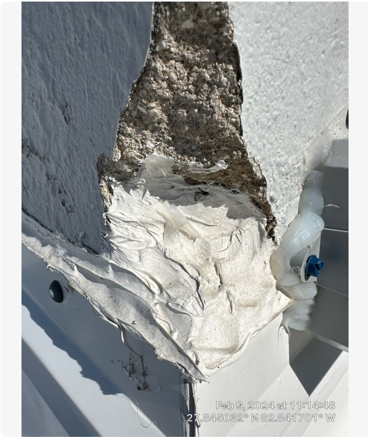
Southeast corner of Roof, block wall appears to have been repaired attempted by filling up with caulk.
