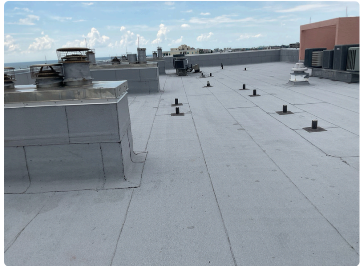
Modified bitumen roof overview
