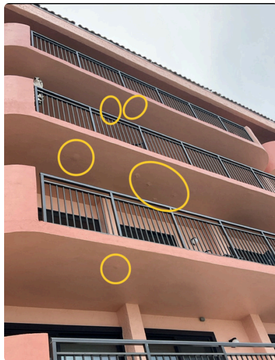
Paint bubbling on Units 403, 503, and 603 balcony soffits
