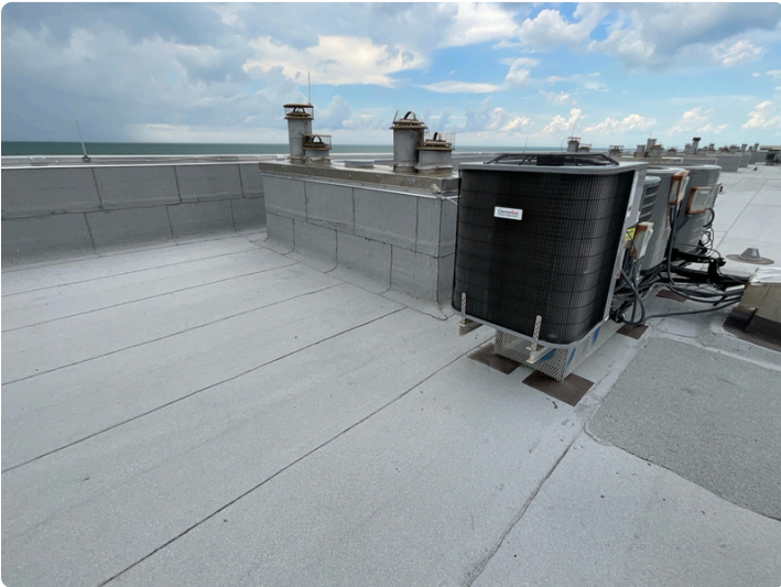
Modified bitumen roof overview
