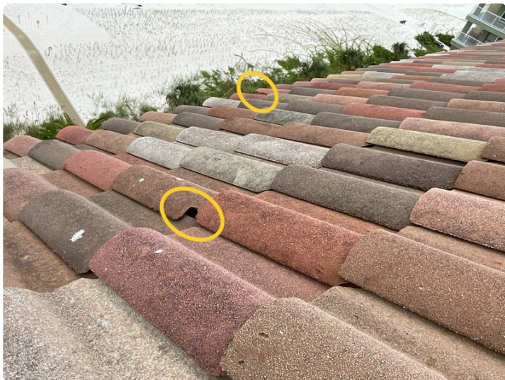
Chipped tiles on rear elevation mansard roof
