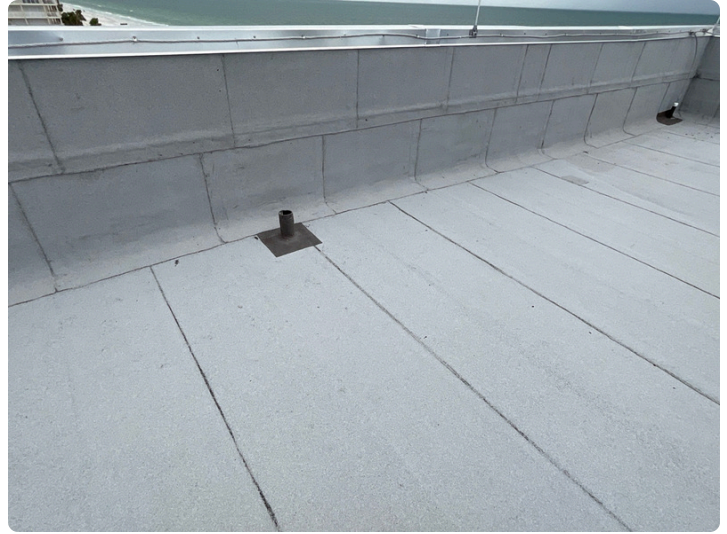
Modified bitumen roof overview
