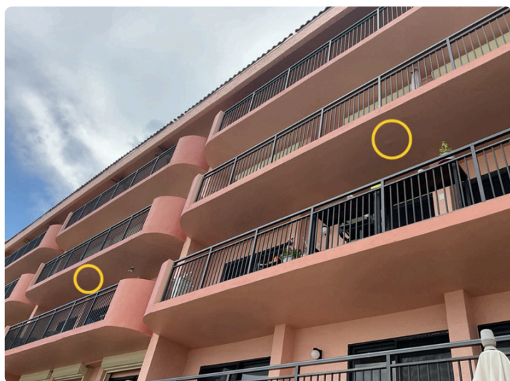
Paint bubbling on Units 504 and 505 balcony soffits
