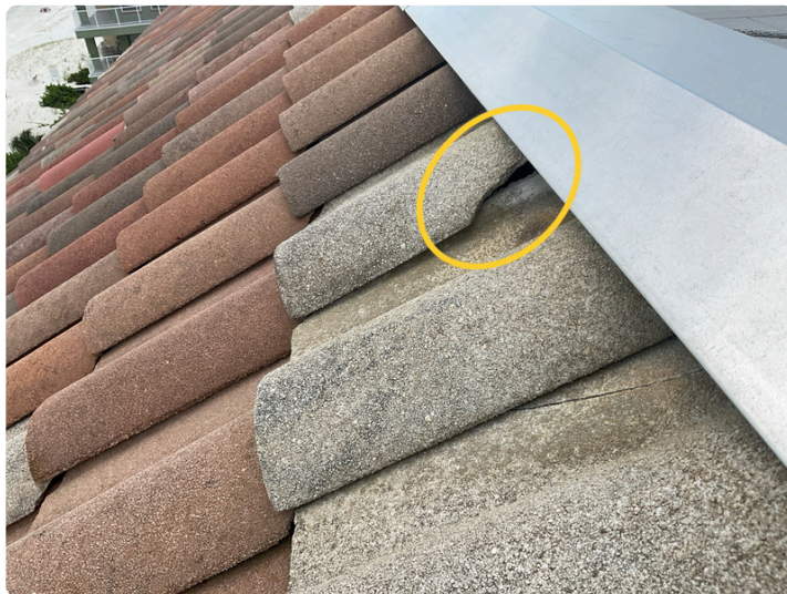
Chipped tile on rear elevation mansard roof
