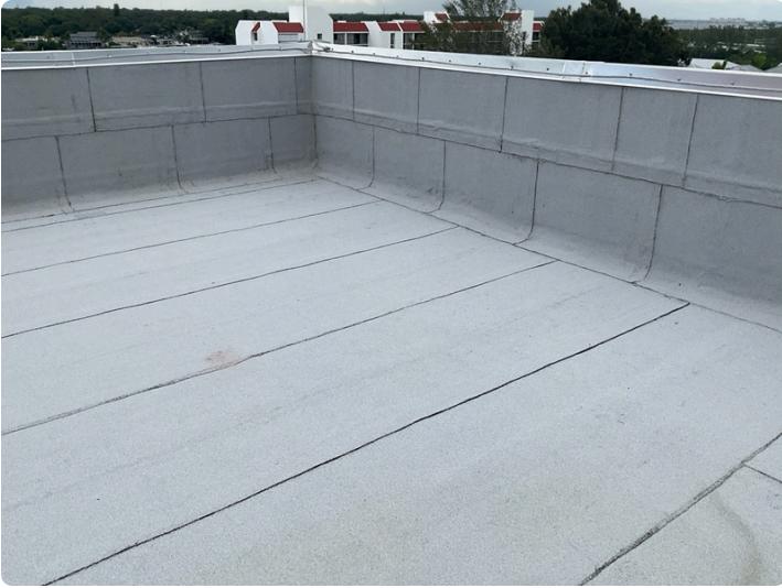
Modified bitumen roof overview
