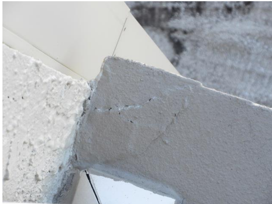
Concrete Spalls at Corner of Railing Post on 4 th Floor Walkway.
