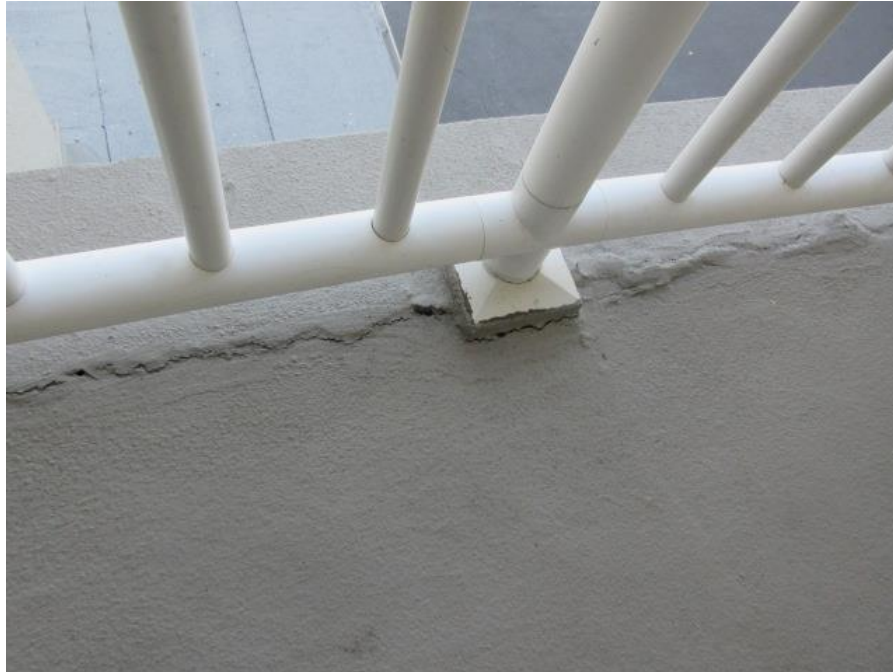
Failed Bond Line at Previous Slab Edge Repair on 4 th Floor Walkway.
