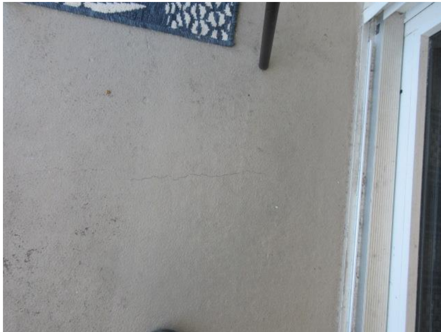
Typical Deck Crack in Front of SGD's Balconies.
