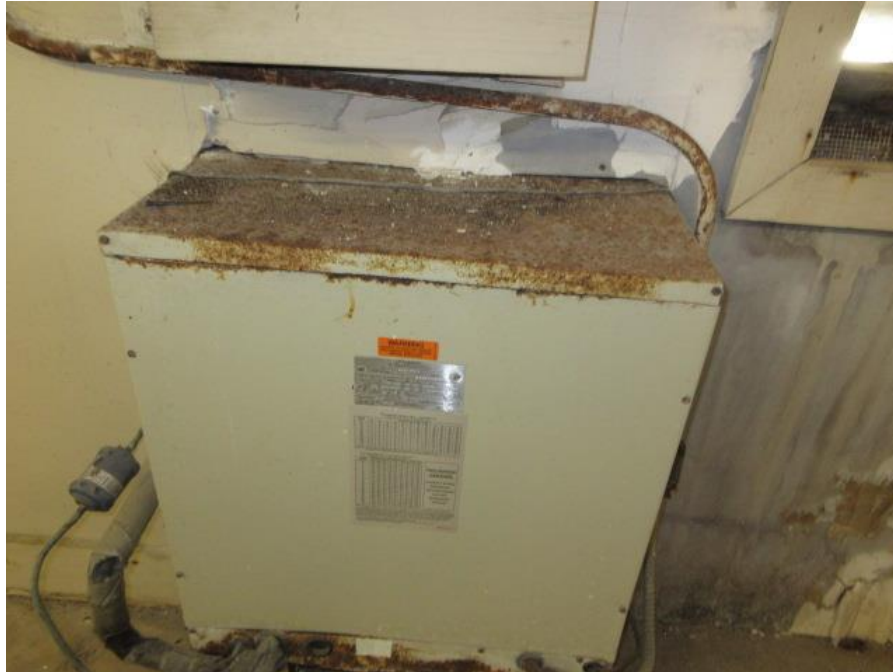
Heavily Rusted Electrical Components (TYP).
