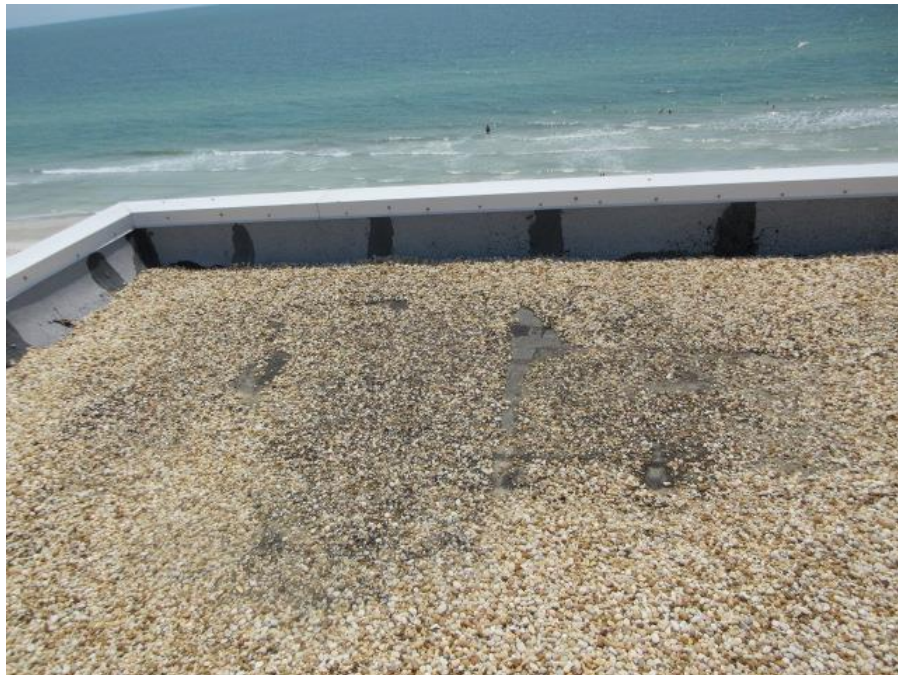
Sign of Water Ponding on Roof Materials.
