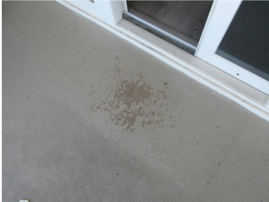
Failed Acrylic Coating over Brown Floor Paint on Balconies (TYP).
