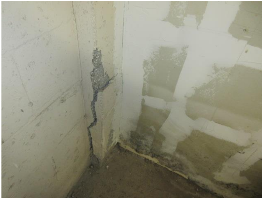
Concrete Spalls at the Top and Bottom of Corner Columns in Electrical Room.
