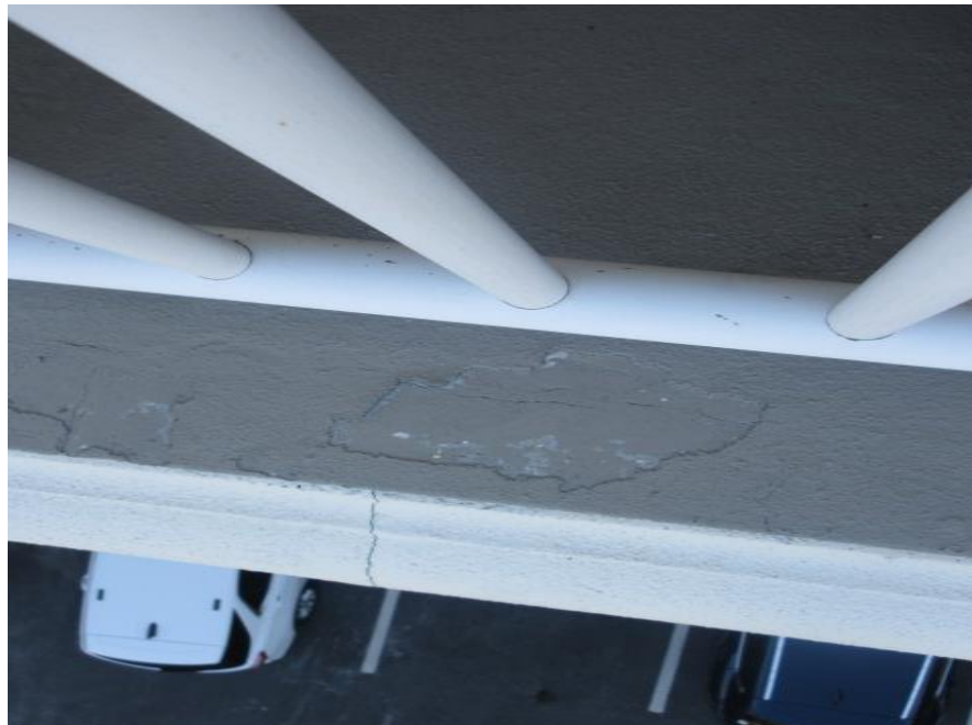
Concrete Delamination and Crack at Slab Edge on Common Walkways(TYP).
