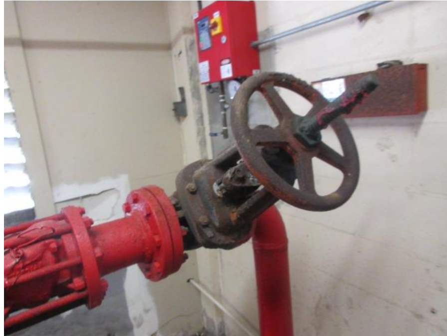
Water Valves with Surface Rust at Fire Pump Room.
