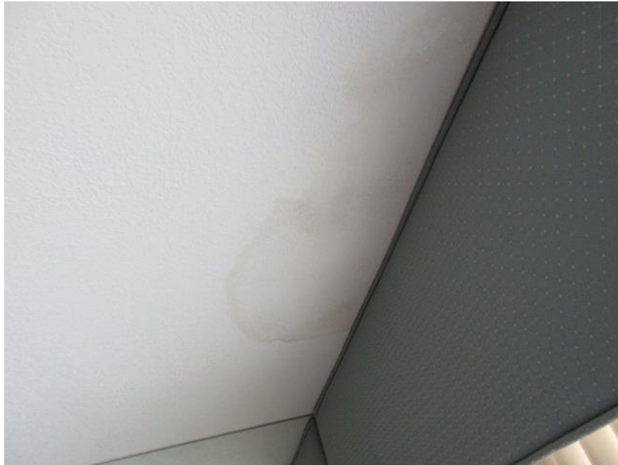
Water Stain on Ceiling at SGD South End in Unit #403.
