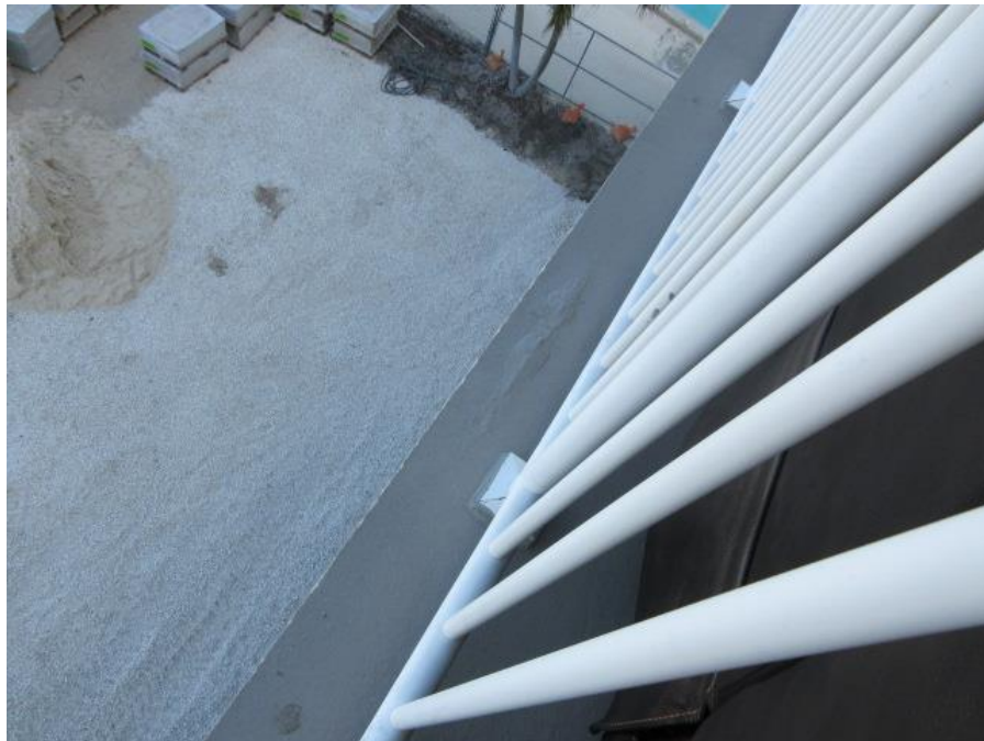
Small Concrete Spalls at Slab Edge on Walkways (TYP).
