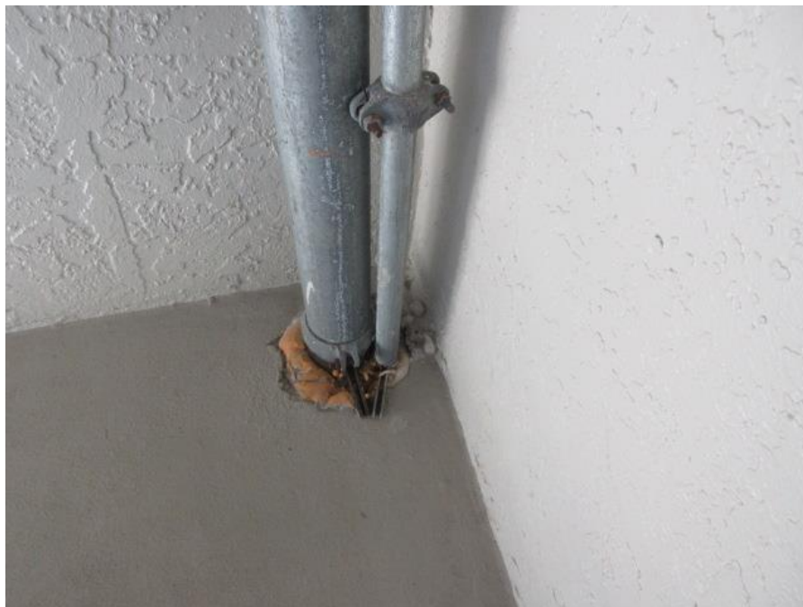
Stand Pipes Holes Filled with Spray Foam on Emergency Stairwells (TYP).
