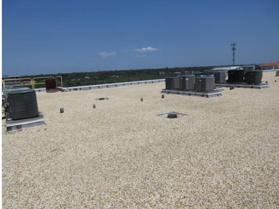
Overview of of Tar and Gravel Roof System.
