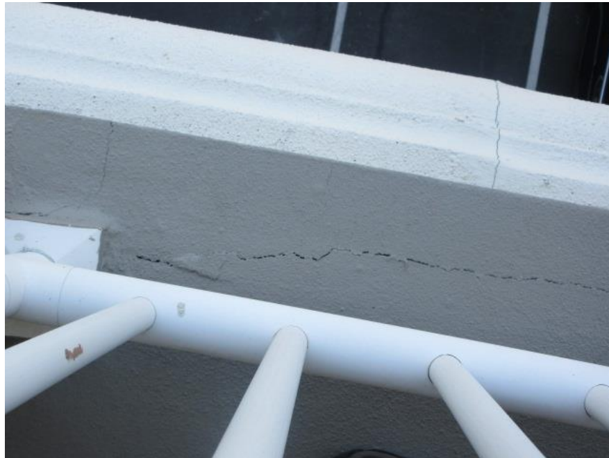
Typical Concrete Cracks Along Slab Edge on Walkways.
