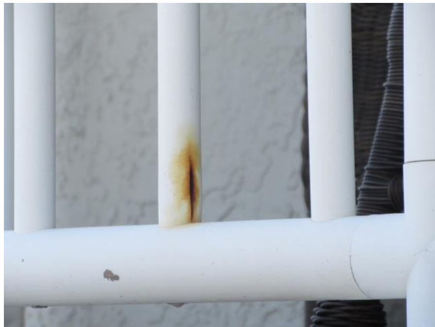
Typical Splitting of PVC Railing Due to Rusted Steel Posts wWthin
