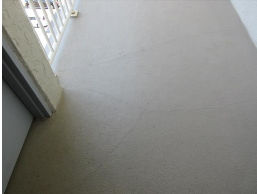
Failed Previous Deck Crack Repairs on Common Walkways (TYP).
