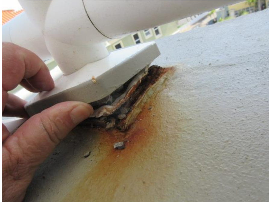
Typical Heavily Rusted Base Plate at Balcony Guardrail
