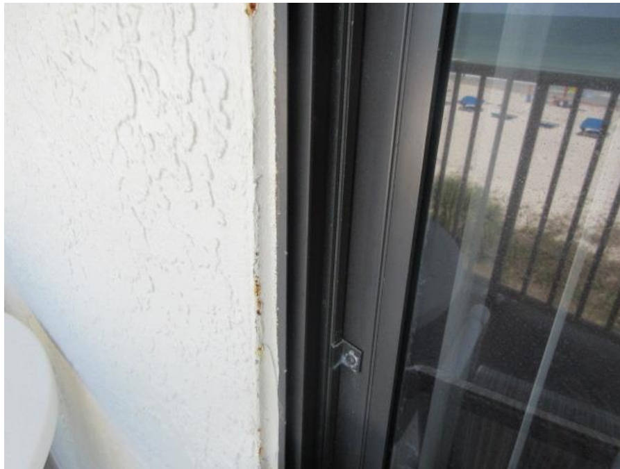
Rusted Corner Bead Stucco at SGD at Unit #201.
