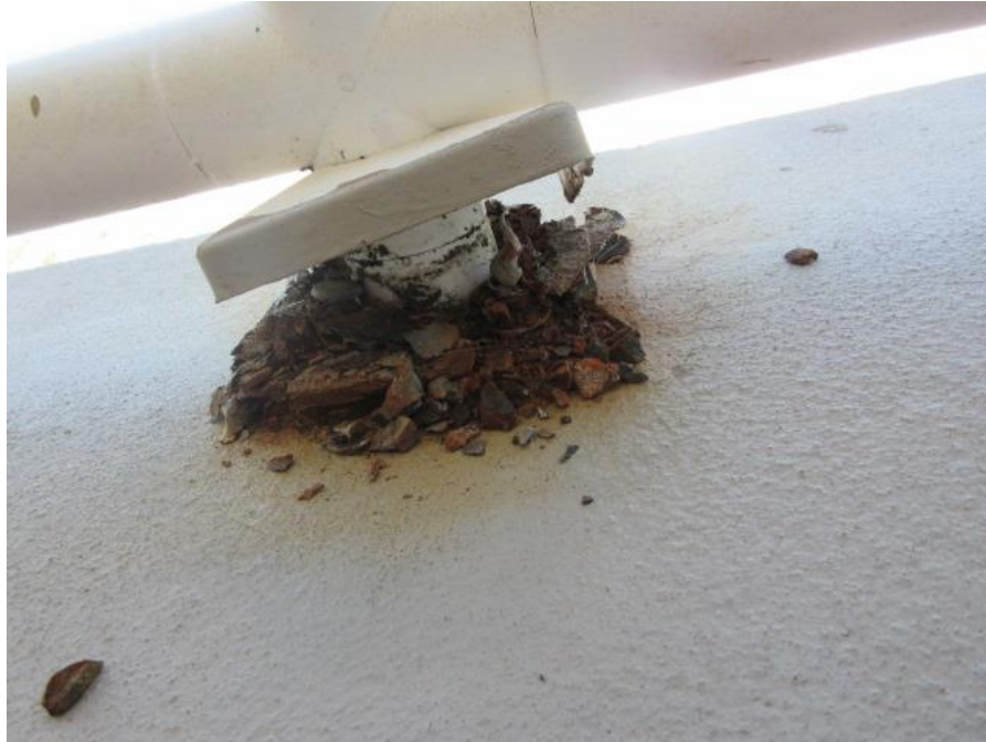
Desintegrated Base Plate due to Rust at Unit #201.
