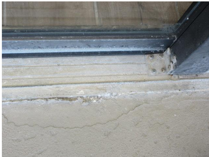
Sliding Glass Door Installed Lower Than Balcony Deck in Unit #406 with Missing/Failed Track Perimeter Sealant and Peeled Floor Coating
