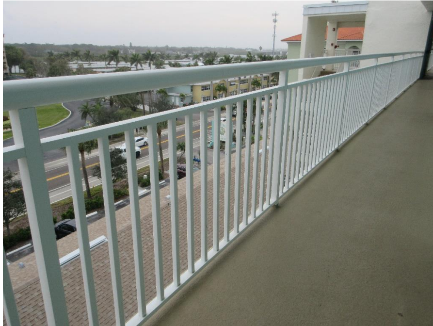
Photo #25 – Typical Balcony Railing at Elevated Walkways (42 ¼" Height, 3 ½" Picket Spacing, 1 ¾" Bottom Rail Height).
