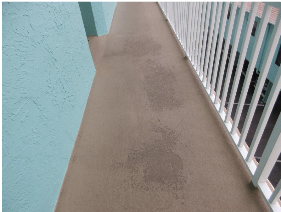
Photo #22 – Typical Concrete Slab Surface Damages or Spalls Covered with Floor Paint (TYP.)
