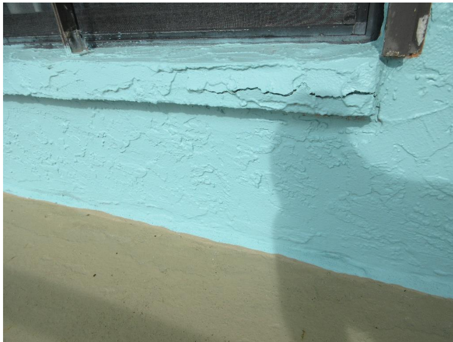
Photo #18 – Broken Windowsill at Unit #501.
