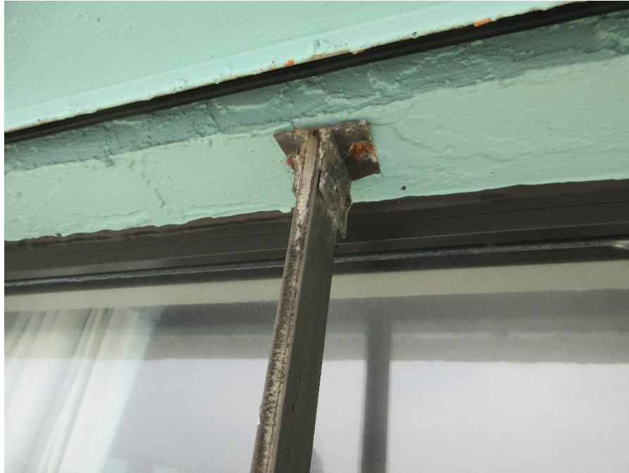
Photo #17 –Corroded Shutters Framing (TYP.)
