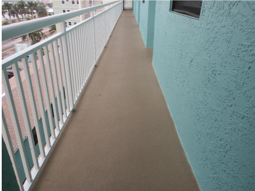
Photo #21 – Overview of Walkways Deck Coating
