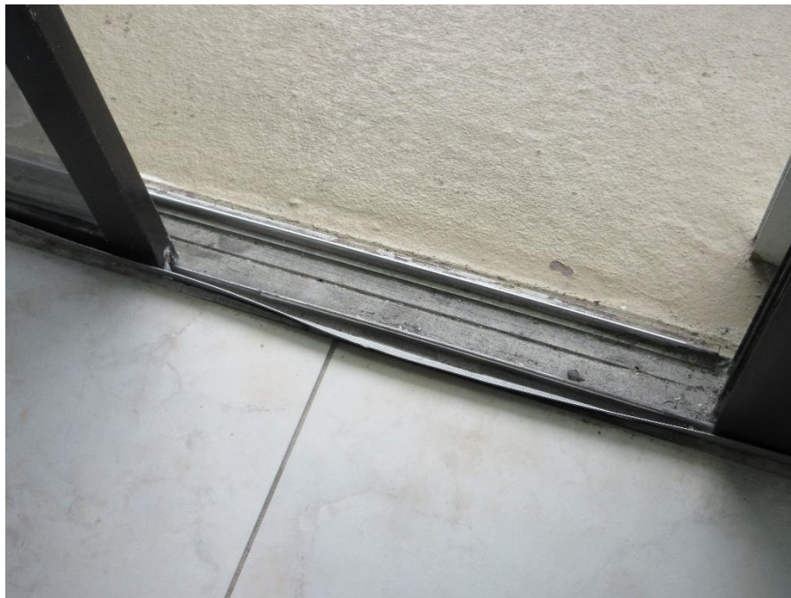
Photo #10 – Damaged and Low Door Threshold (TYP.).
