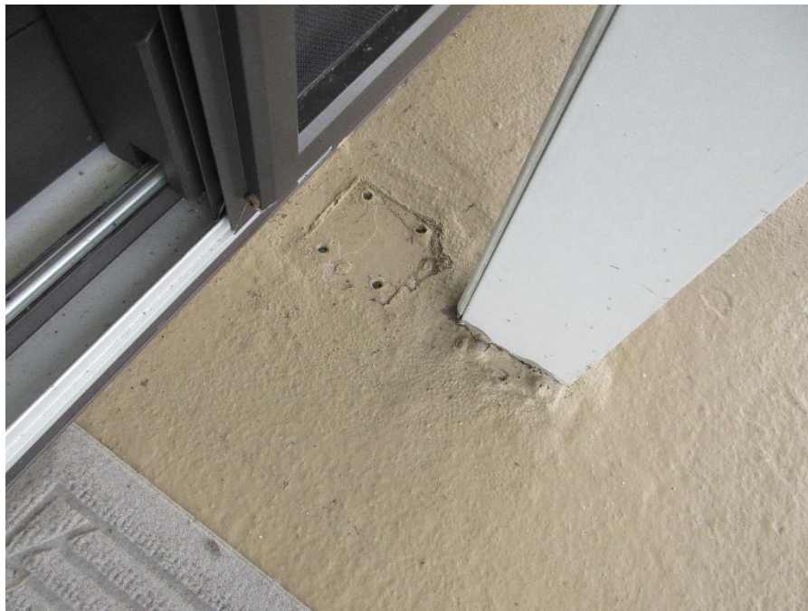
Photo #16 –Unfilled Holes Left in Balcony Deck.
