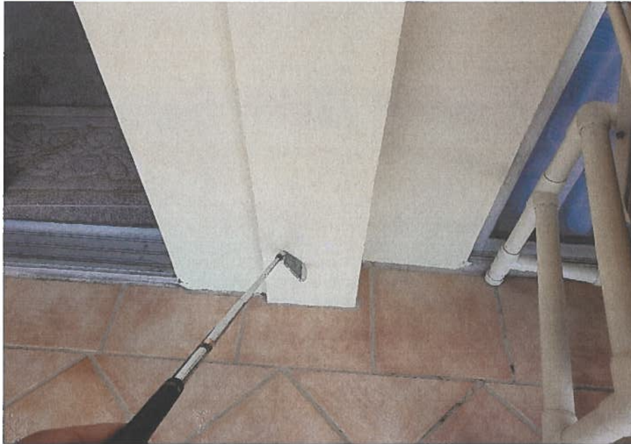
Figure A- 11: Typical delaminated area at the bottom of concrete column.
