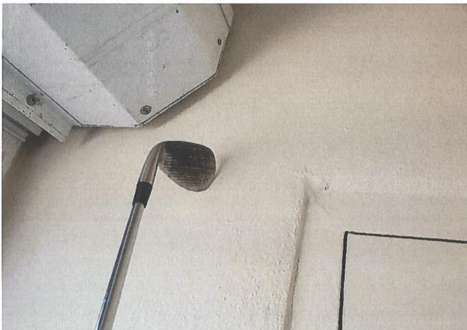
Figure A- 12: Typical delaminated area on side of exterior storage wall.
