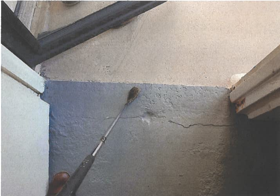
Figure A- 36: Typical hairline cracking on slab surface at the entrance of the stairs.
