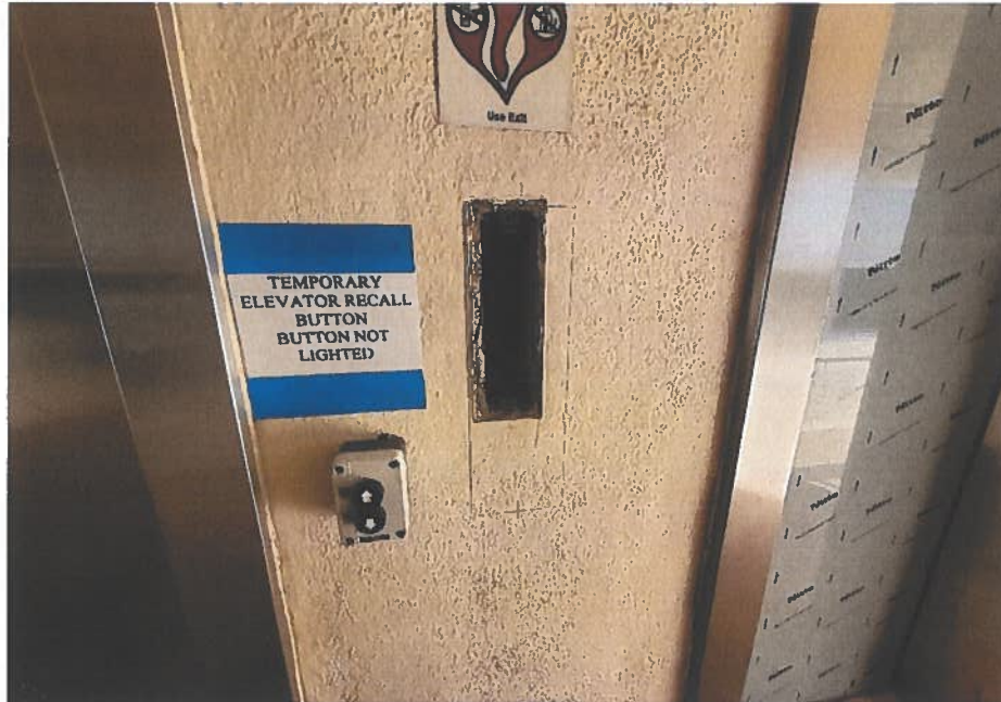
Figure A- 37: Observation of opening at the corridor wall due to elevator maintenance work.
