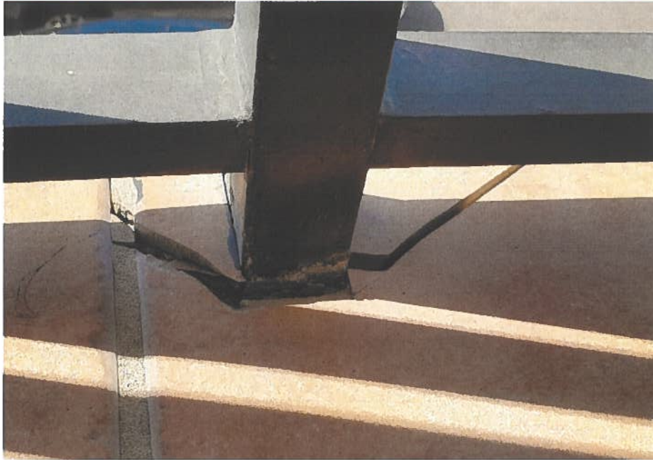
Figure A- 23: Typical spalling area on top of balcony slab surface with Cracked tiles around guardrail post
