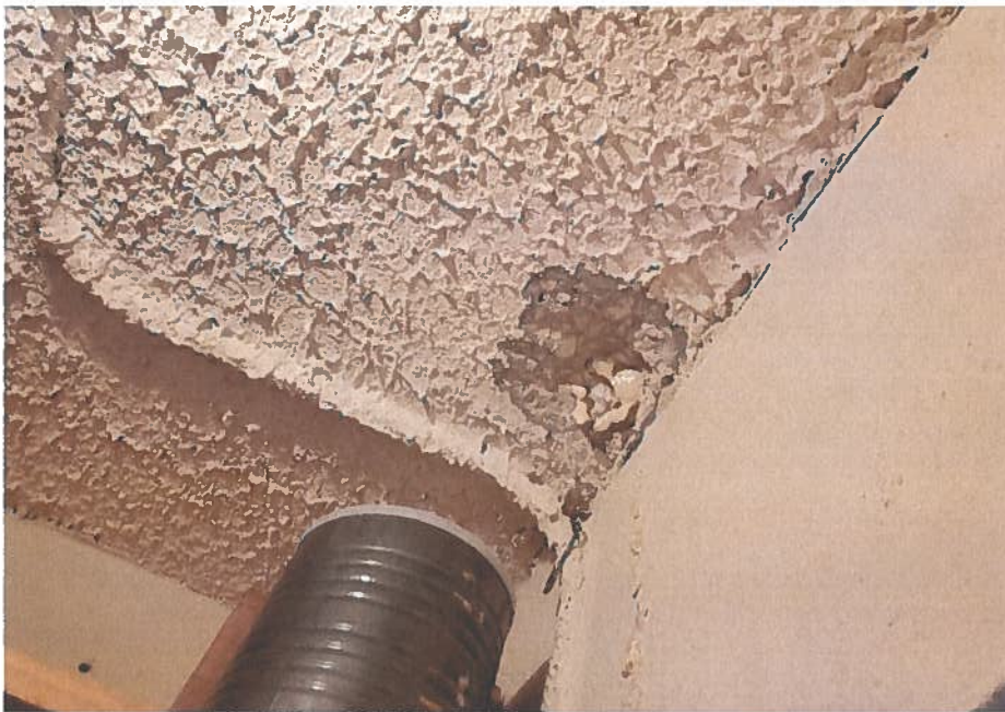
Figure A- 26: Typical concrete spall on storage ceiling.
