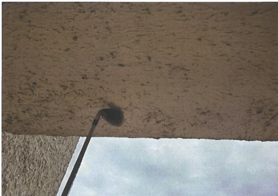
Figure A- 38: Delaminated area at corridor ceiling slab.
