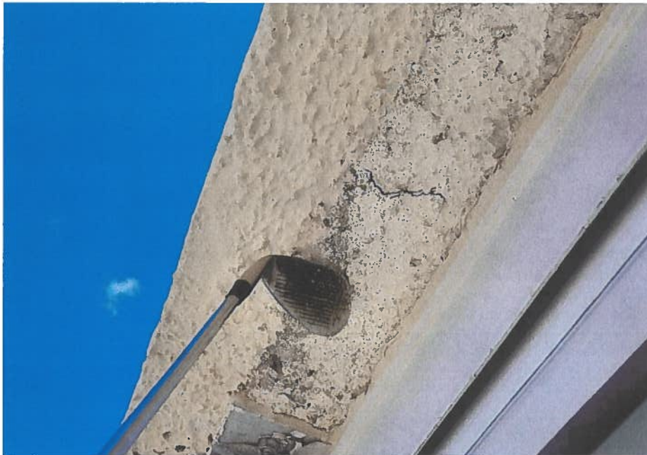
Figure A- 8: Typical spalled area at balcony slab edge.
