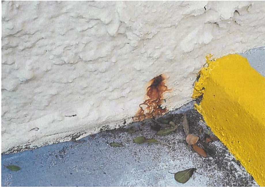
Figure A- 45: View of corroded metal and spalling on the exterior stucco finish.
