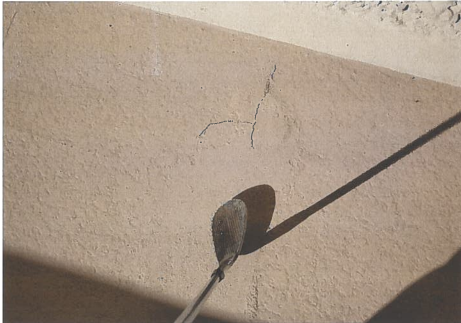
Figure A- 34: Observation of spalling over knee wall scupper
