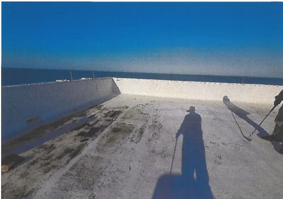
Figure A- 2: Observation of signs of typical roof ponding water.
