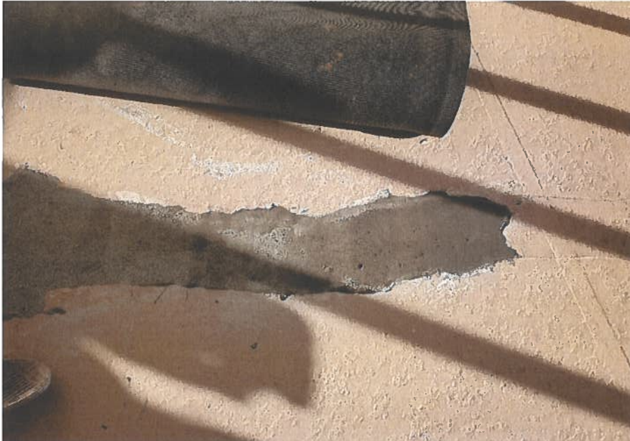
Figure A- 32: Typical hairline cracking over apparent repair on corridor surface.
