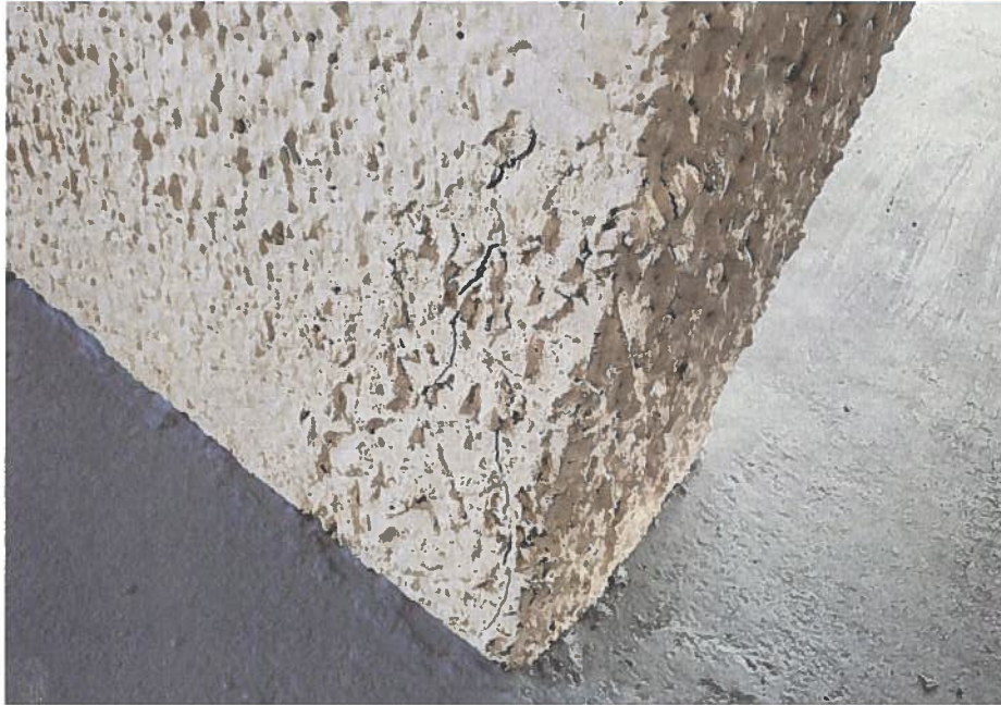
Figure A- 43: Typical cracking at base of wall on parking garage entrance.
