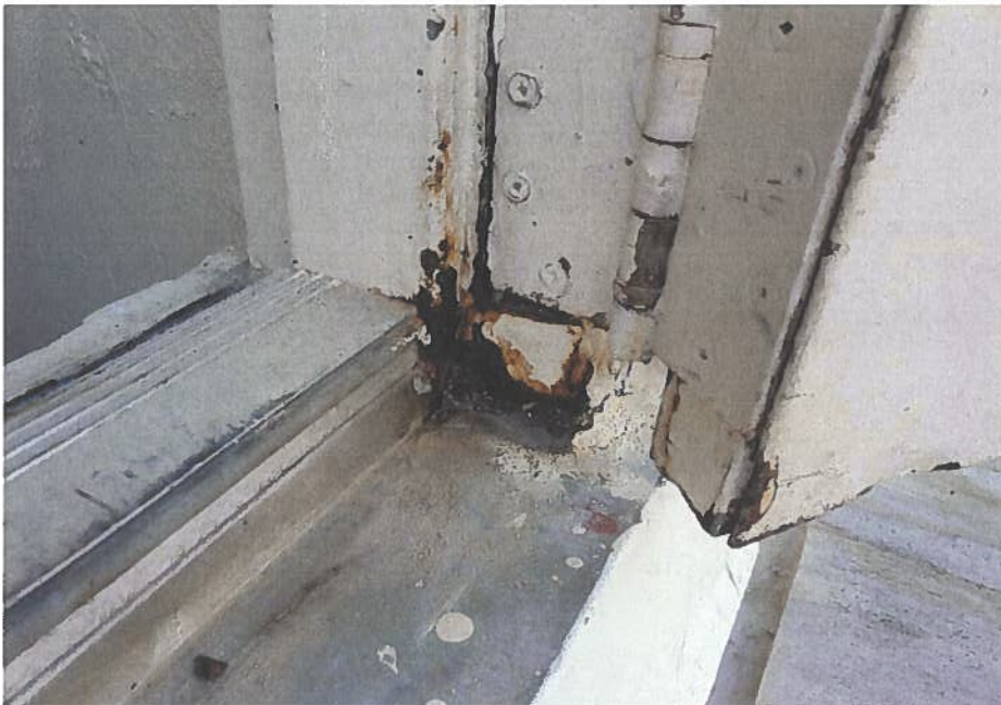
Figure A- 4: Typical rusty metal at the door frame on the roof area.
