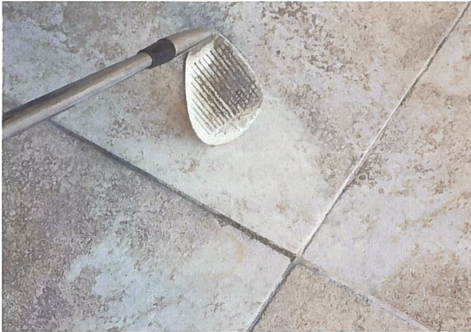
Figure A- 17: Observation of popped up tile on balcony surface.
