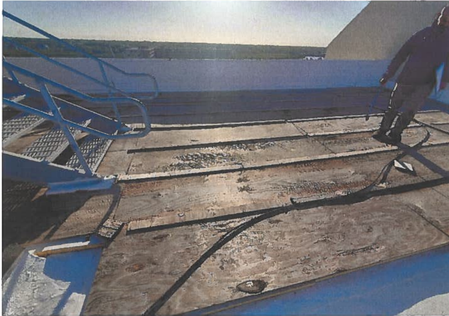
Figure A- 3: Observation of protective cover while carrying out maintenance work on the elevator.
