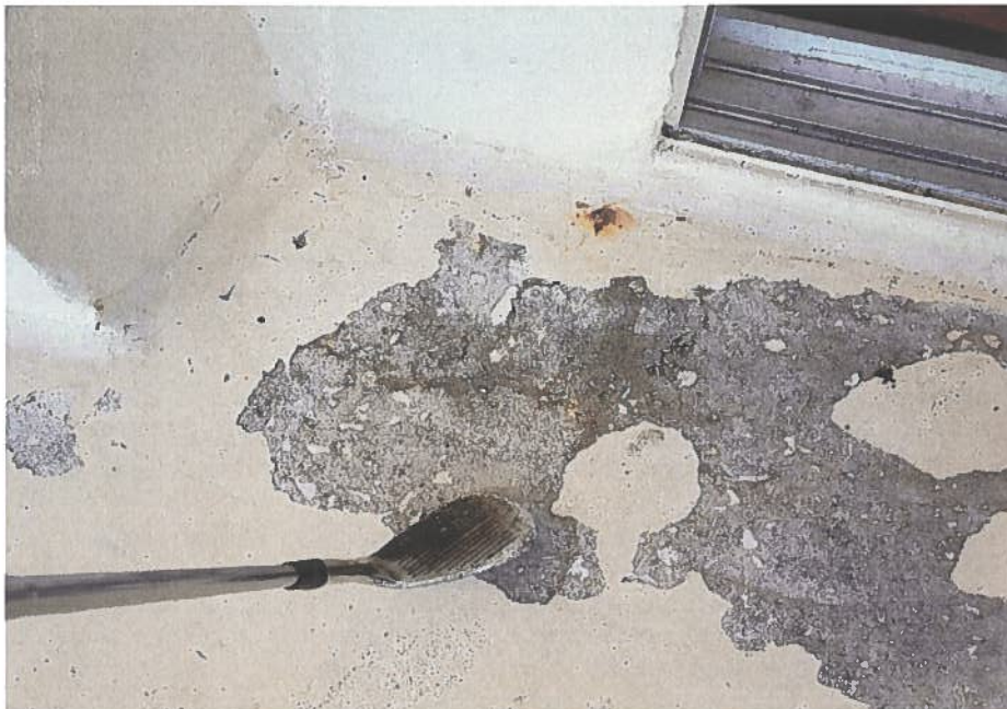
Figure A- 20: Spall on balcony surface with missing waterproofing
