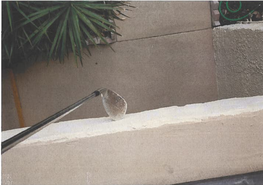
Figure A- 39: Typical delaminated area at corridor slab edge.
