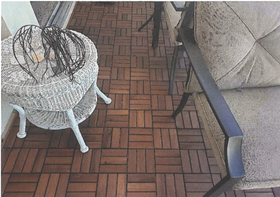
Figure A- 24: Typical view of balcony covering that does not allow for proper inspection.
