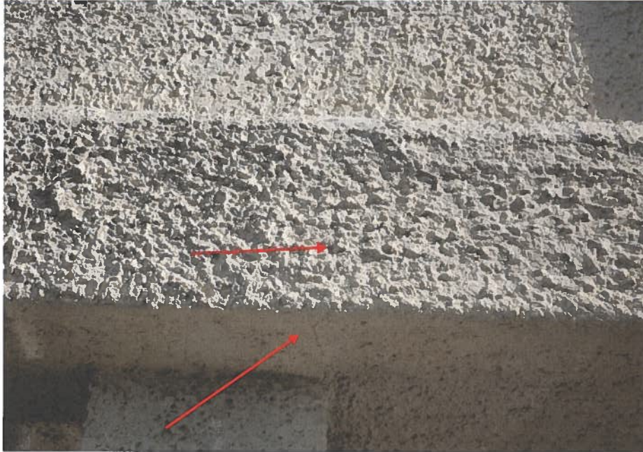
Figure A- 41: Stucco cracking at the left garage entrance ceiling slab.
