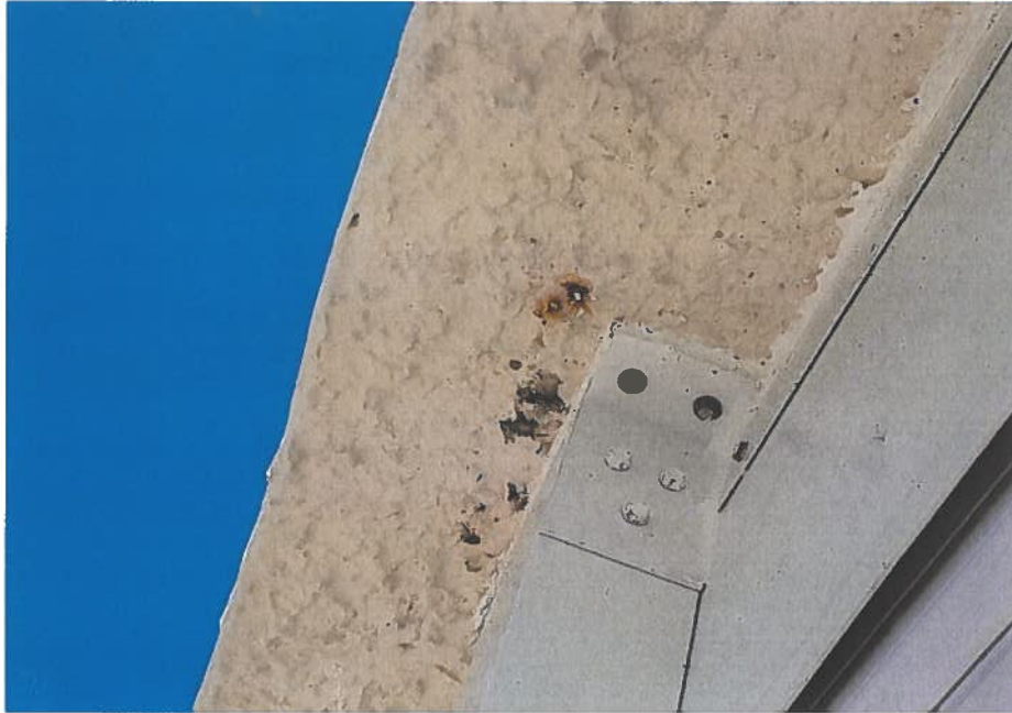
Figure A- 25: View of corroded metal on balcony ceiling.
