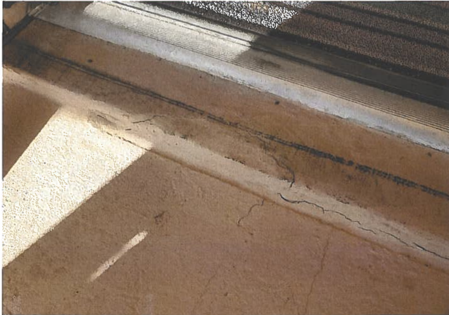
Figure A- 31: Typical hairline cracking with spalling in front of a unit entrance.
