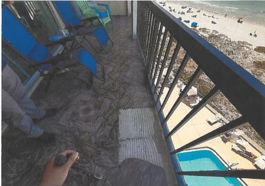
Figure A- 19: Observation of missing tiles on the balcony surface that allows the entry of water beyond the tile.
