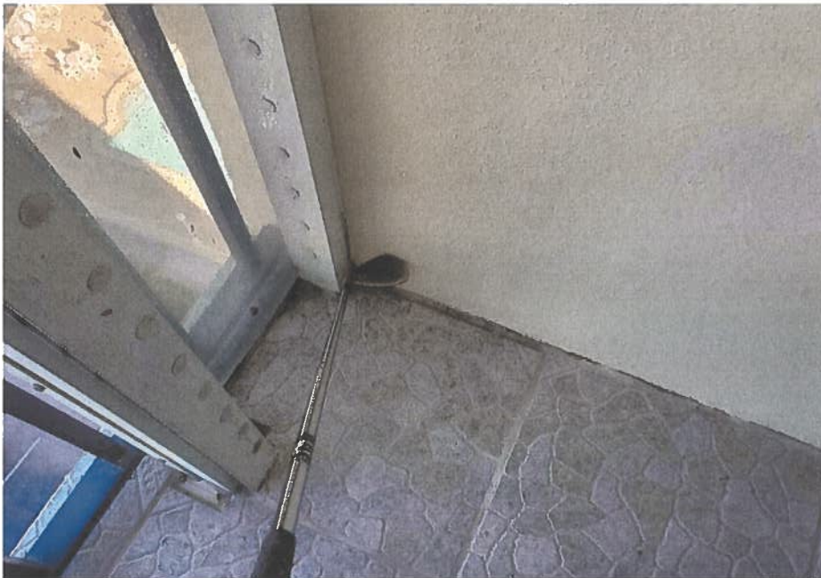
Figure A- 10: Typical delaminated stucco area on side of concrete wall.
