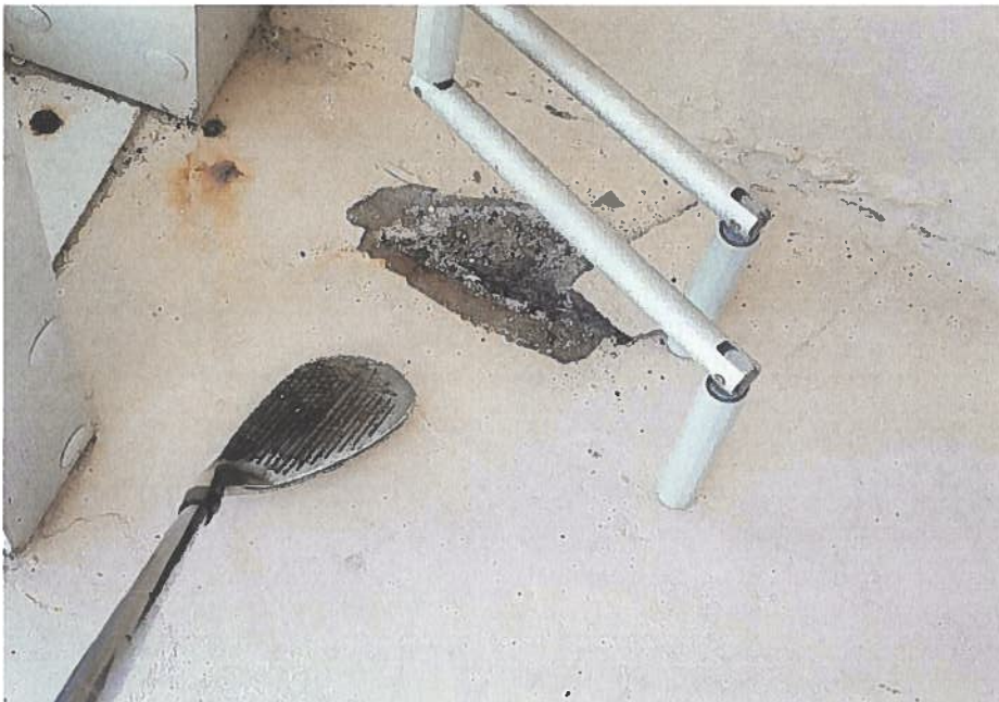
Figure A- 16: View of spall area on balcony surface with corroded rebar and penetration through waterproofing.
