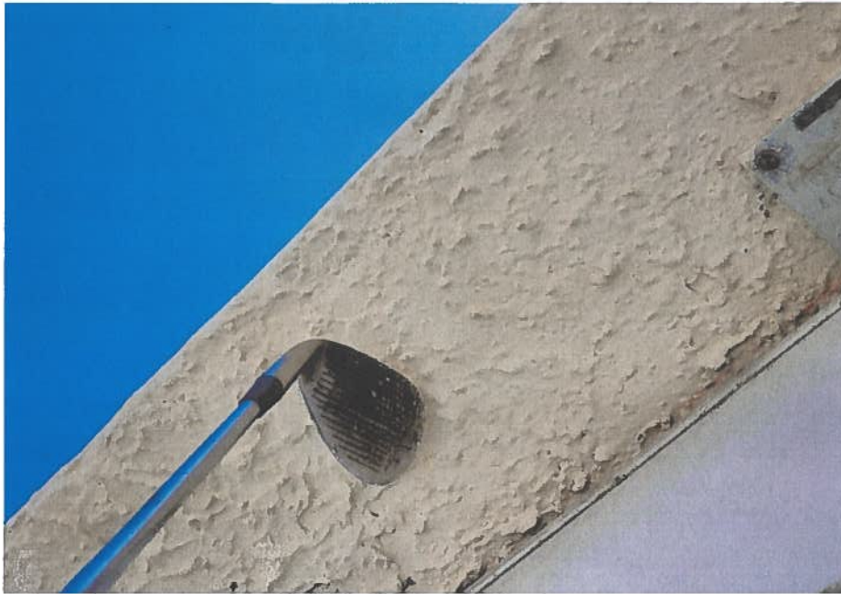
Figure A- 9: Typical delaminated area at balcony slab edge.
