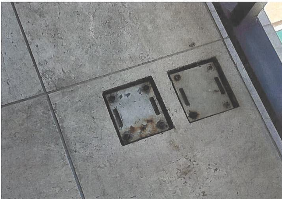
Figure A- 18: Observation of tiles with openings that allows water intrusion on the balcony surface.
