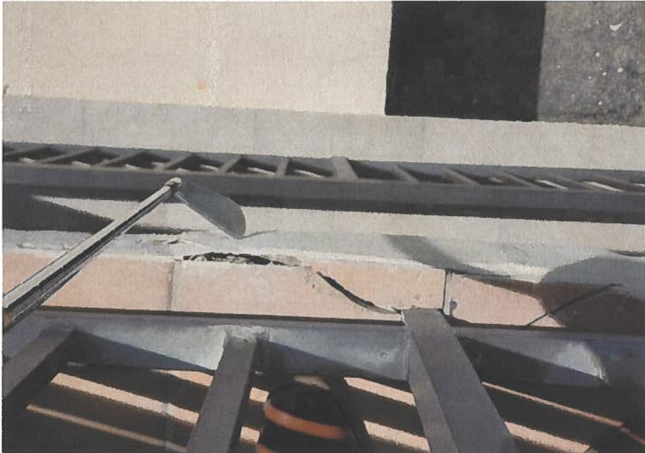
Figure A- 22: Typical spalling area at slab edge with cracked tiles
