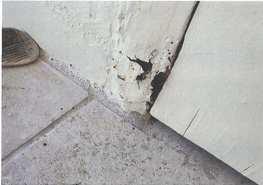
Figure A- 13: Typical rusty metal at the door frame on balcony storage.
