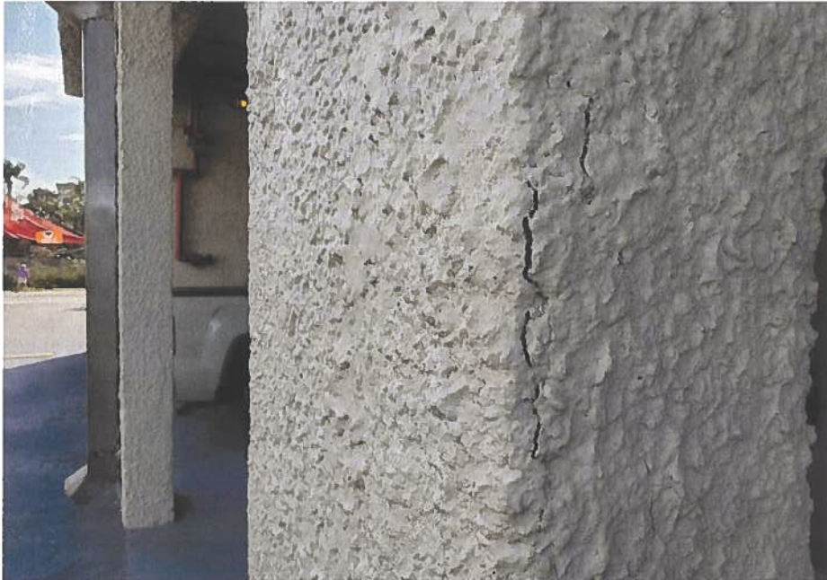
Figure A- 42: Typical vertical hairline stucco cracking at the column side.
