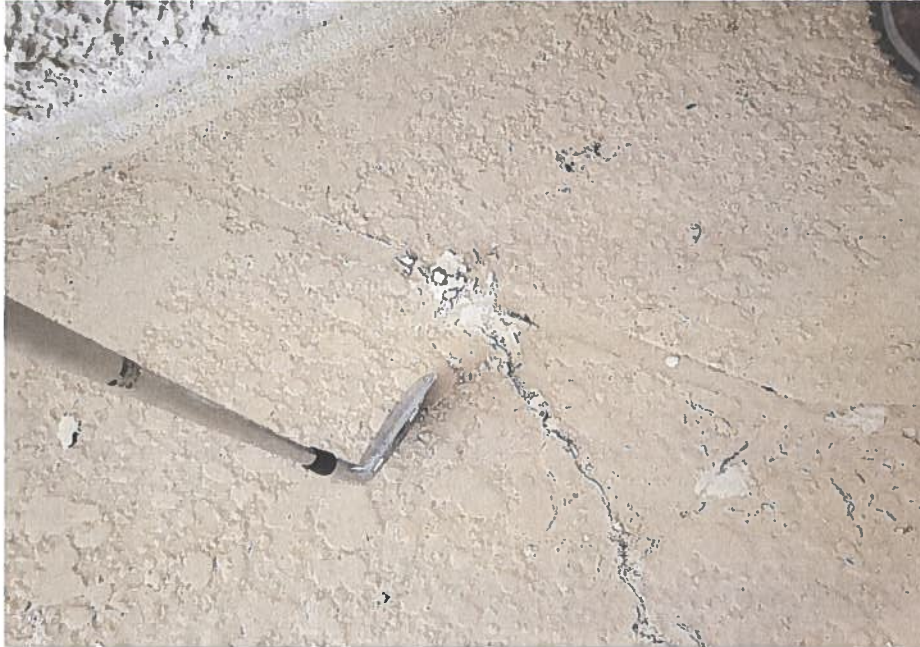
Figure A- 35: View of worn hallways waterproofing membrane
