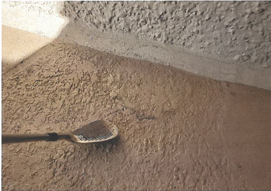
Figure A- 33: Typical spalled area at corridor surface.
