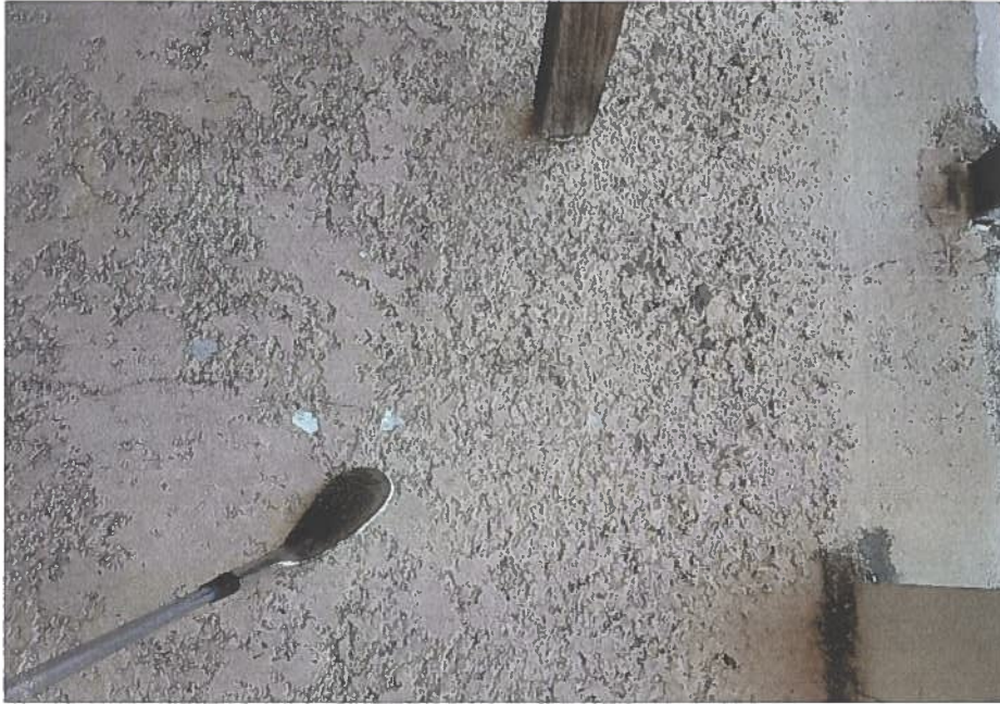
Figure A- 15: Typical hairline cracking on top of concrete slab on balcony surface.
