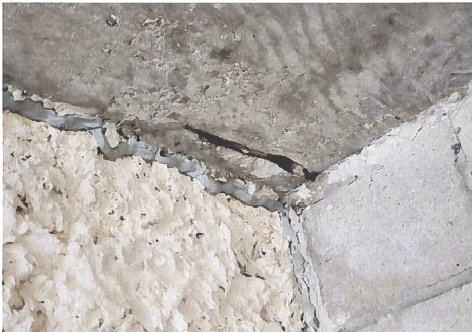
Figure A- 44: Spalling with reinforcement corrosion and exposed at the elevated slab on pump room ceiling.
