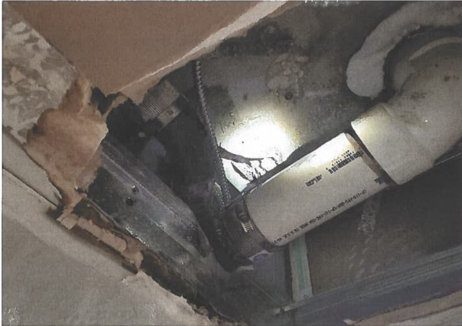
Figure A- 27: Unit #402 with concrete damage from leaks from the upper unit.
