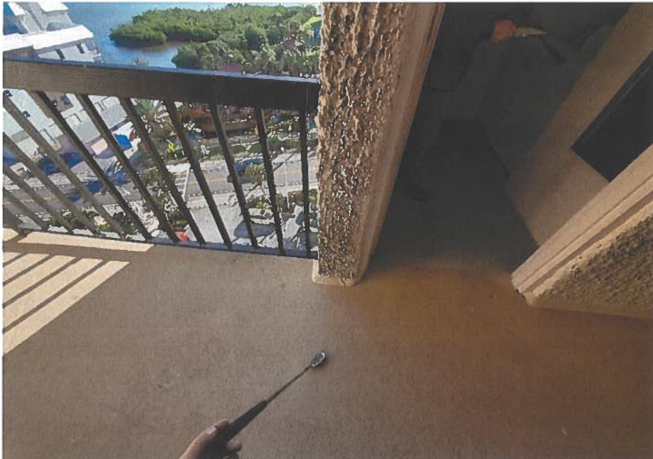
Figure A- 30: Typical delaminated area in front of laundry entrance.
