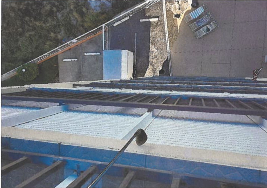
Figure A- 21: Typical delaminated area at slab edge.
