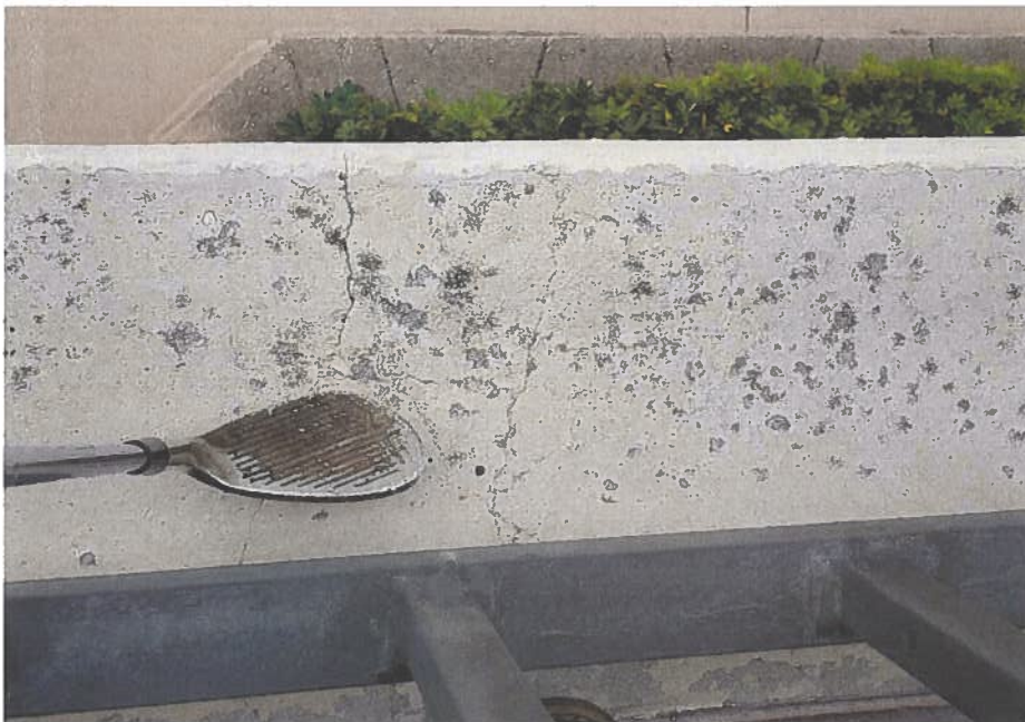
Figure A- 40: Typical cracking around slab edge.
