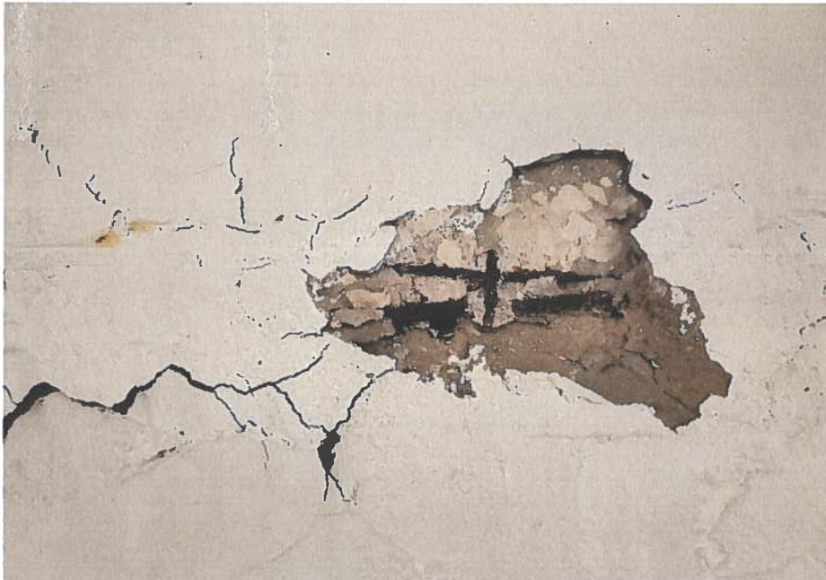
Figure A- 6: Observation of 1SF of concrete spalling and rebar exposure at the wall of communications room.
