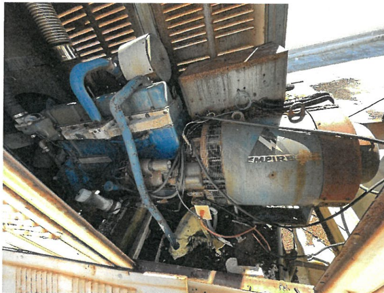
Figure 15: Rusty Generator at Roof of Building 19508
