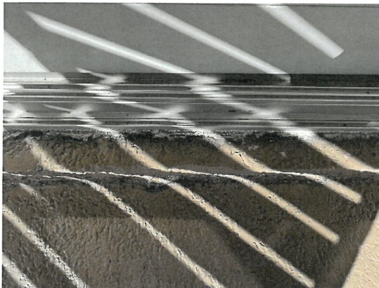
Figure 8: Sliding Glass Door Sealant Deteriorating
