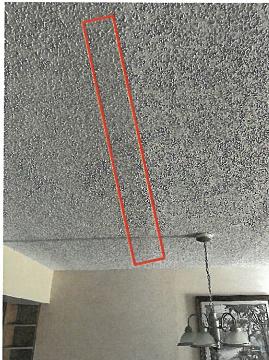
Figure 1: Hollow Core Precast Crack in Ceiling, Unit 101
