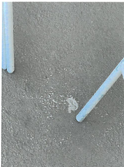
Figure 10: Visualization of Deteriorating Balcony Deck Coating
