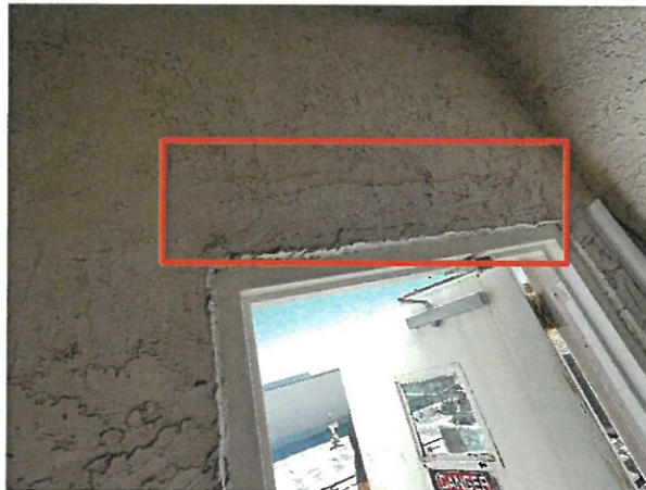
Figure 17: Visual of Spalling at Roof Access Door Lintel 19508
