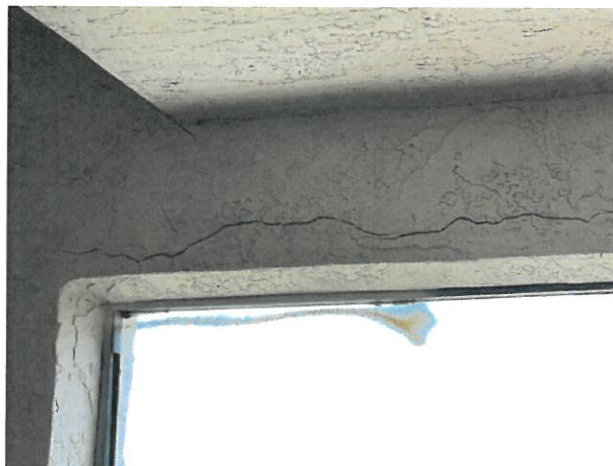
Figure 18: Visual of Spalling / Crack of 4 th Floor Landing South Stairwell of 19509
