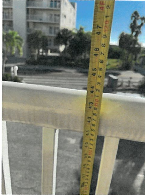
Figure 11: Visualization of Guard Rail Being to Code Vertically
