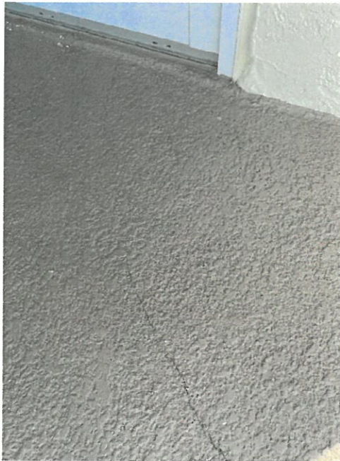
Figure 9: Visualization of Cracking at Balcony Deck
