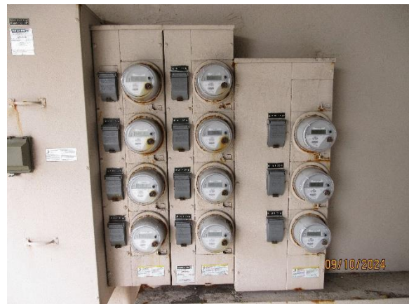
Close-Up - Moderate Corrosion Present
