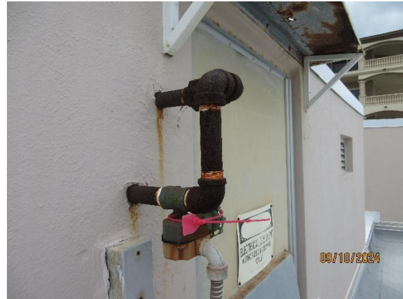
Corrosion at Fire Sprinkler Pipe Roof
