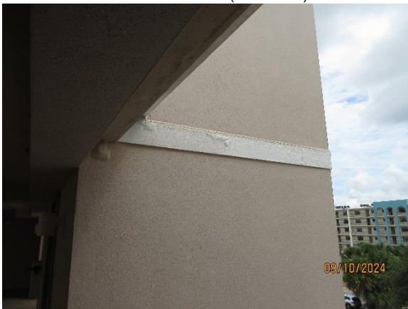
Paint Bubbles at Elevator Tower Band
