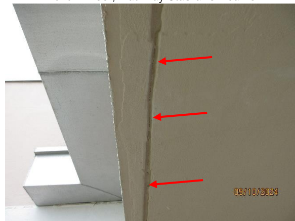
Close-Up Crack at Slab Edge/Drip Edge
