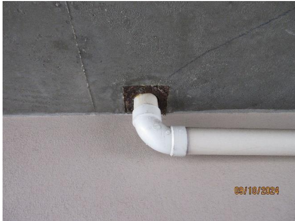
Close-Up Corrosion at Plumbing Penetration
