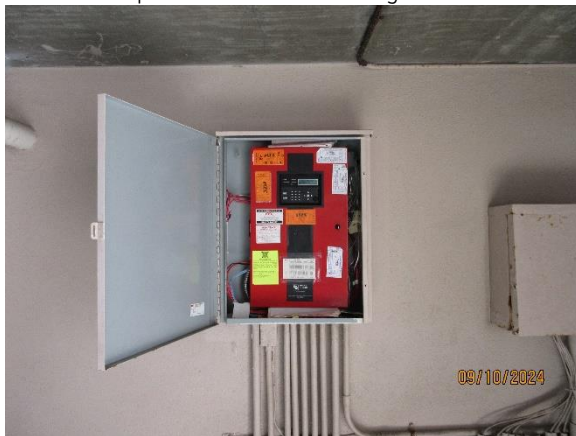
Fire Alarm System Control Panel
