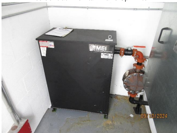
Hydraulic Elevator Power Unit
