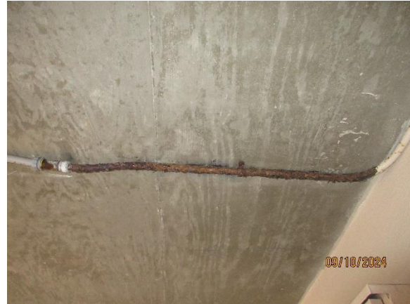
Corrosion at Conduit Garage
