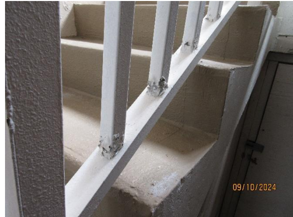
Damage to Railing Pickets at Stairs
