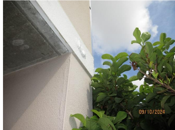
Close-Up Paint Bubble NE Garage Entrance
