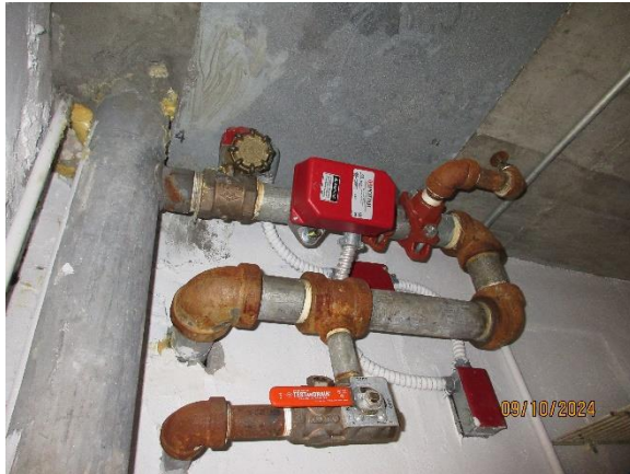
Fire Sprinkler Plumbing at Utility Closet
