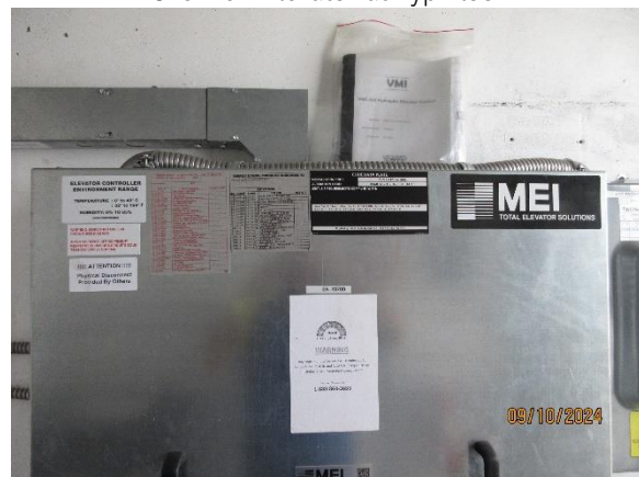
Hydraulic Elevator Control
