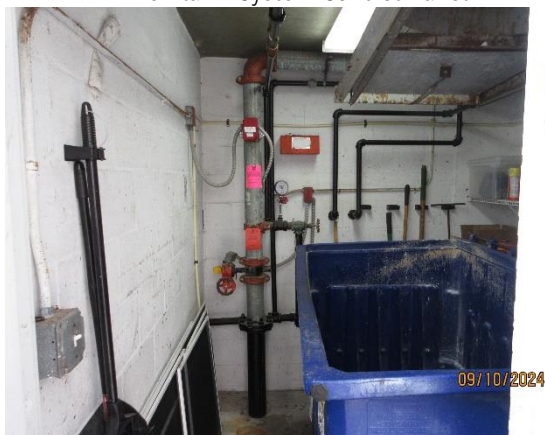
Fire Sprinkler Pipe
