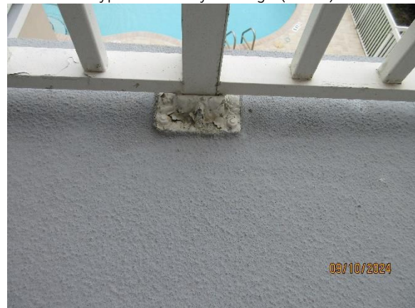
Railing Coating in Poor Condition at Base Plate
