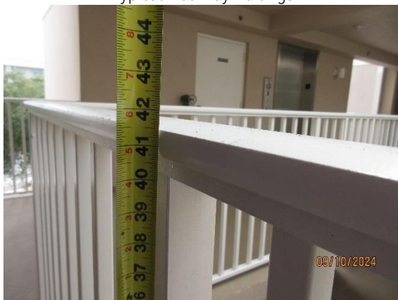
Walkway Railing Measurement
