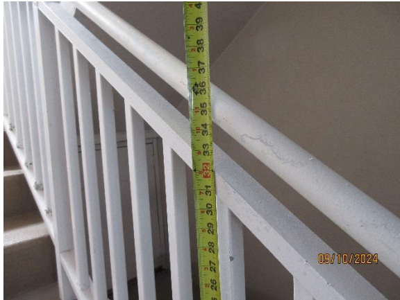
Stair Railing Measurement
