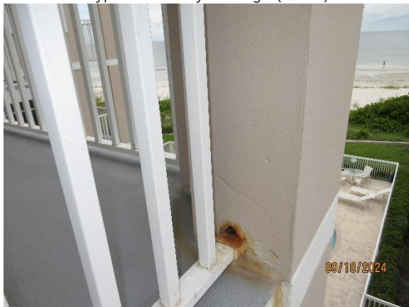
Corroded Fastener at Balcony Railing
