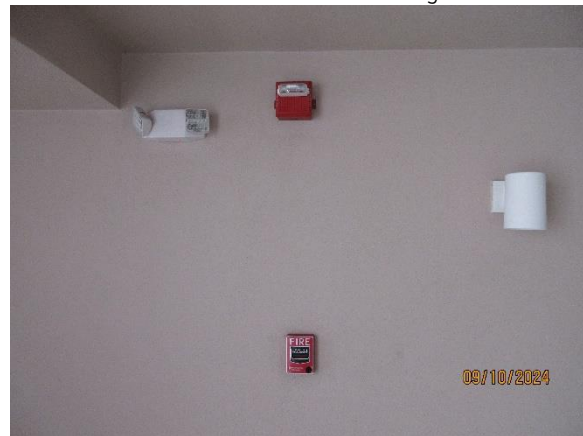
Typ. Pull Station, Flasher, Sounder, Emergency Lights
