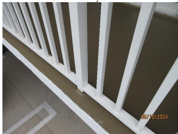
Close-Up New Waterproofing at Railing Post Pocket
