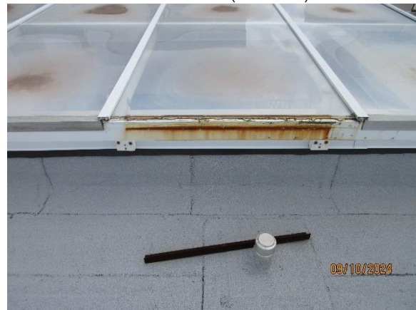
Corrosion and Damage to Steel Angle at Panel Edge
