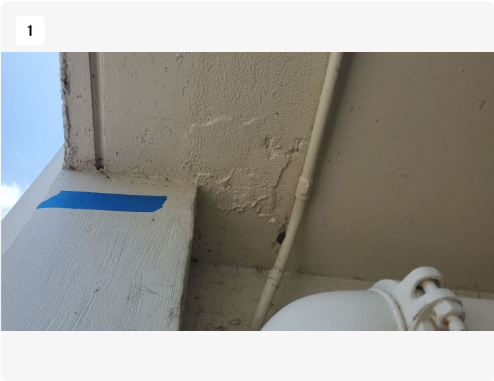
Overhead spall.
