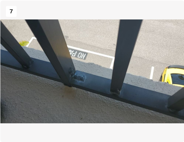
Supplemental clips on rail system
