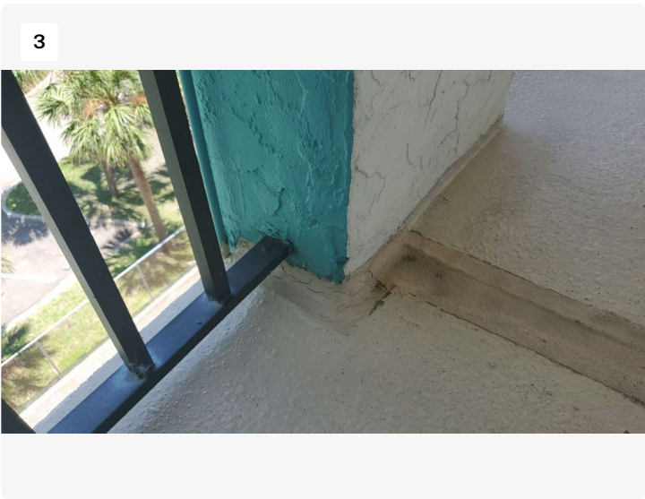
Cracking in expansion joint sealant coating.
