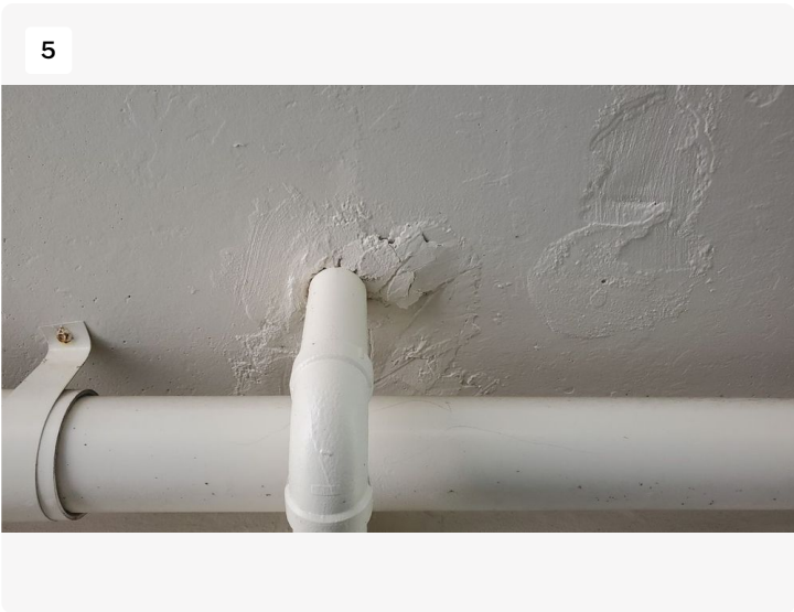
Overhead spall
