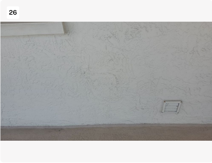
Previously repaired wall cracks
