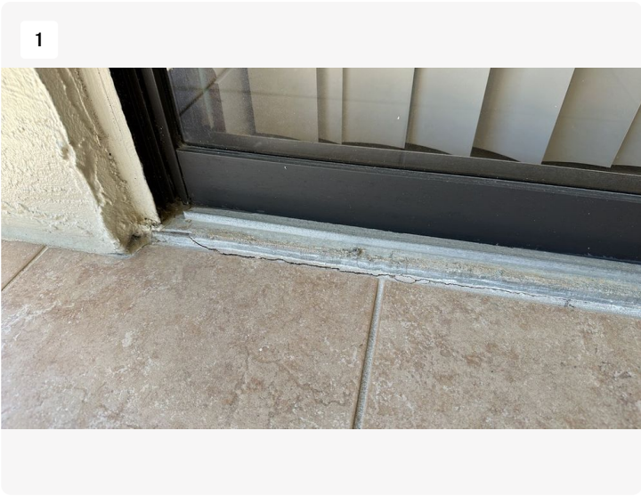
Crack in tile grout beneath sliding glass door track.
