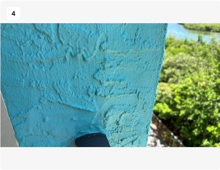
Crack in column stucco
