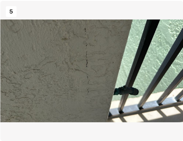
Crack in column stucco
