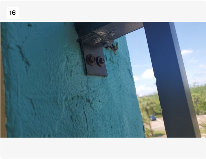
Corroded clips
