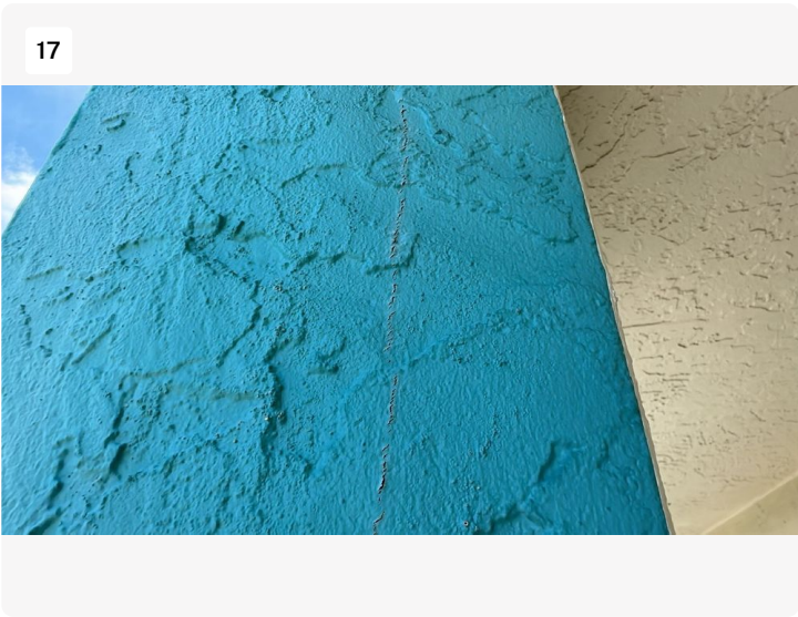
Crack in column stucco
