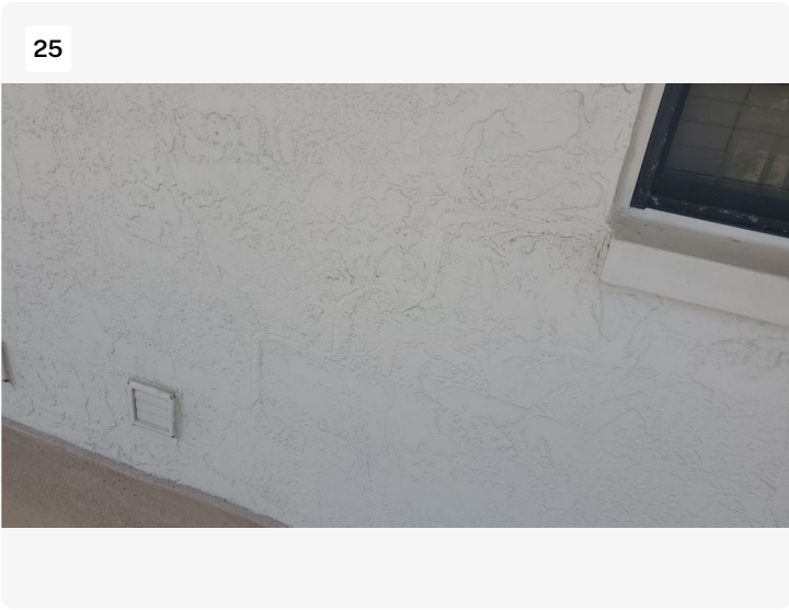
Previously repaired wall cracks
