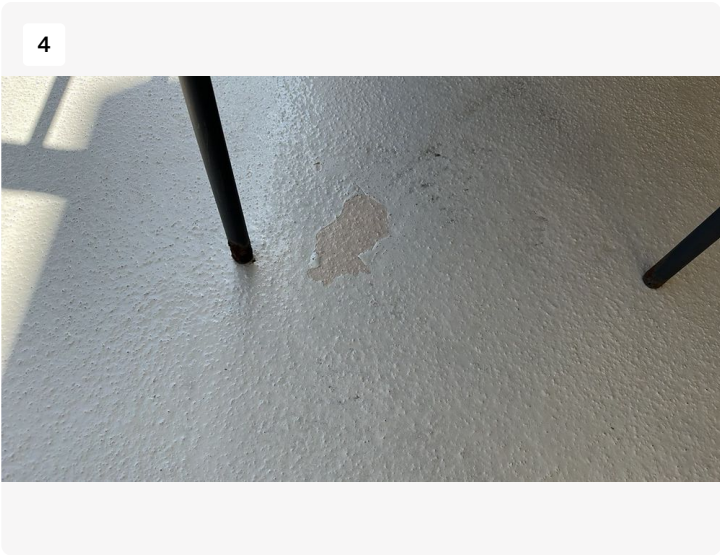
Peeling of urethane balcony coating
