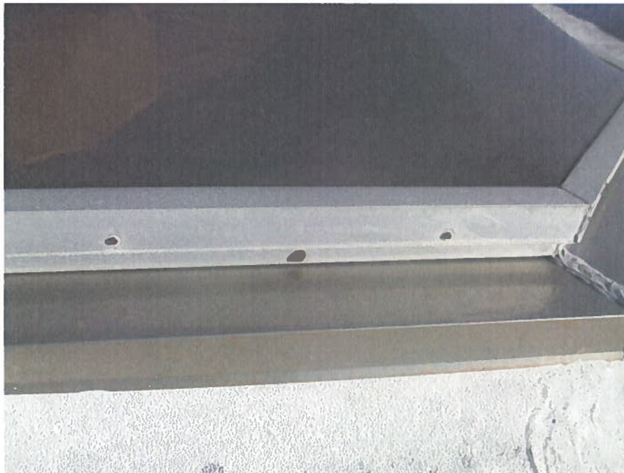
Photo #8 – Rusty fastener at solar opening
