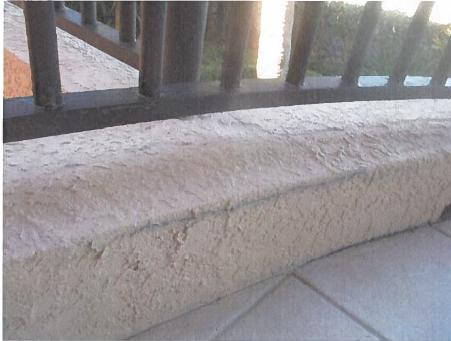
Photo #31 – Delaminating stucco at the balcony
