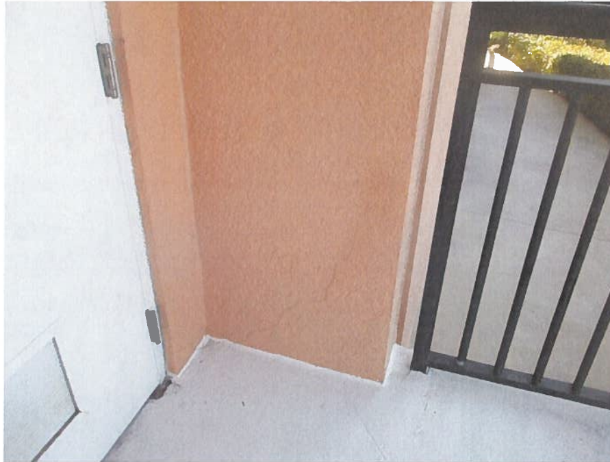
Photo #23 – Cracks at stucco and at wall to slab transition
