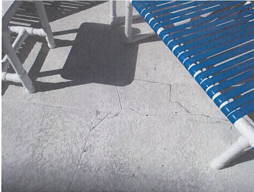
Photo #21 – Cracks and spalls at the pool plaza slab
