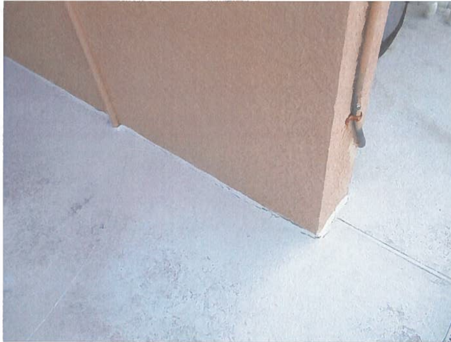
Photo #25 – Failed sealant
