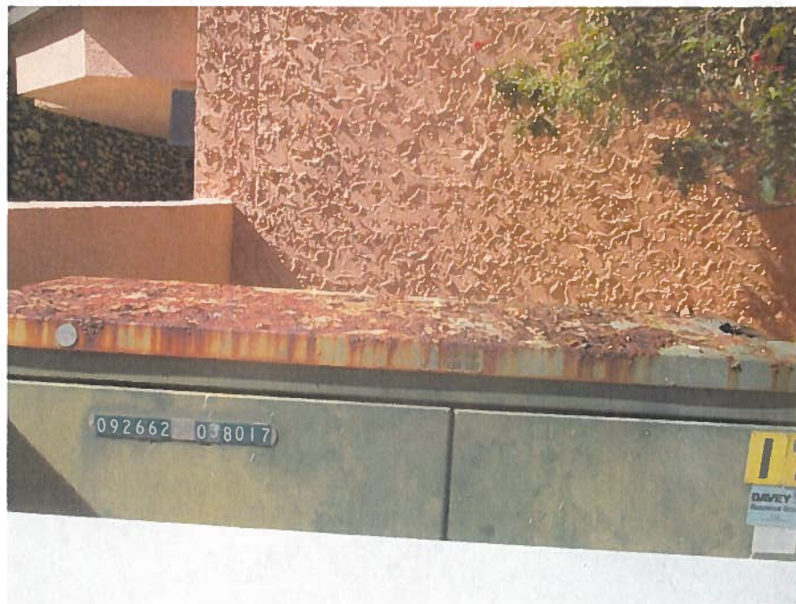
Photo #28 – Rusted electric panel
