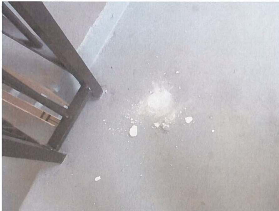
Photo #12 – Landing painted over built-up efflorescence residue
