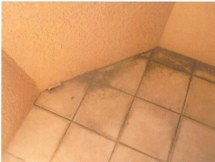
Photo #32 – Pounding water on the small balcony
