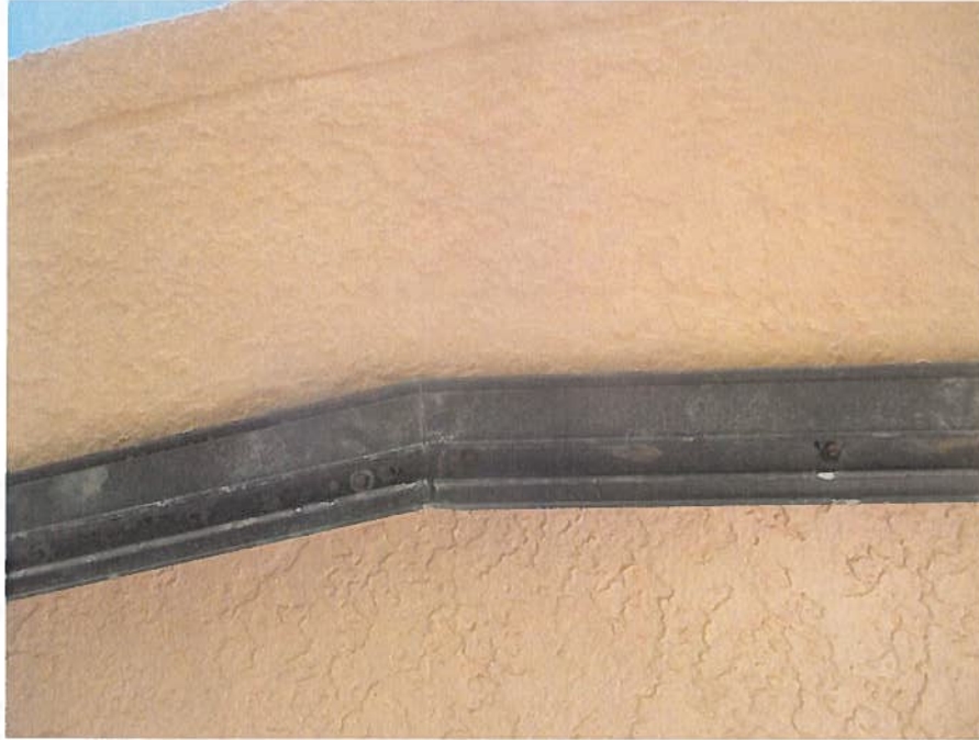
Photo #45 – Rusted screws attaching balcony storm shutter
