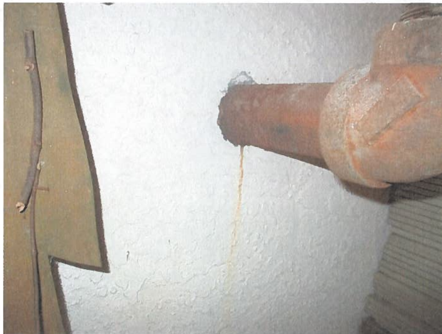
Photo #16 – Galvanized pipe (fire protection system) rusting at the exterior wall
