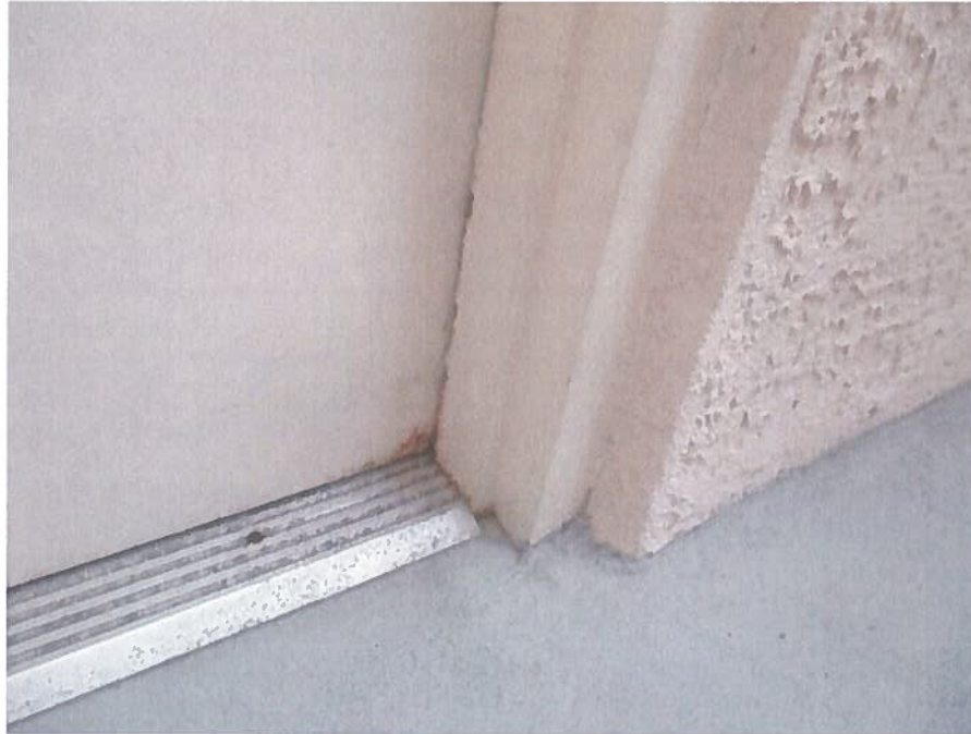
Photo #15 – Rusted base of steel wall
