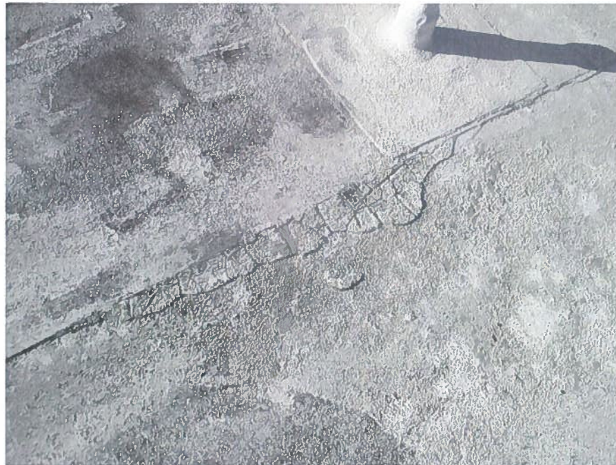
Photo #10 – Roof matt transition cracked.
