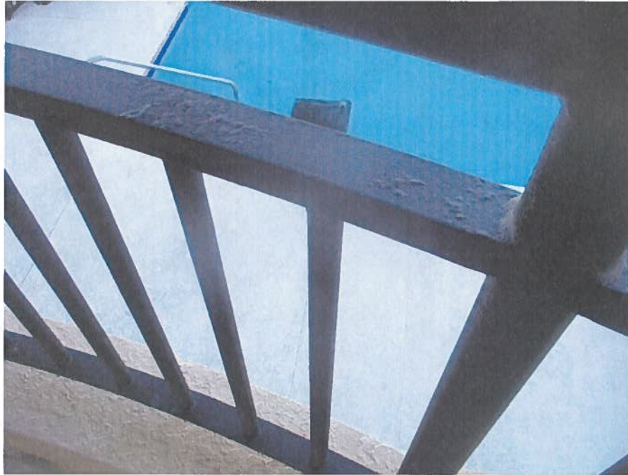
Photo #33 – Railing with some paint peeling
