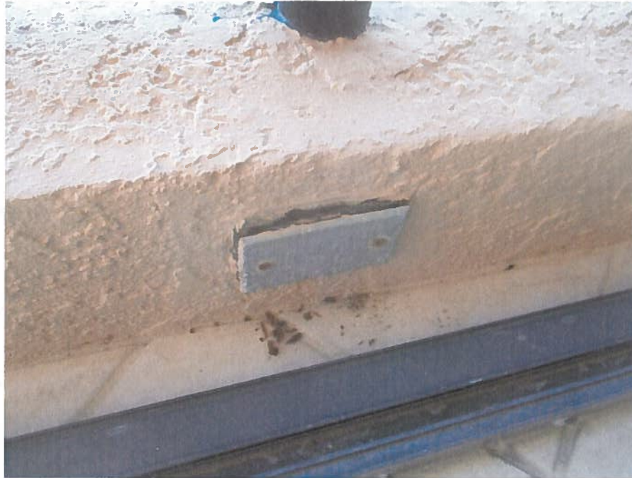
Photo #39 – Electric with corrosion
