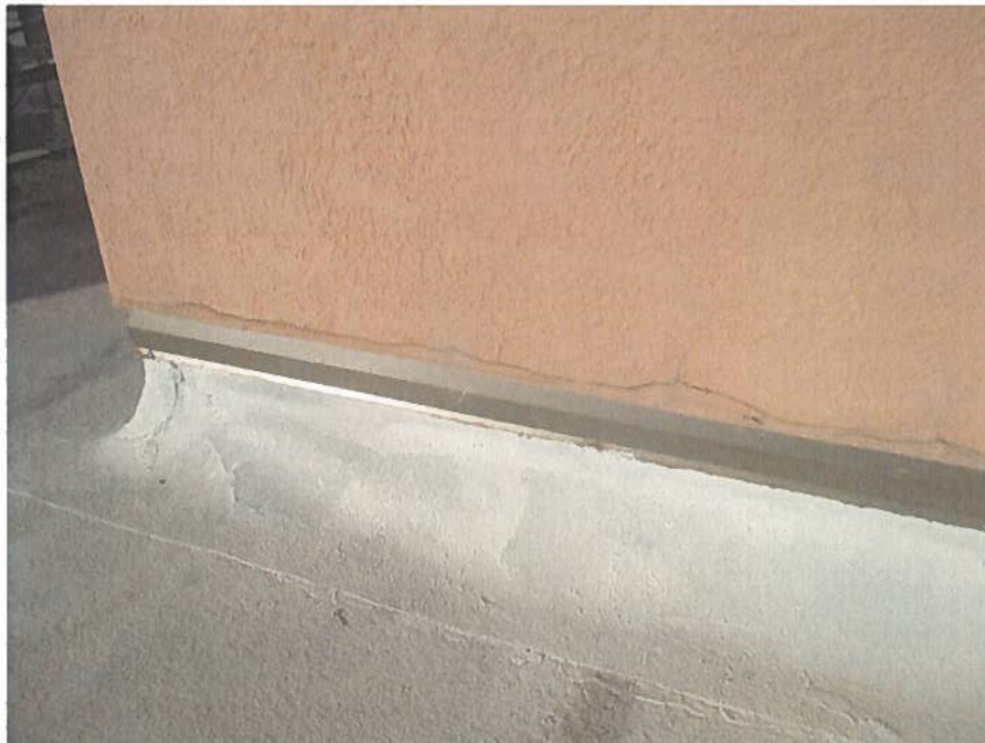
Photo #2 – Stucco delamination and crack at the transition with the flashing at bottom of walls at the west stair tower and elevator penthouse
