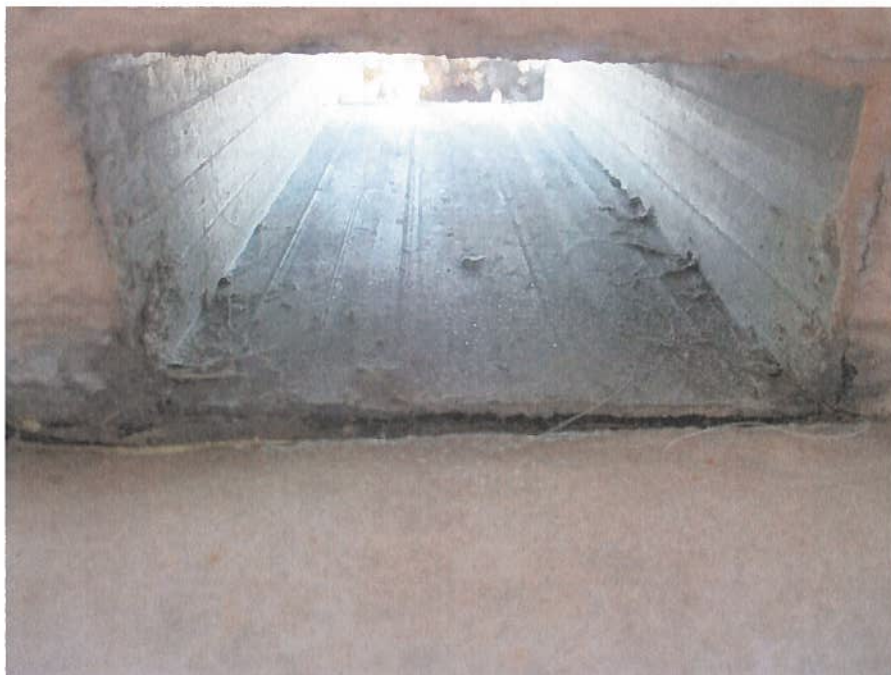
Photo #30 – Gap between scupper and tile
