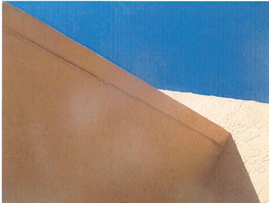
Photo #38 – Edge spall at the small balcony
