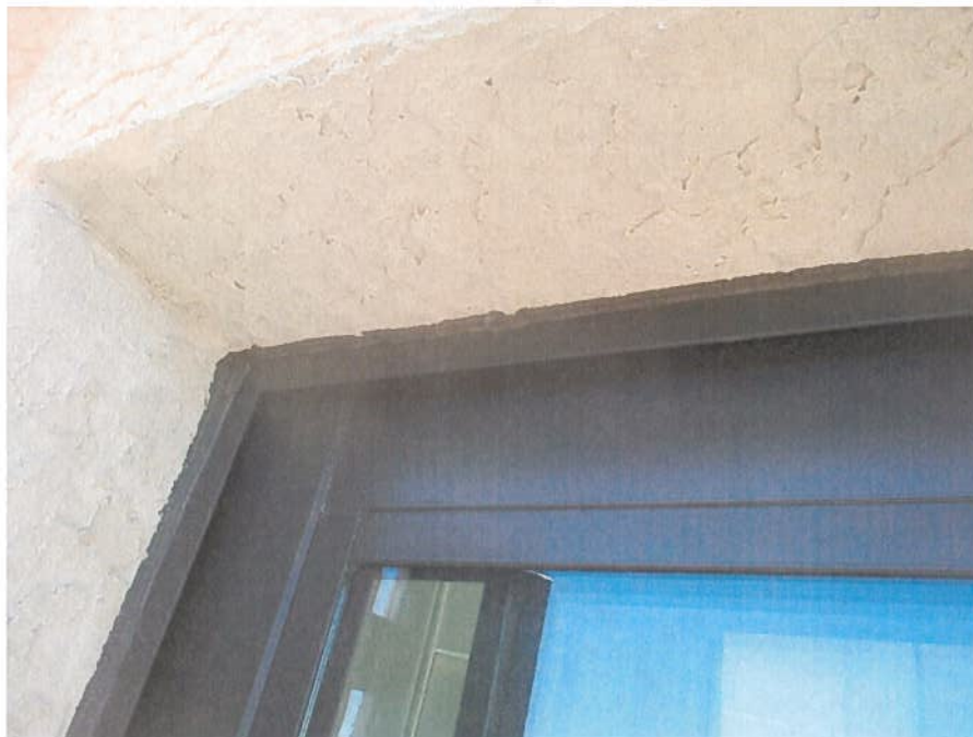
Photo #44 – Replaced SGD w/ bad stucco patch and failed selant
