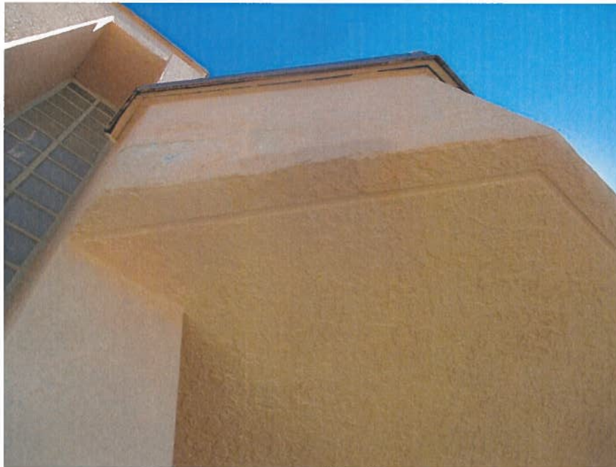
Photo #46 – Efflorescence at parapet above unit #501
