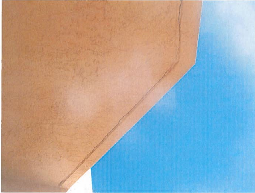
Photo #37 – Edge spall at the small balcony
