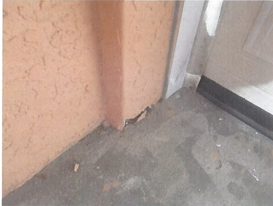
Photo #19 – Stucco failed at transition with slab
