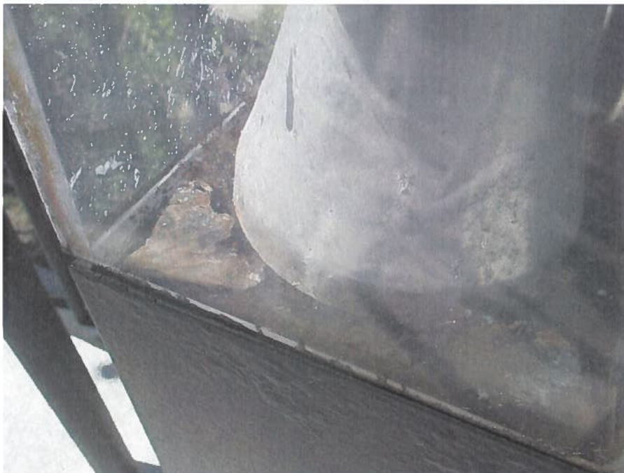
Photo #22 – Decorative lamps at pool plaza rusted. That includes the sections into the concrete slab
