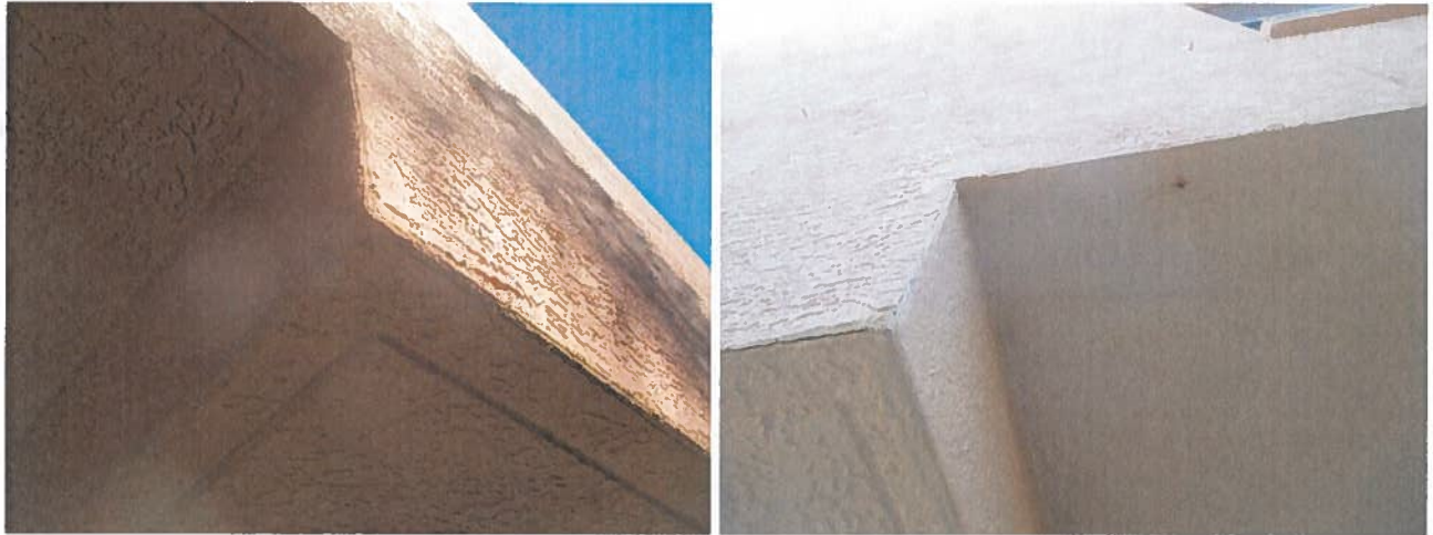
Photo #27 – Cracks at the transition of different materials
