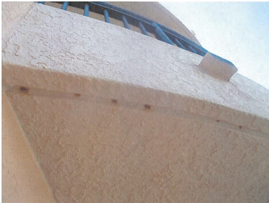
Photo #26 – Shallow reinforcement under stucco
