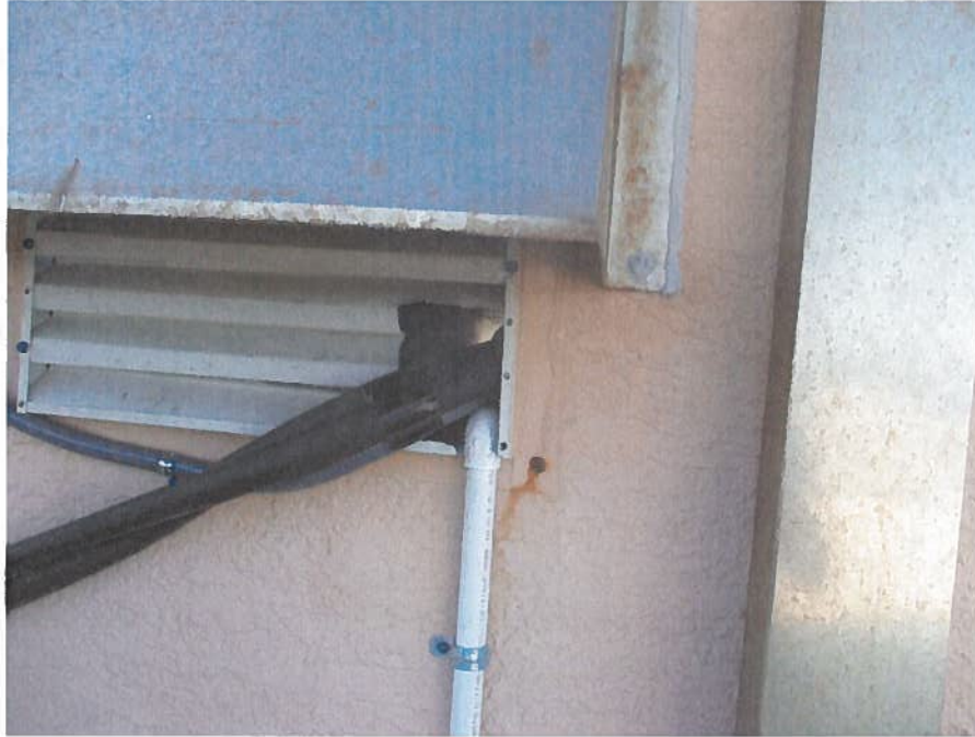
Photo #3 - Rusty fastener at the elevator penthouse louver.
