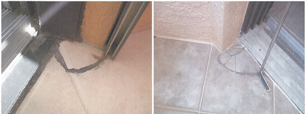
Photo #42 – Typical cracked tile under small balcony sliding glass door
