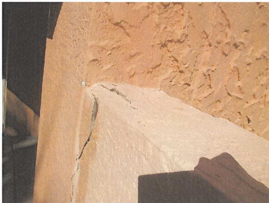
Photo #18 – Sealant failed at expansion joint
