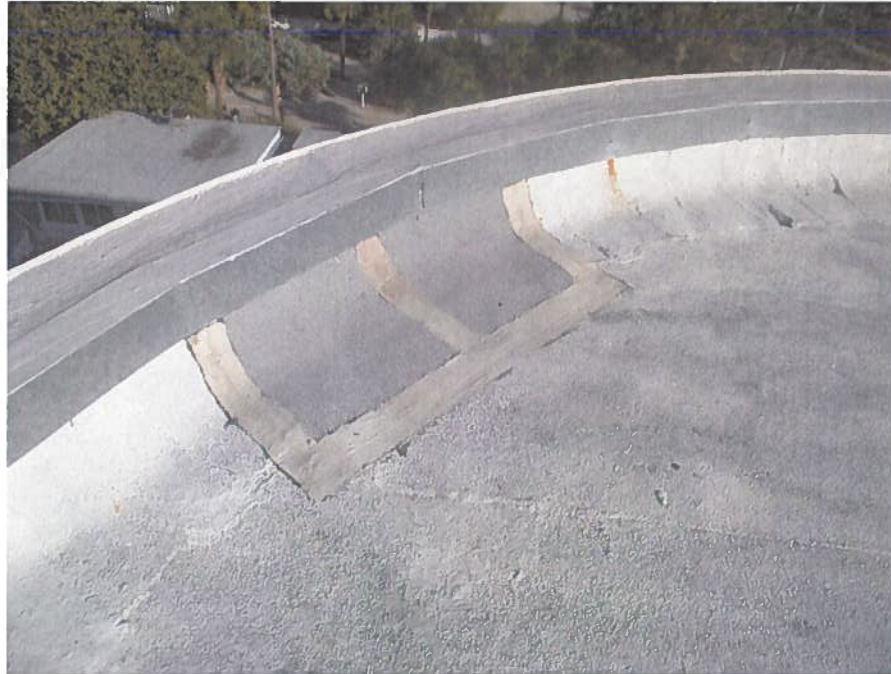
Photo #7 – Roof coated and previously patched
