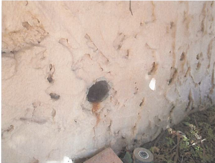
Photo #17 – Galvanized pipe rusting at the exterior wall
