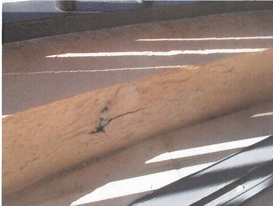
Photo #41 – Damaged stucco at balcony curb
