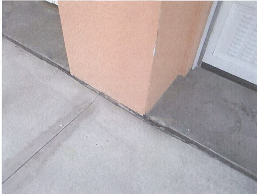
Photo #29 – Failed sealant at transitions
