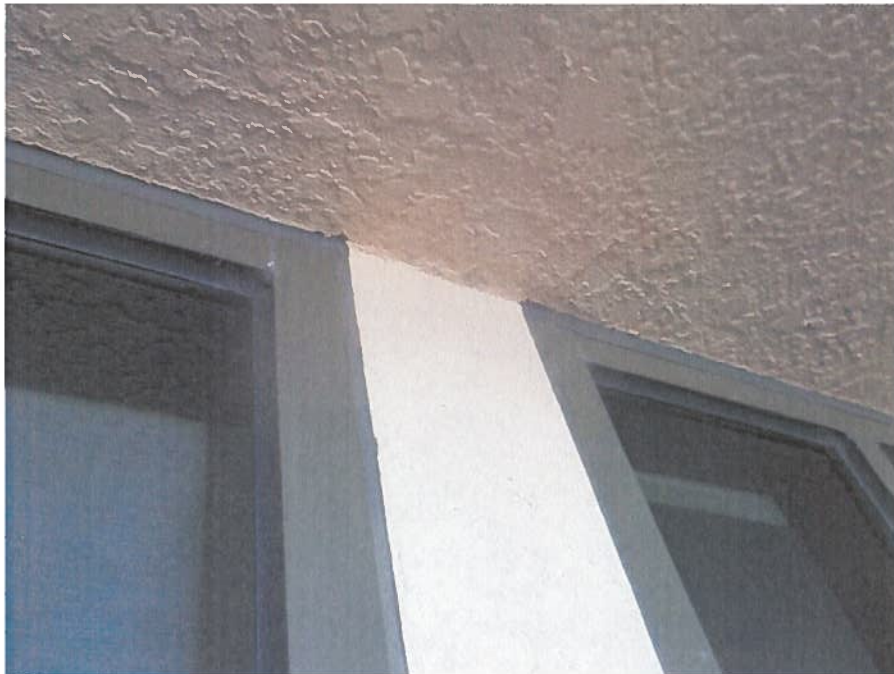
Photo #36 – Typical good sealant around windows
