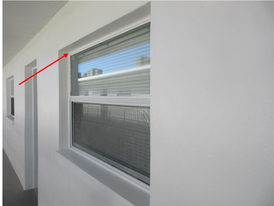
Photo #9 – Recently Updated Exterior Windows (2018) with New Perimeter Sealant Installed. (TYP)
