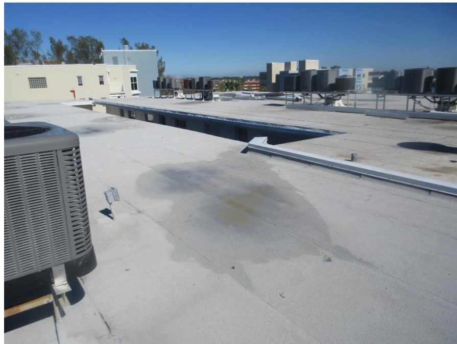
Photo #6 – Overview of Main Roofs Covered with Two-Ply Modified Bitumen Membrane.
