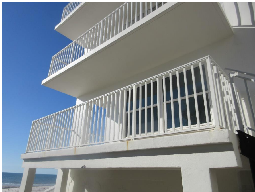
Photo #8 – Overview of Aluminum Railing on Private Unit Balconies. (TYP.)
