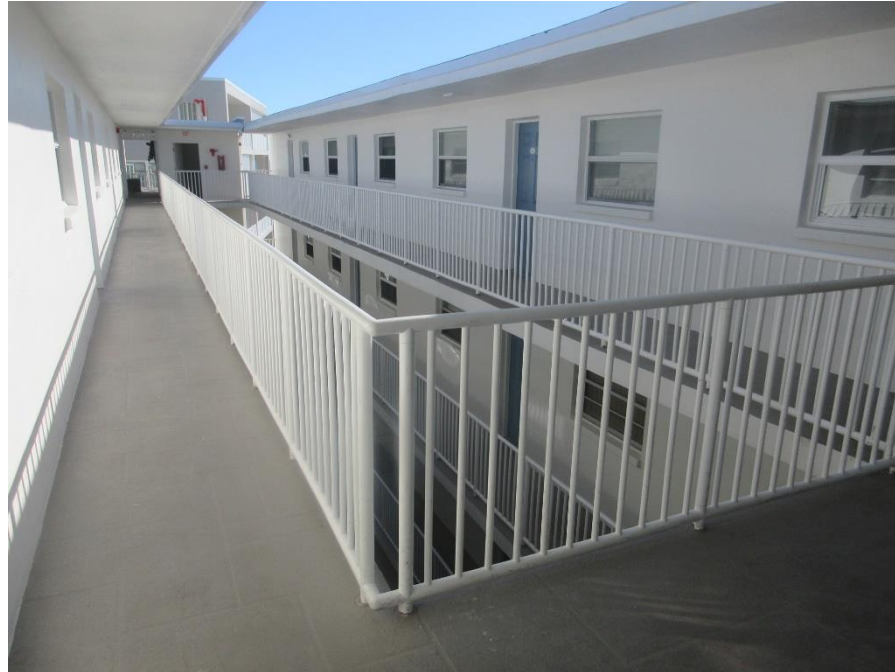
Photo #7 – Overview of PVC Railings on Walkways. (TYP.)
