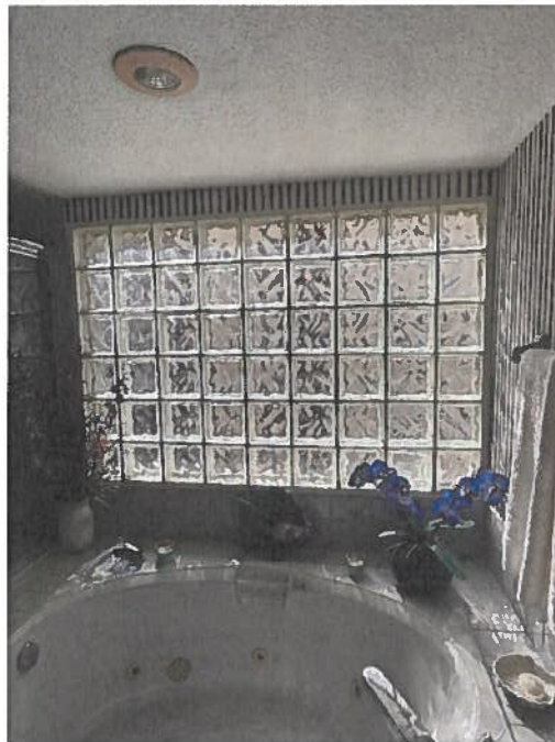
Glass Blocks Typical in Master Bathroom
