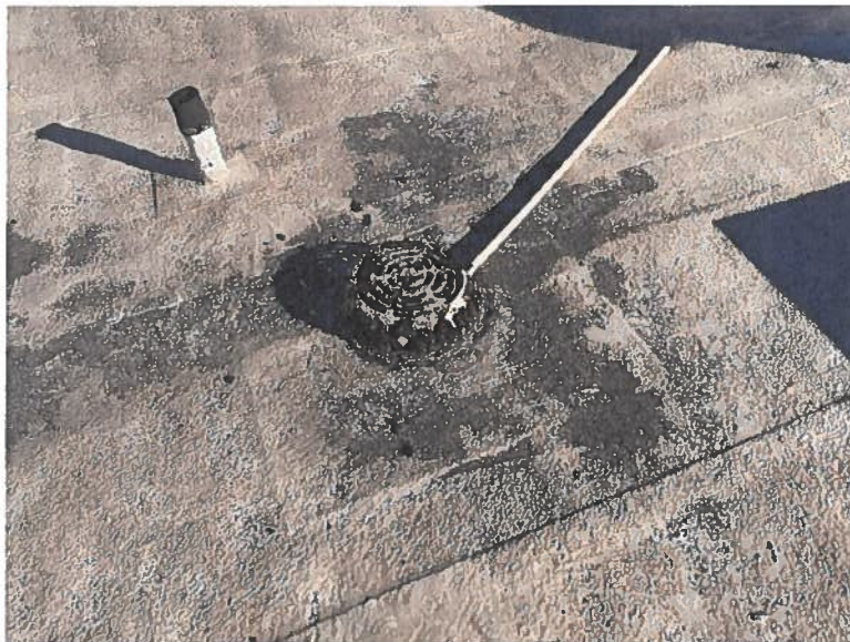
Roof Drain Cover with Significant Corrosion
