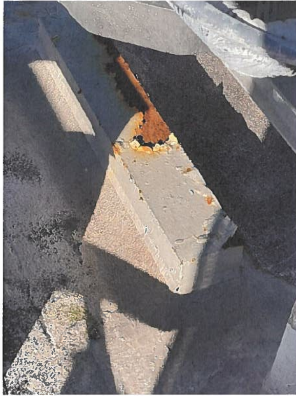
Old Metal Flashing at Existing Curb Corroding
