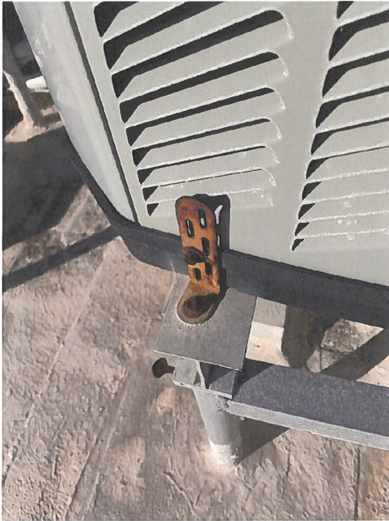
Hurricane AC Strap Observed to be in Poor Condition
