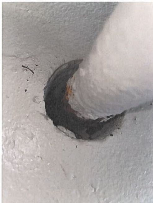
Visualization of Sprinkler Line Missing Fire Caulking
