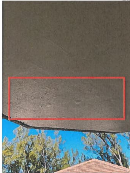
Bubbling Painted Finish Observed at Balcony Ceiling
