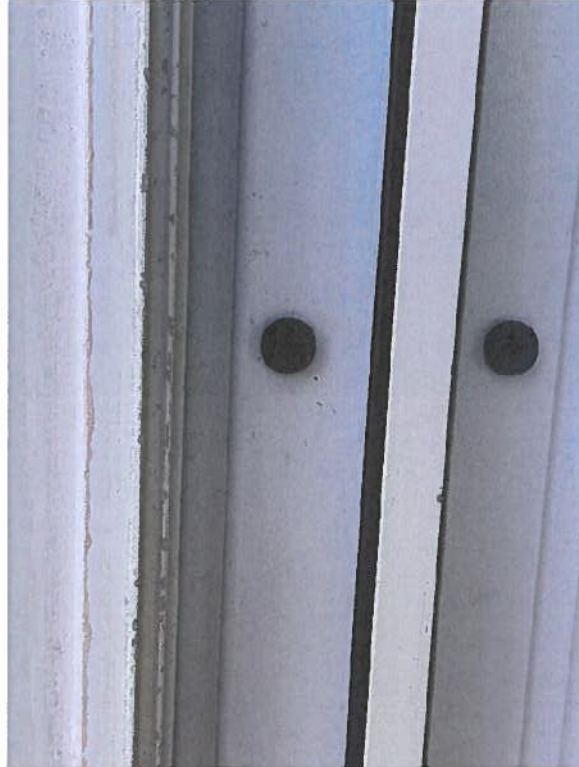
Observed Fasteners Rusting at Sliding Glass Doors
