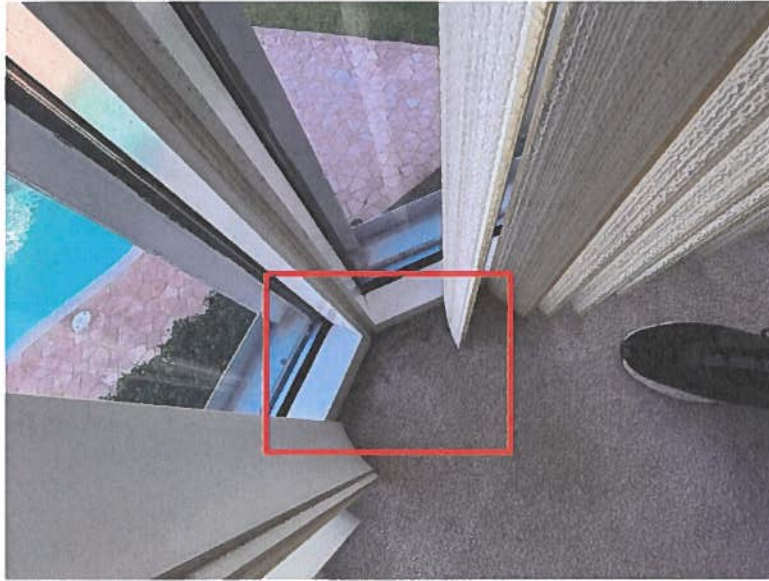
Water Stains Typical in Carpet at Master Bedroom Window
