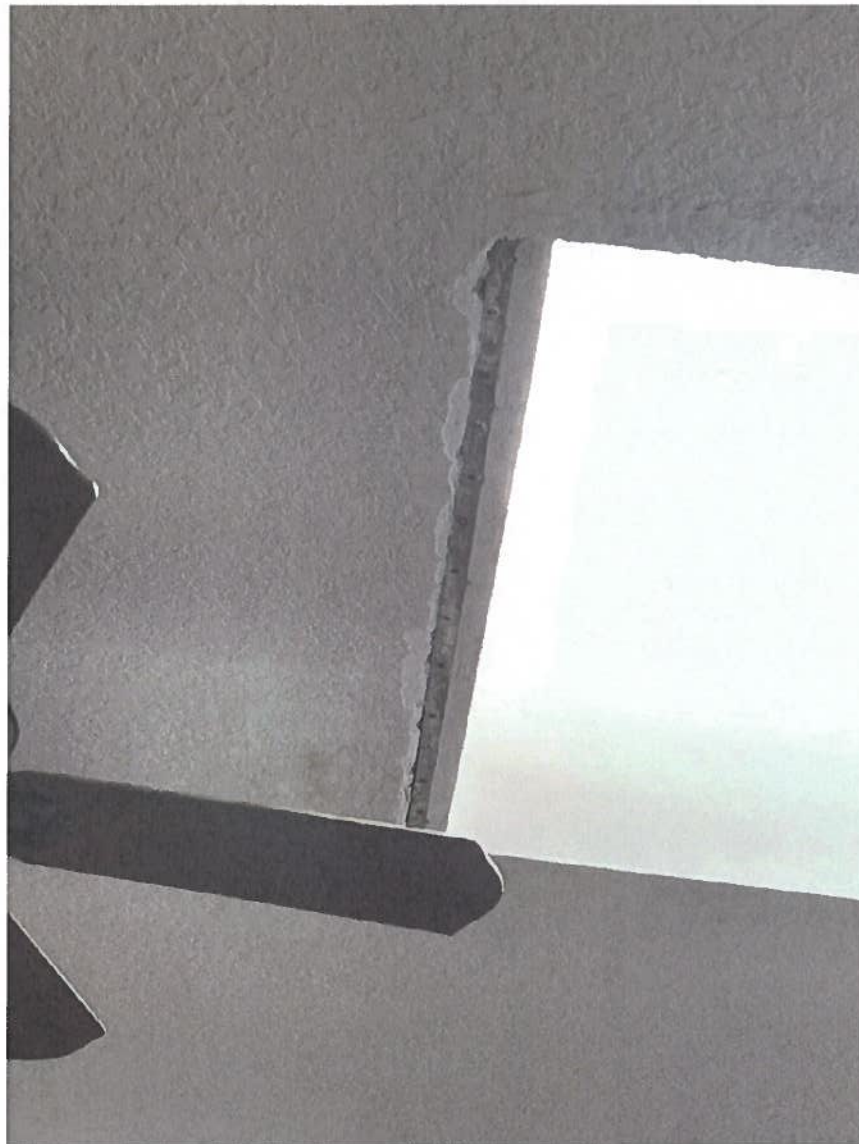
Drywall Damage at Ceiling Skylight, Unit 502
