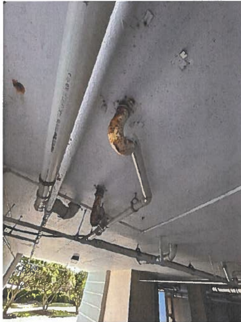
Metal Pipes Showing Signs of Oxidizing and Rusting
