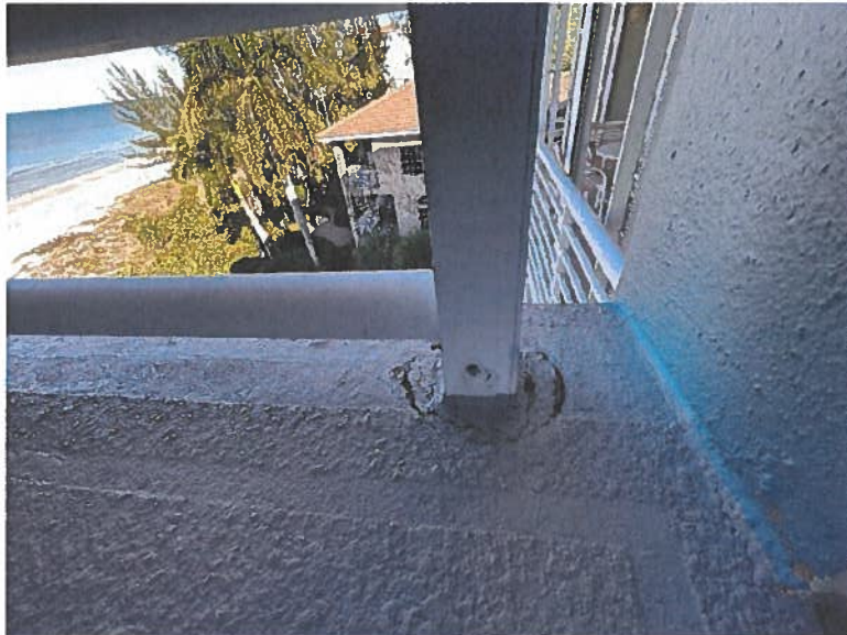
Cracking Sealant at Handrail in West Stairwell
