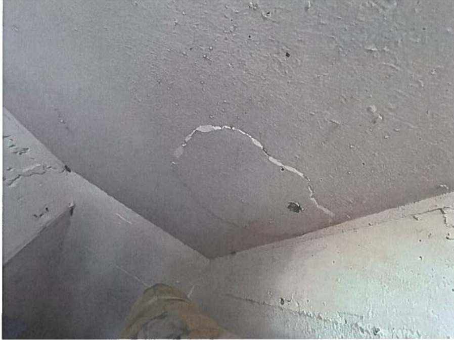
Spall Occurring Under West Stairwell
