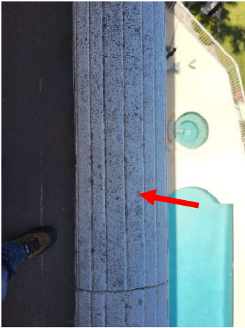
Photo 7.4.1 – Unit 503 - Handrail Balcony paint failure and mild corrosion.
