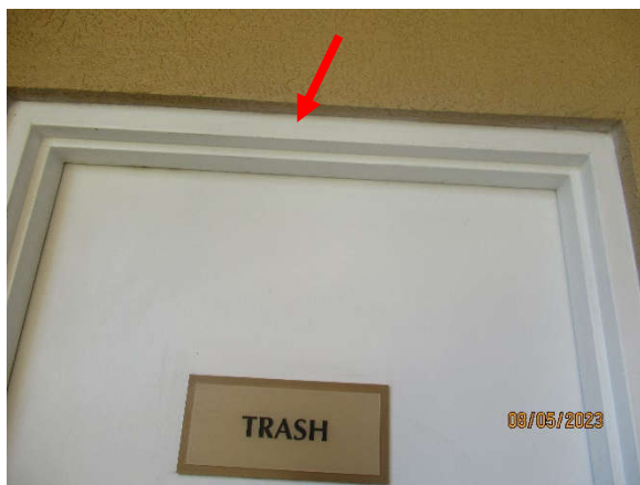
Photo 7.3.a.3 – Level 2 nd trash room paint crack and peeling off.
