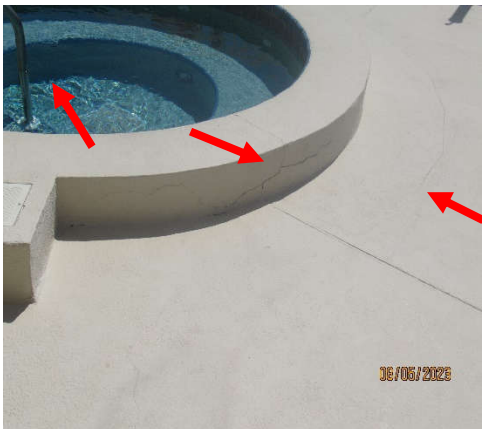
Photo 7.7.5 – Pool area - Concrete crack in the pool slab on grade. Concrete cracks in the spa curb.
