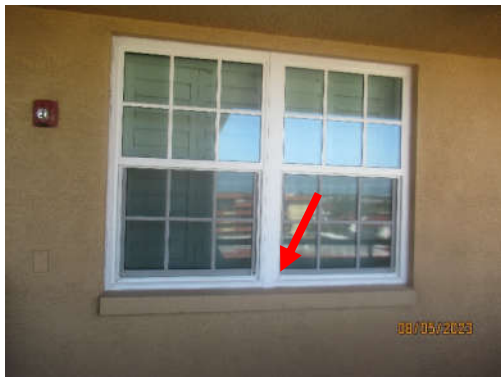
Photo 7.3.b.1 – Front corridor (East Façade) Level 4 th window perimeter sealant showing substrate and window frame separation
