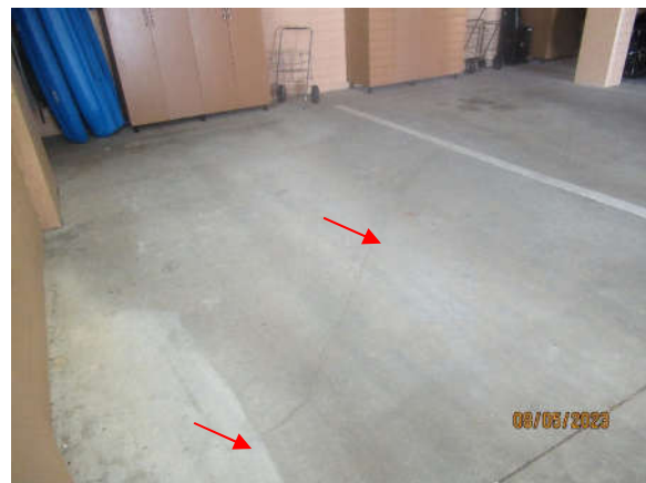
Photo 7.8.a.8 – Garage Level - Drying shrinkage cracks observed at the slab on grade.
