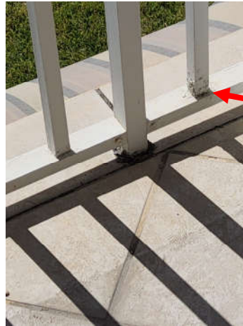
Photo 7.4.2 – Unit 101 - Handrail Balcony paint failure and mild corrosion.
