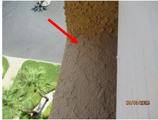
Photo 7.2.c.6 – Stairwell #2 stucco hairline crack.
