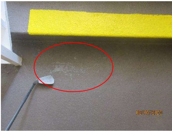
Photo 7.2.b.1 – Stairwell #2 – Waterproofing membrane peeling between 2 nd and 3 rd level
