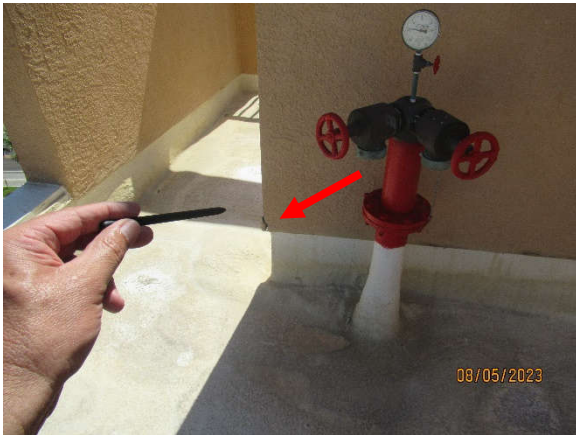
Photo 7.2.c.7 – Roof level vent shaft southeast corner – Stucco crack and de-bonded.
