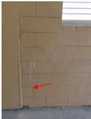
Photo 7.8.b.5 – Garage Level – Evidence of efflorescence was observed through some of the walls in the garage level.
