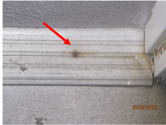
Photo 7.3.a.6 – Level 2 nd trash room corroded fastener at the door threshold.
