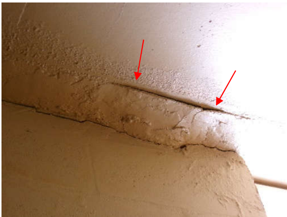
Photo 7.1.a.5 – Garage Level – Delaminated area observed at the ceiling slab.
