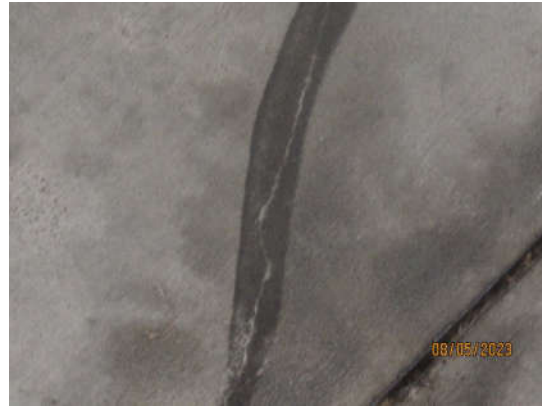
Photo 7.8.a.4 – Garage Level - Drying shrinkage cracks observed at the slab on grade. The application of cementitious material to repair and seal the crack was observed.
