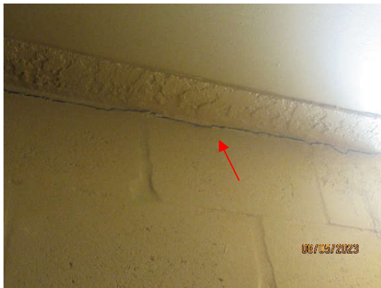
Photo 7.8.b.3 – Garage Level – Anticipated cracks in buildings and building materials typically result from restrained movement.
