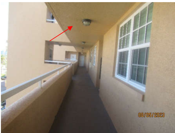
Photo 7.1.a.3 – Level 4 th Front Corridor – Sounding of the post-tense concrete slab did not reveal delaminated areas.
