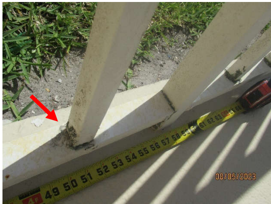
Photo 7.4.7 – Pool deck railing with paint weathered and mild corrosion.
