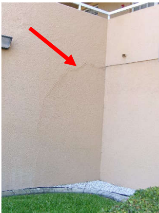
Photo 7.2.a.9 – East façade typical stucco cracked routed and sealed. The repair was observed to be in good condition.
