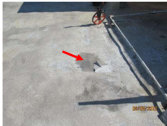
Photo 7.6.4 – Roof level – Roof patch repairs were observed to be detached and peeled off.
