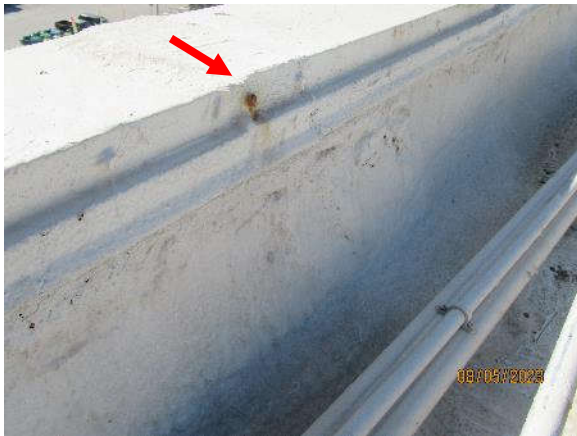
Photo 7.6.7 – Roof level – Corrosion in the cap flashing fastener.
