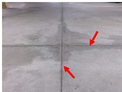
Photo 7.5.6 – Garage level saw cut contraction joint in good condition.
