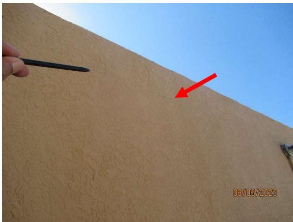
Photo 7.2.c.3 – Roof level stairwell #1 stucco horizontal crack.
