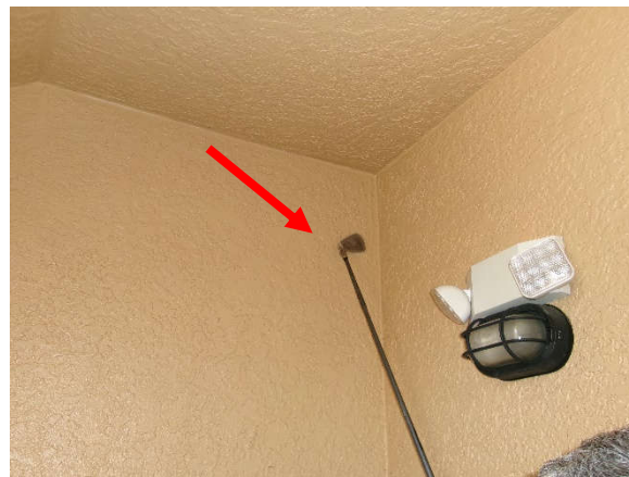
Photo 7.2.c.10 – Stairwell #1 Level 2 nd – Tapping revealed a hollow sound in the stucco.
