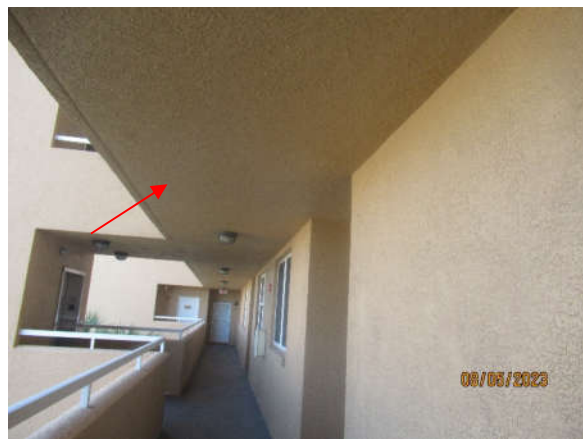
Photo 7.1.a.4 – Level 2 nd Front Corridor – Sounding of the post-tense concrete slab did not reveal delaminated areas.
