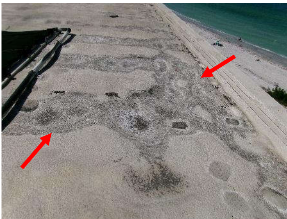
Photo 7.6.3 – Roof level – Uneven surface and evidence of temporary water ponding.
