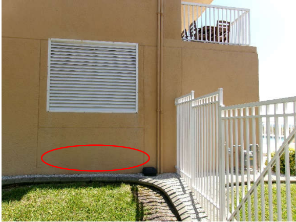
Photo 7.2.a.5 – North façade hairline cracks and evidence of efflorescence.
