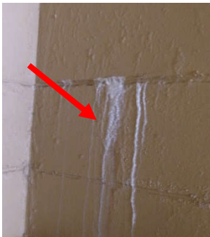
Photo 7.2.b.5 – Garage level – Evidence of efflorescence.
