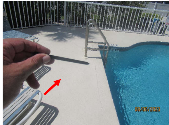
Photo 7.7.6 – Pool area – Concrete crack in the pool slab on grade. Likely between the slab on the grade and the pool wall.
