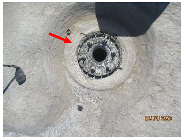
Photo 7.6.10 – Roof drain dome gate loss.
