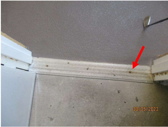
Photo 7.3.a.5 – Level 2 nd trash room corroded fastener at the door threshold.
