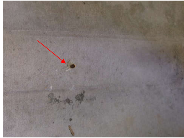
Photo 7.1.b.2 – Garage Level – Embedded rust metal at the slab on grade.
