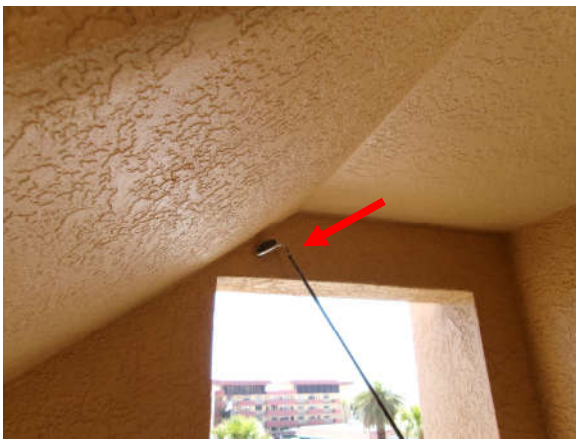
Photo 7.2.c.9 – Stairwell #1 Level 2 nd – Tapping revealed a hollow sound in the stucco.
