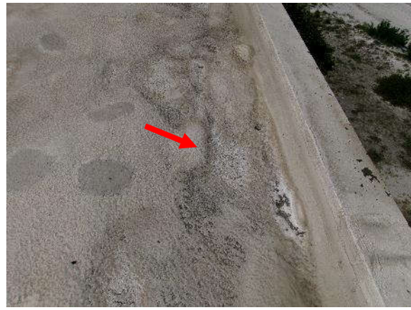
Photo 7.6.2 – Roof level – Uneven surface and evidence of temporary water ponding.
