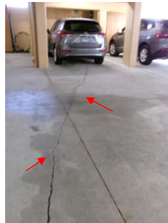
Photo 7.8.a.6 – Garage Level - Drying shrinkage cracks observed at the slab on grade.
