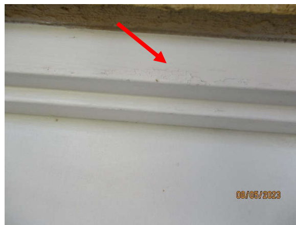
Photo 7.3.a.4 – Level 2 nd trash room paint peeling off.
