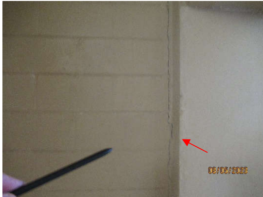
Photo 7.8.b.1 – Garage Level – Anticipated building cracks usually result from restrained movement in buildings and building materials.
