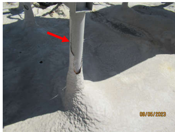
Photo 7.6.12 – Peeled off the coating in the rooftop structure base.
