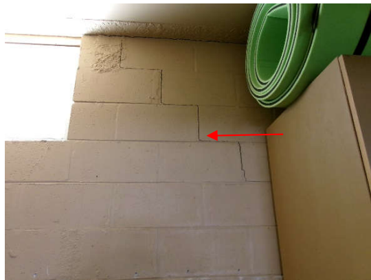
Photo 7.8.b.4 – Garage Level – Anticipated cracks in buildings and building materials typically result from restrained movement.
