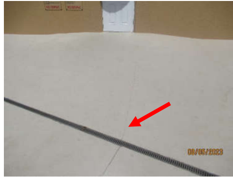
Photo 7.5.2 – Pool Deck - Visual assessment showed joint construction deficiencies such as cracks and de-bonding.
