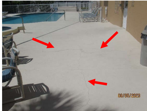
Photo 7.7.2 – Pool area - Concrete crack in the pool slab on grade.
