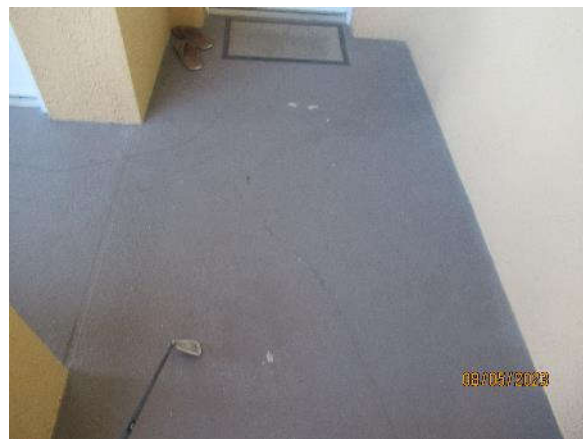
Photo 7.2.b.10 – Front corridor level 3 rd – De-bonding and peeling off the waterproofing membrane.
