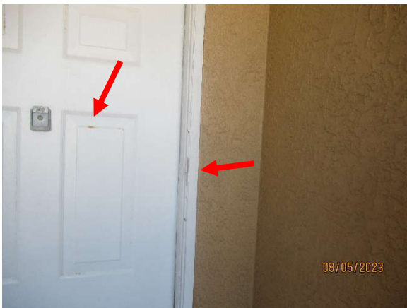
Photo 7.3.a.9 – Front corridor (East Façade) level 3 rd unit door showing rust stains, paint cracks, and peeling off.
