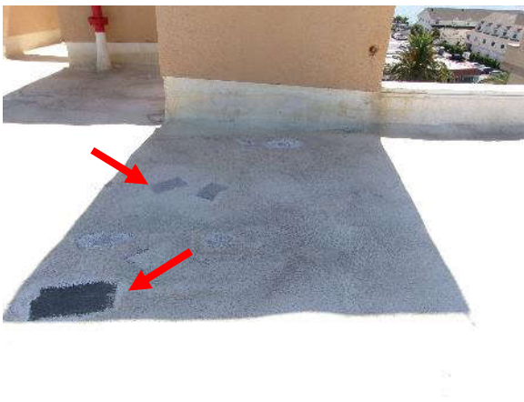
Photo 7.6.5 – Roof level – Repair patch in good condition.
