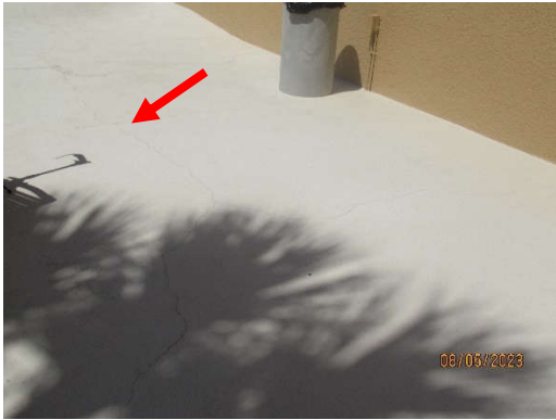
Photo 7.7.1 – Pool area - Concrete crack in the pool slab on grade.
