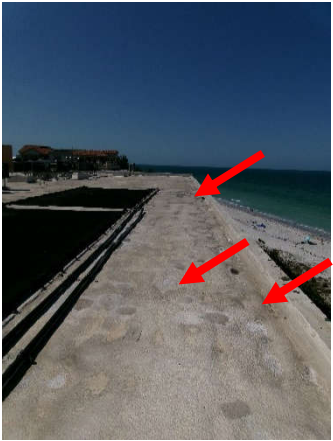
Photo 7.6.1 – Roof level – Uneven surface and evidence of temporary water ponding.
