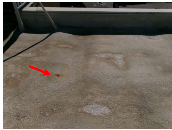
Photo 7.6.6 – Roof level – Rust spots observed.
