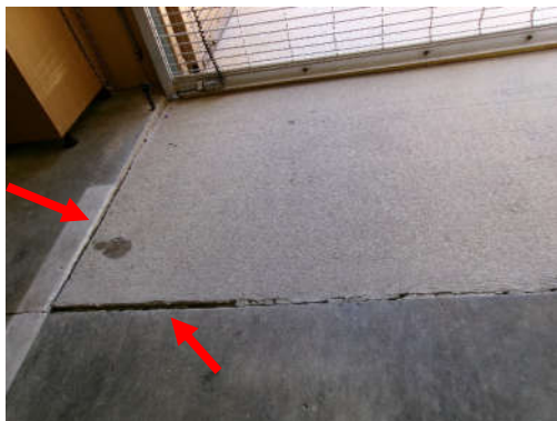
Photo 7.5.5 – Garage level isolation joint. In good to fair condition.
