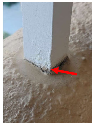
Photo 7.4.4 – Front corridor (East Façade) corrosion in the base of the railing.
