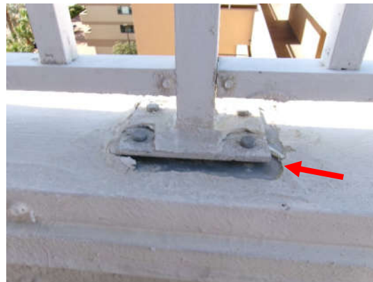
Photo 7.4.6 – Roof level - a vertical picket was observed with deflection, and vertical post anchors were loose.
