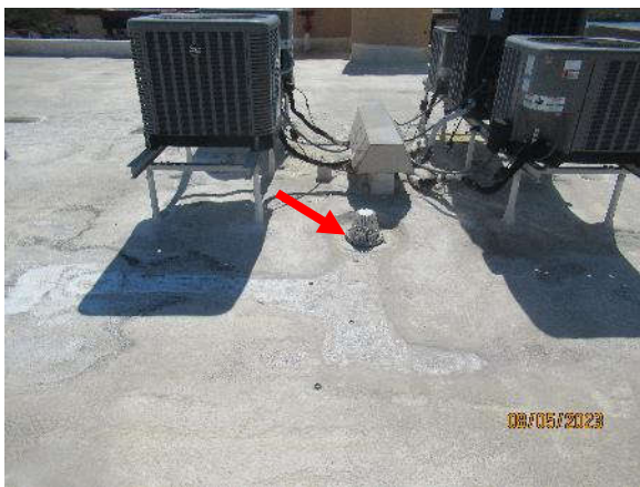
Photo 7.6.9 – Roof level – Roof drain dome gate loose.
