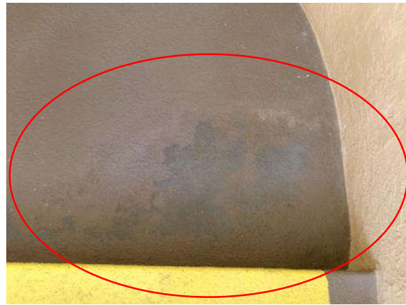
Photo 7.2.b.2 – Stairwell #1 – Evidence of ponding between the 3 rd and 2 nd levels.
