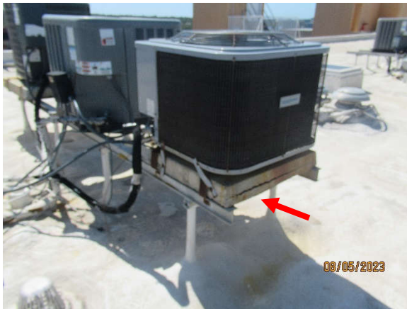
Photo 7.6.13 – Roof level – Rooftop equipment with corroded fastener and concrete base damaged.
