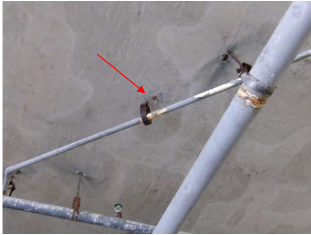
Photo 7.1.b.1 – Garage Level – Sprinkler system insert at the ceiling.
