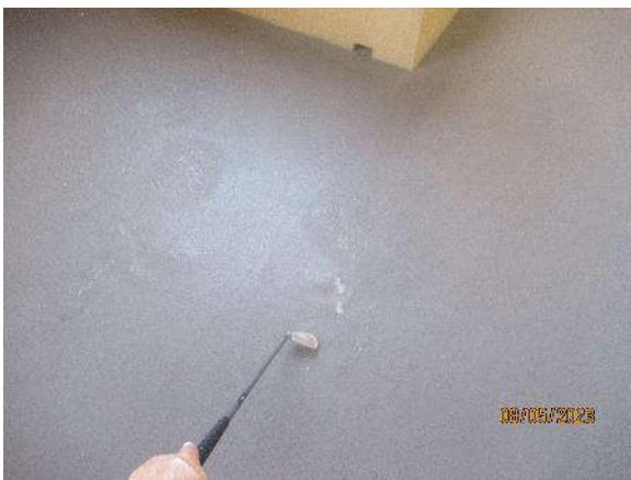
Photo 7.2.b.11 – Front corridor level 2 nd – De-bonding and peeling off the waterproofing membrane.
