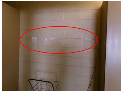
Photo 7.2.b.6 – Garage level – Evidence of efflorescence.
