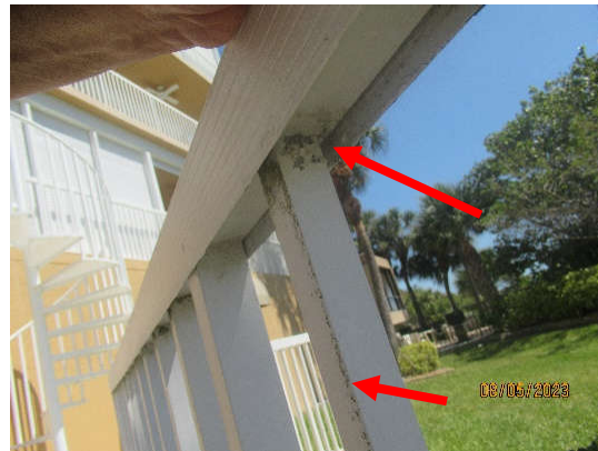
Photo 7.4.8 – Pool deck railing with paint weathered and mild corrosion.
