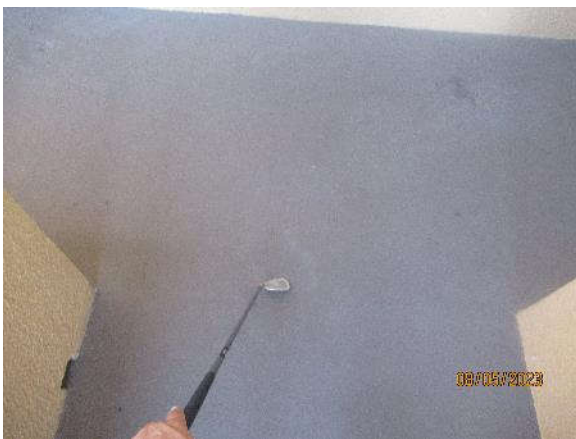
Photo 7.2.b.9 – Front corridor level 3 rd – De-bonding waterproofing membrane.
