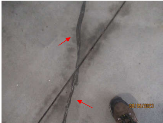
Photo 7.8.a.3 – Garage Level – Drying shrinkage cracks observed at the slab on grade. The application of cementitious material to repair and seal the crack was observed.
