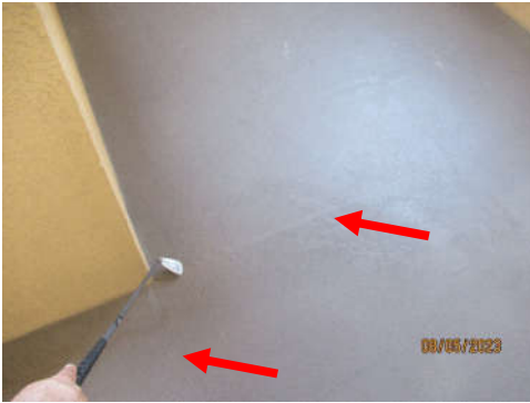
Photo 7.5.1 – Front corridor – Observed joint likely related to installing a cementitious topping or installing the waterproofing membrane. These joints were observed to be in good condition.
