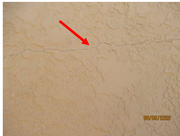
Photo 7.2.c.4 – Roof level stairwell #1 stucco horizontal crack.
