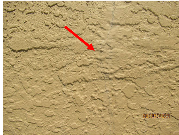
Photo 7.2.c.2 – West façade 1 st level stucco hairline crack.
