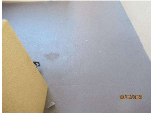
Photo 7.2.b.8 – Front corridor level 4 th – Delaminated waterproofing membrane.
