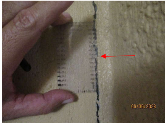
Photo 7.8.b.2 – Garage Level – Anticipated cracks in buildings and building materials typically result from restrained movement.
