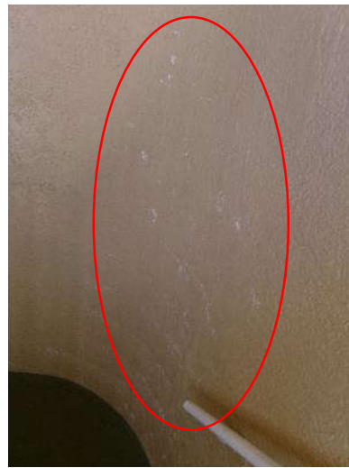
Photo 7.2.b.4 – Stairwell #1 – Evidence of efflorescence between the roof and the 4 th levels.
