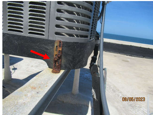
Photo 7.6.8 – Roof level – Rooftop equipment with corroded fasteners and steel angles.
