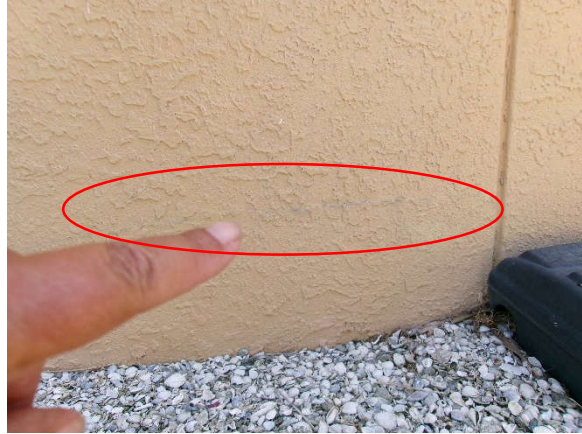
Photo 7.2.a.6 – North façade hairline cracks and evidence of efflorescence.
