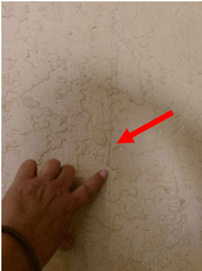
Photo 7.2.c.5 – Stairwell #2 stucco hairline crack.
