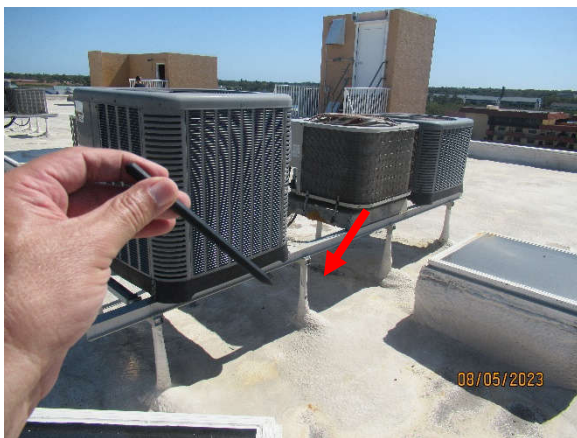
Photo 7.6.11 – Roof level – Peeled off the coating in the rooftop structure base.
