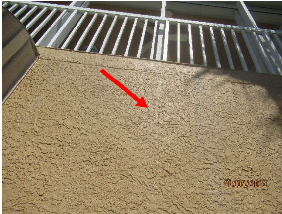
Photo 7.2.c.1 – West façade 1 st level repaired stucco crack.
