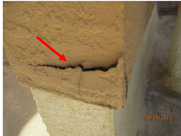
Photo 7.2.c.8 – Roof level vent shaft southeast corner – Stucco crack and de-bonded.
