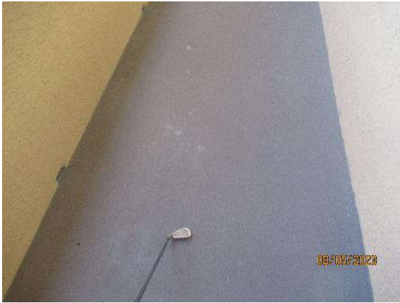
Photo 7.2.b.7 – Front corridor level 4 th – De-bonding waterproofing membrane.
