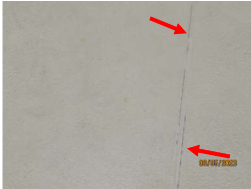
Photo 7.5.3 – Pool Deck - Visual assessment showed construction joint deficiencies such as cracks and de-bonding.
