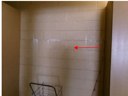
Photo 7.8.b.6 – Garage Level – Evidence of efflorescence was observed through some of the walls in the garage level.
