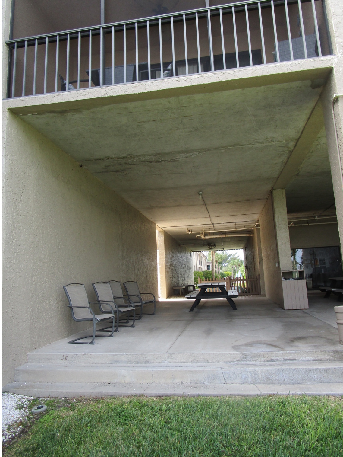
Precast concrete ceiling at ground level, Building 5. Minor concrete spalling observed.
