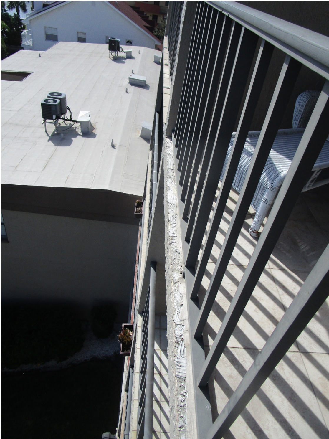
Balcony slab edge should be waterproofed to prevent corrosion deterioration of the concrete. Building 5, Unit 404.
