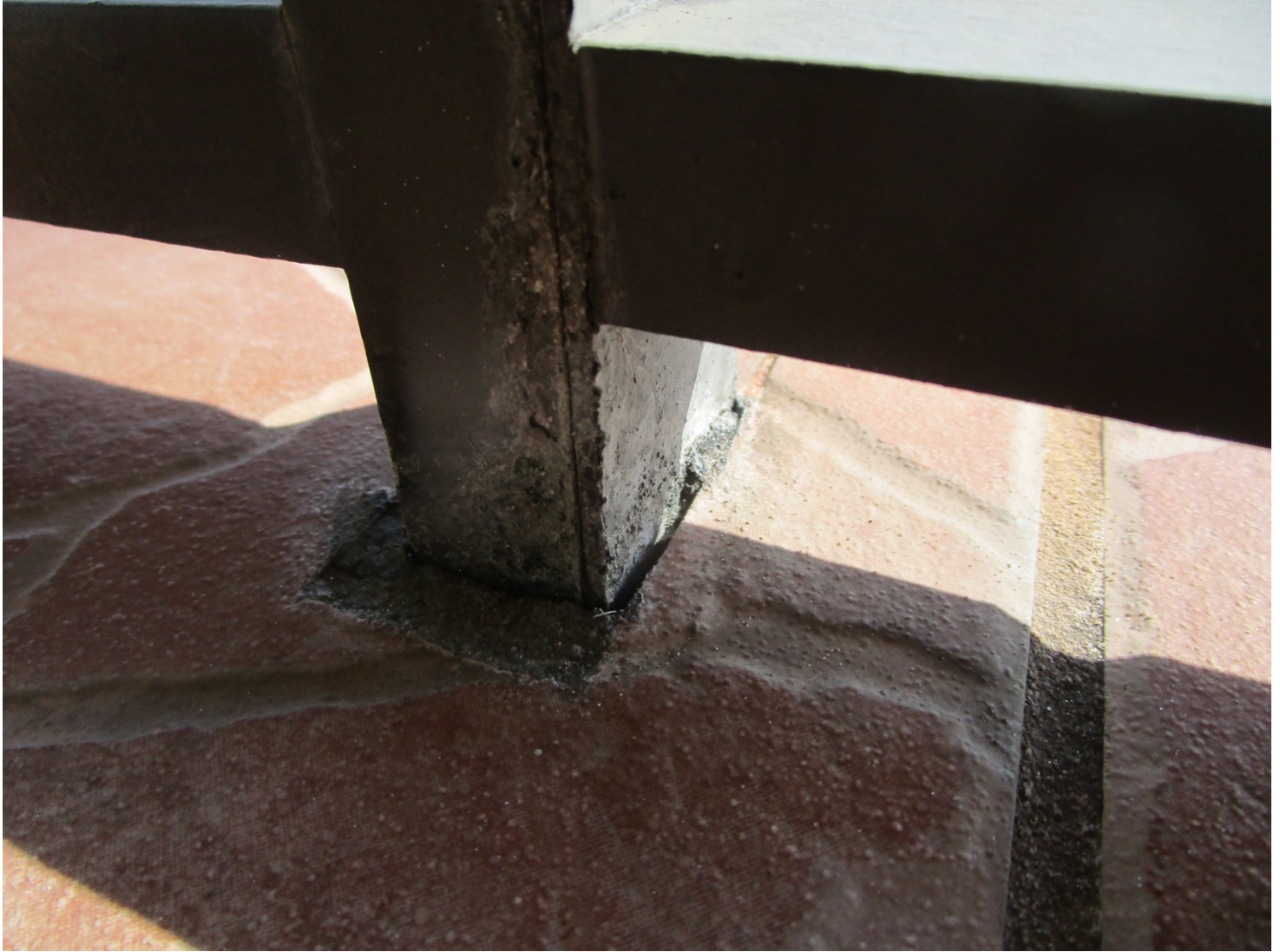
Typical “post pocket” requiring repair to re-anchor loose guardrail. Unit 502, Building 5.
