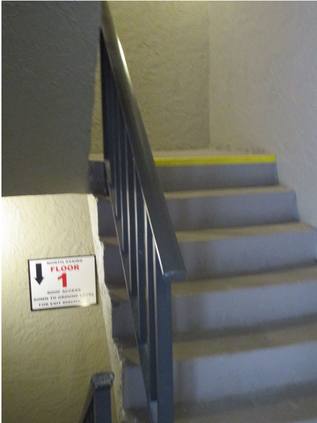
Loose handrail in stairwell. North stairwell of building 5, nearest to unit 101
