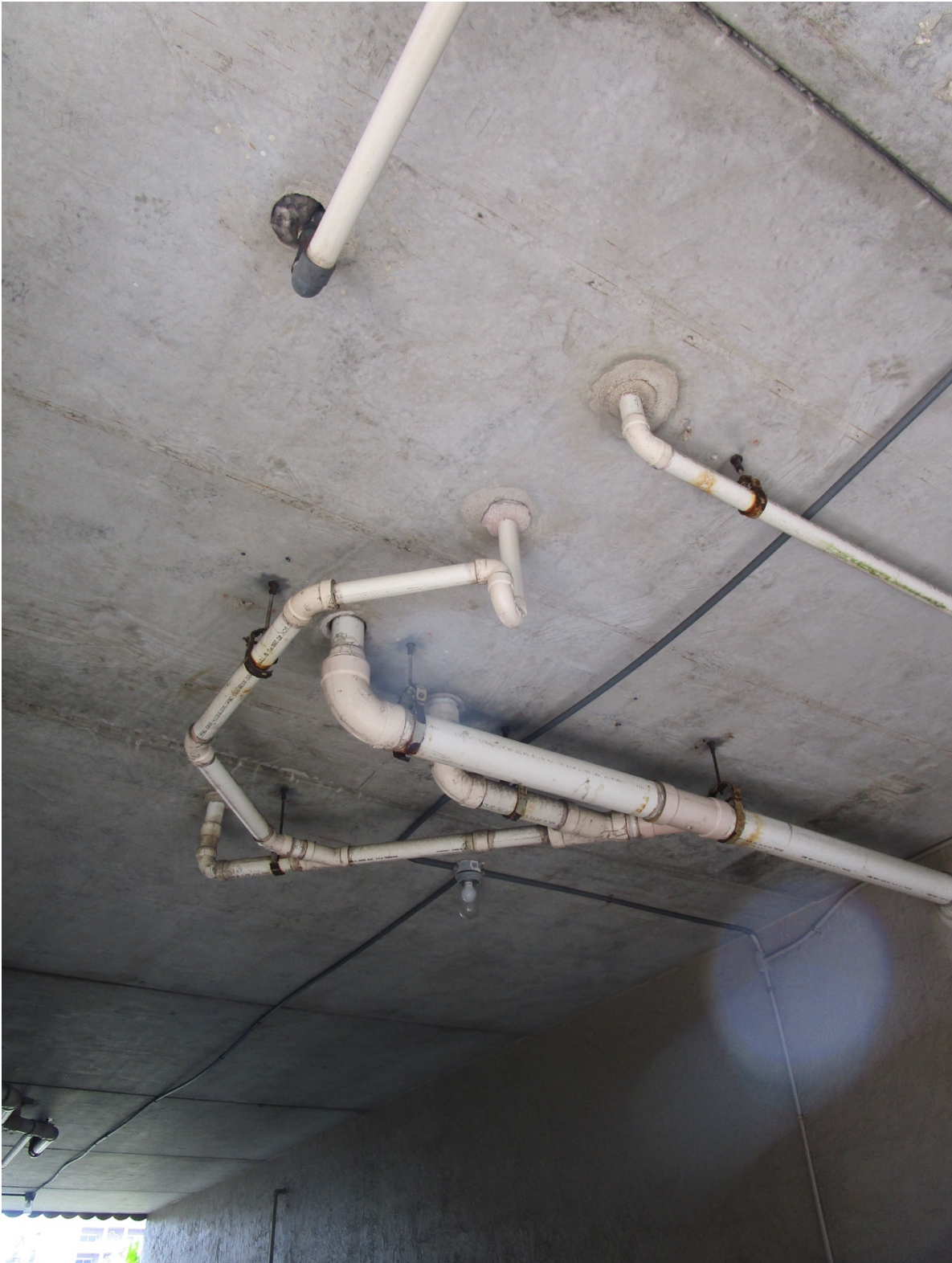
Support clamps around the pipes exhibit significant corrosion and many are broken. This is a typical condition on the ground floor ceiling of building 5.
