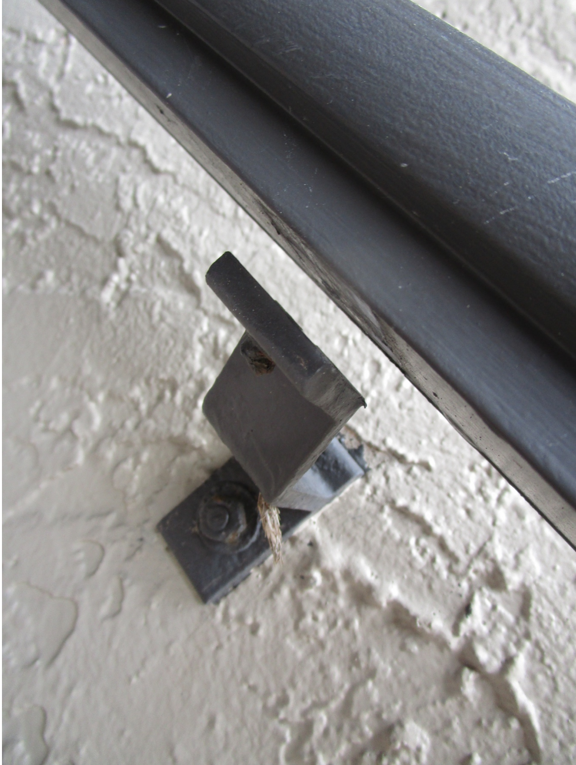
Building 8, Missing Fastener at Handrail
