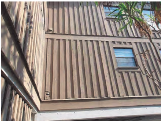
87 Wood Siding Peeling and Buckling
