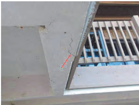
55 Rear Garage Beam Cracks
