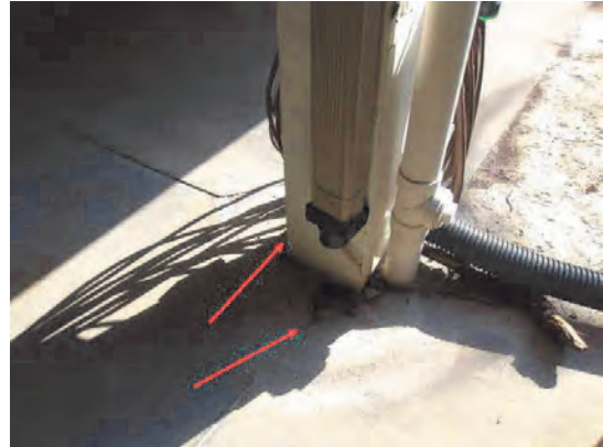
100 Left Front Gutter Downspout Discharge at Pier Footing
