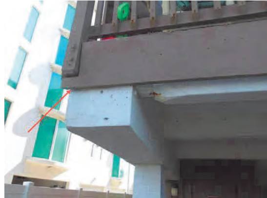
68 Right Rear Beam Cracking, Bulging and Rusting
