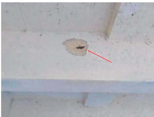
39 Right Middle Garage Cracking and exposed Re-Bar
