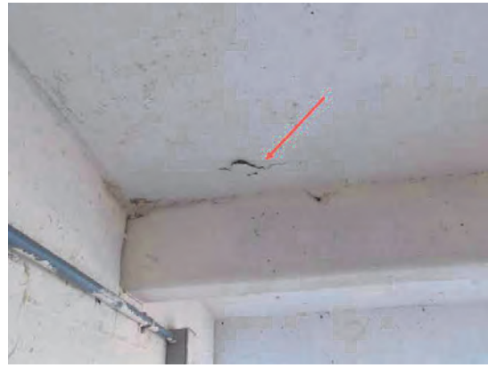
42 Right Rear Garage Cracking
