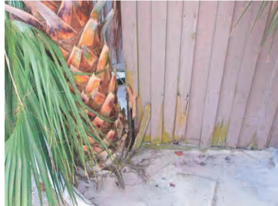
92 Wood Siding Peeling and Buckling
