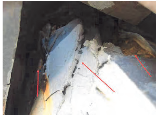
70 Right Rear Beam Cracking, Bulging and Rusting
