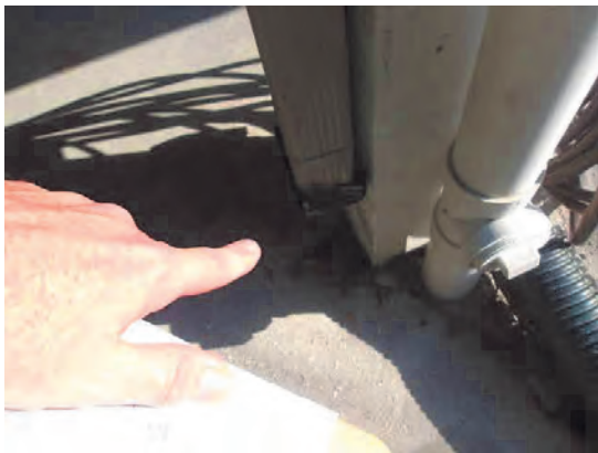
101 Left Front Gutter Downspout Discharge at Pier Footing
