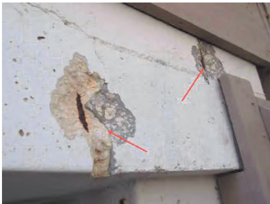
63 Right Front Garage Exposed Re-Bar
