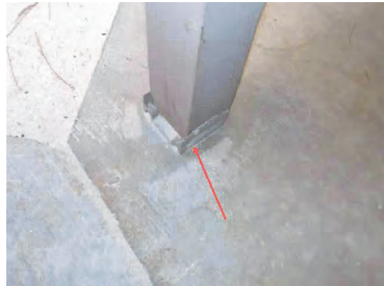
110 Left Front Stairs 4x4 Posts Not Secured to Slab
