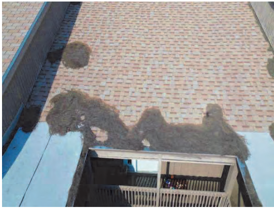
113 Clogged Gutters and Debris on Roof
