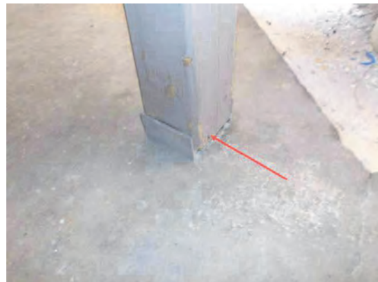
112 Left Front Stairs 4x4 Posts Not Secured to Slab
