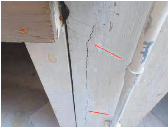
57 Left Side Garage Pier Cracks
