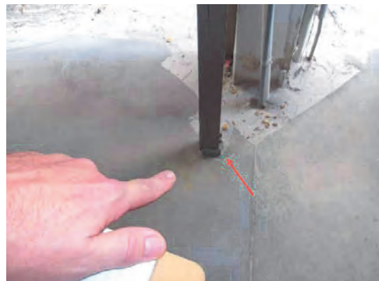
104 Right Front Stairs 4x4 Posts Not Secured to Slab
