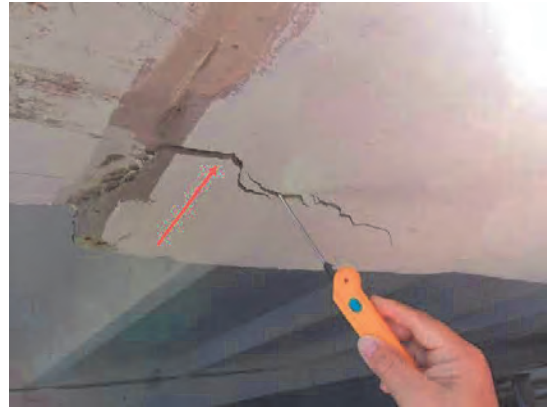
36 Damage to Left Rear Garage Beam From Flood Wall
