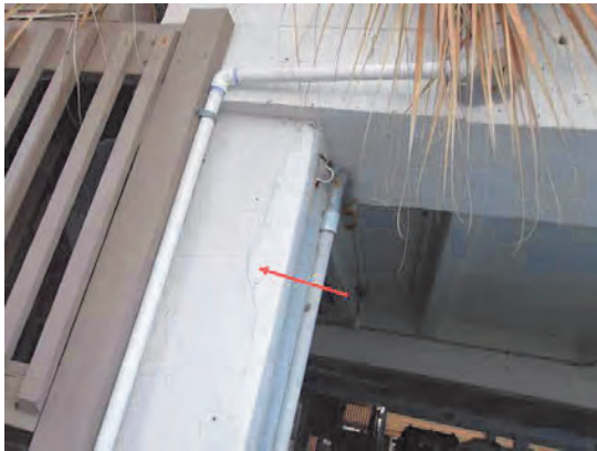
61 Right Side Garage Pier Cracks
