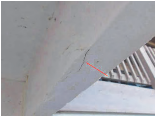
53 Rear Garage Beam Cracks
