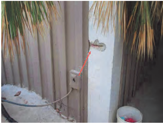
65 Right Front Garage Exposed Re-Bar
