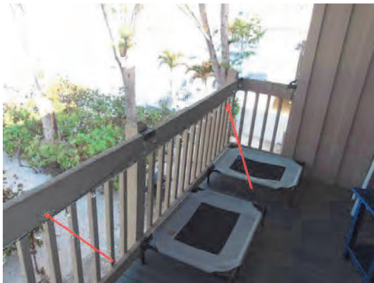
71 Loose Handrail Unit 6
