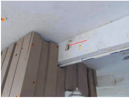
41 Right Rear Garage Cracking and exposed Re-Bar
