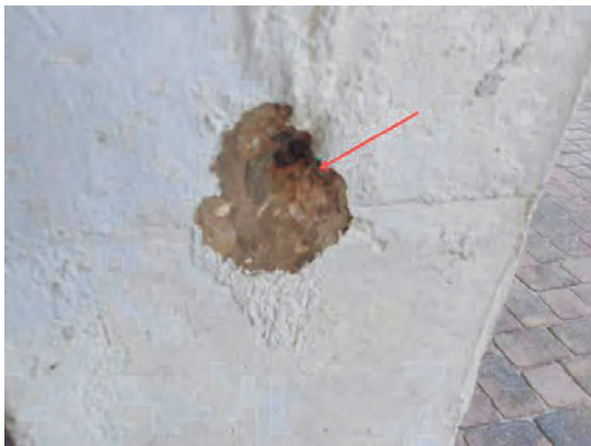
47 Rear Garage Pier Cracks and Exposed Re-Bar
