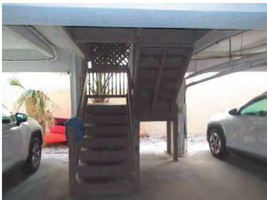
103 Right Front Stairs 4x4 Posts Not Secured to Slab
