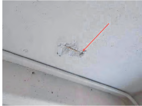
60 Left Side Garage Exposed Re-Bar
