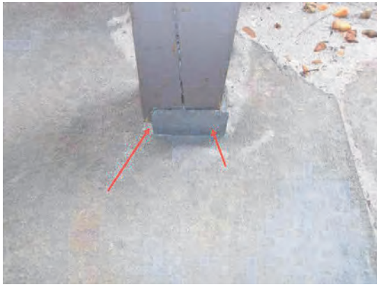
105 Right Front Stairs 4x4 Posts Not Secured to Slab
