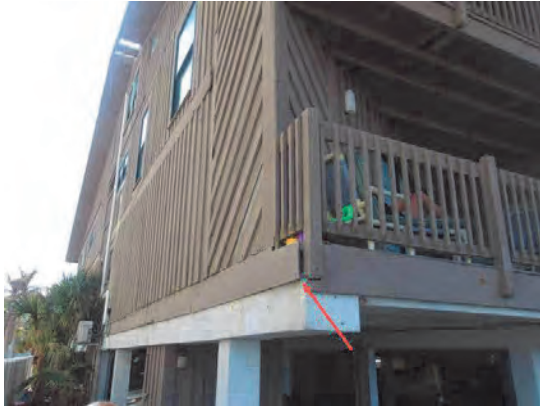
67 Right Rear Beam Cracking, Bulging and Rusting
