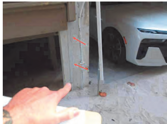
56 Left Side Garage Pier Cracks
