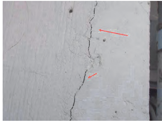
58 Left Side Garage Pier Cracks
