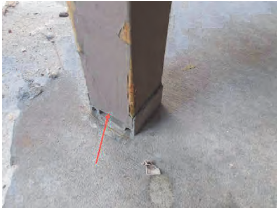
107 Right Front Stairs 4x4 Posts Not Secured to Slab
