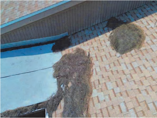
116 Clogged Gutters and Debris on Roof
