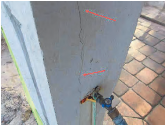
49 Rear Garage Pier Cracks
