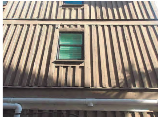
86 Wood Siding Peeling and Buckling
