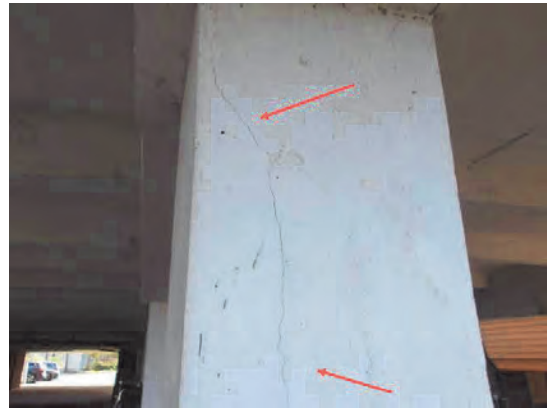
50 Rear Garage Pier Cracks
