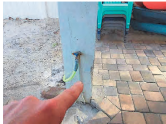
48 Rear Garage Pier Cracks
