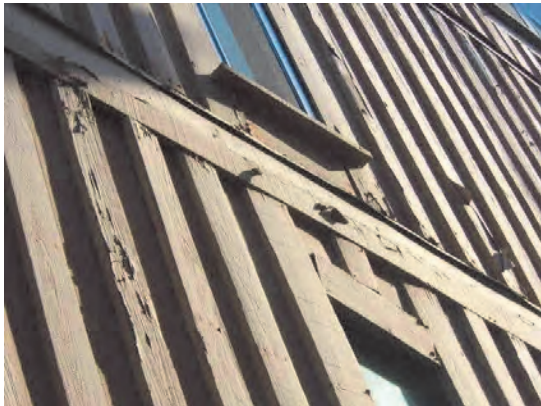
85 Wood Siding Peeling and Buckling
