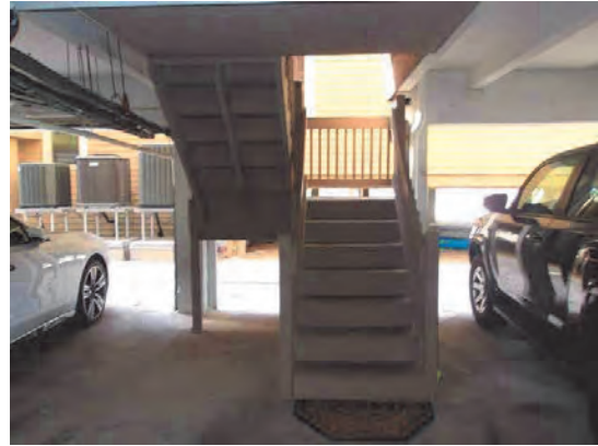
108 Left Front Stairs 4x4 Posts Not Secured to Slab
