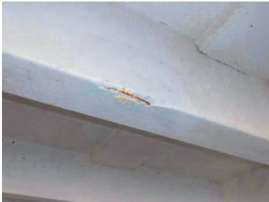
45 Left Rear Garage Cracking and exposed Re-Bar
