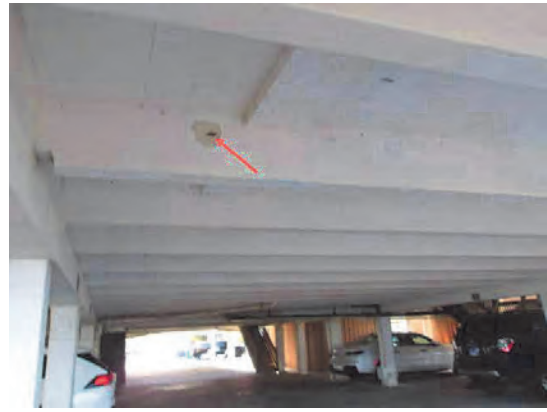
34 Right Middle Garage Cracking and exposed Re-Bar
