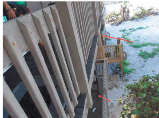
72 Loose Handrail Unit 6
