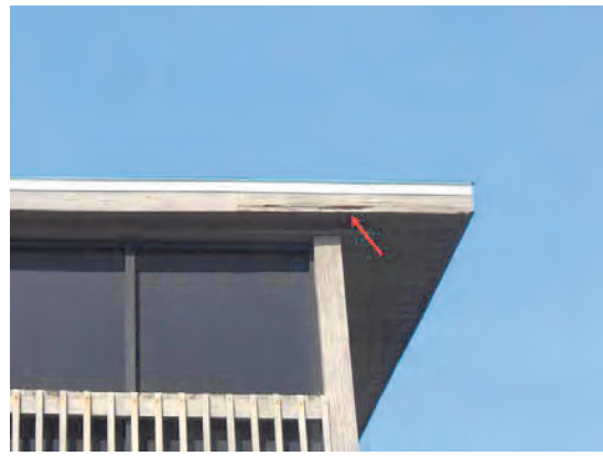
82 Right Front Facia Deterioration
