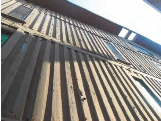
83 Wood Siding Peeling and Buckling
