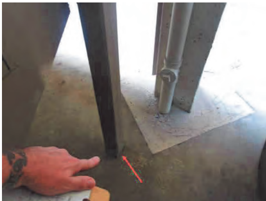
111 Left Front Stairs 4x4 Posts Not Secured to Slab
