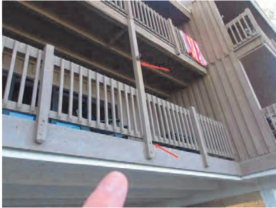
75 Loose and Cracked Handrail Unit 3
