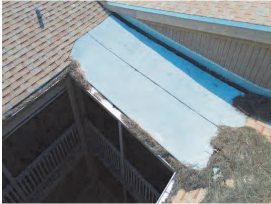
115 Clogged Gutters and Debris on Roof
