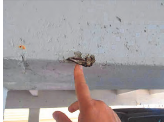
52 Middle Garage exposed re-Bar
