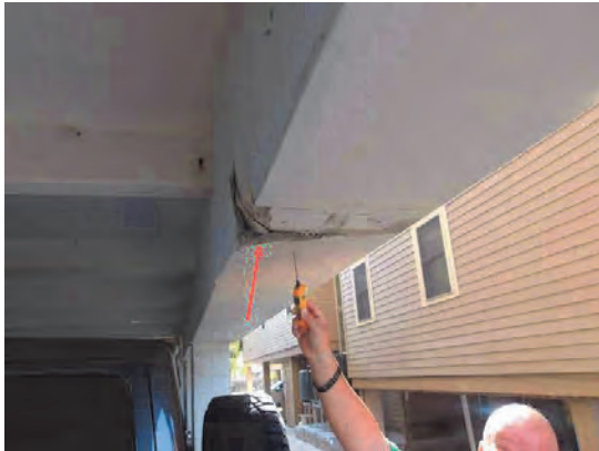
35 Damage to Left Rear Garage Beam From Flood Wall
