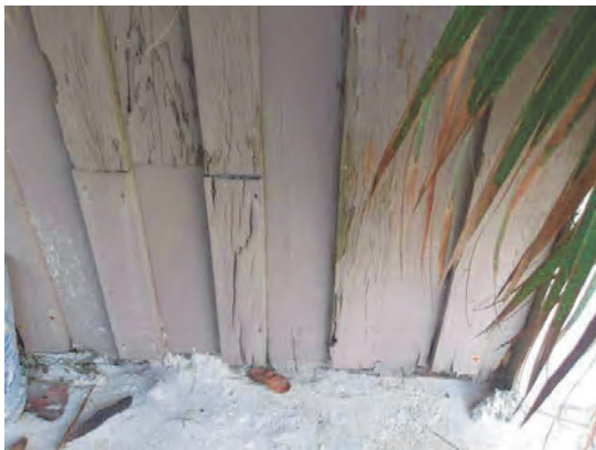
95 Wood Siding Deterioration
