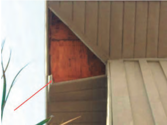
99 Right Front Soffit Damage
