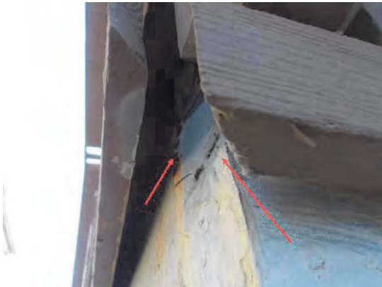
69 Right Rear Beam Cracking, Bulging and Rusting
