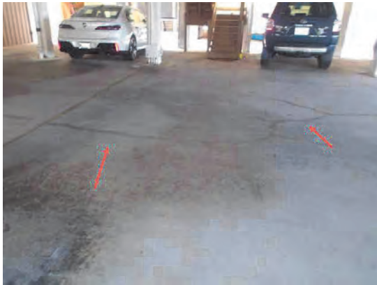
77 Garage Slab Cracks
