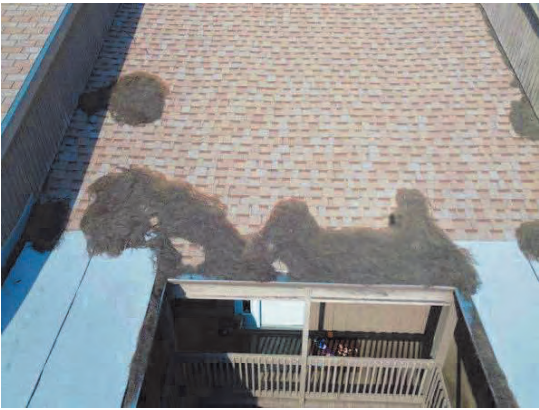
114 Clogged Gutters and Debris on Roof
