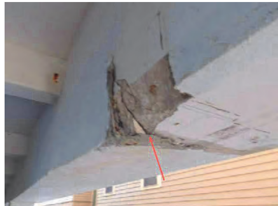
38 Damage to Left Rear Garage Beam From Flood Wall
