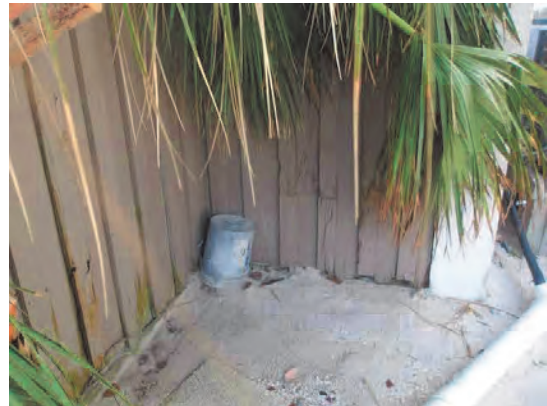
94 Wood Siding Deterioration
