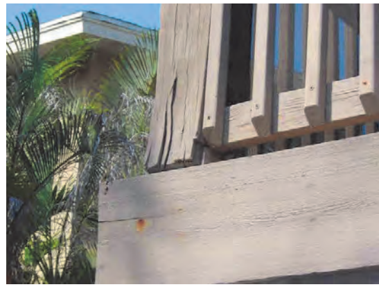
90 Wood Trim Peeling and Buckling
