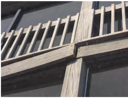
89 Wood Trim Peeling and Buckling
