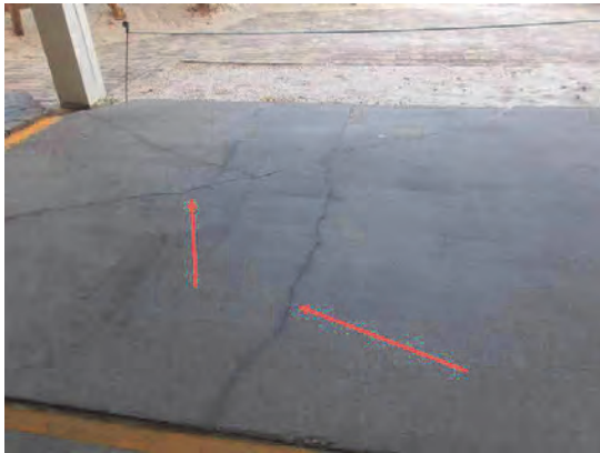
79 Garage Slab Cracks
