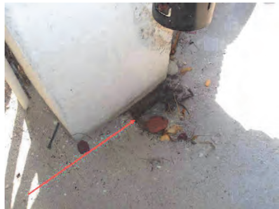
102 Left Front Gutter Downspout Discharge at Pier Footing
