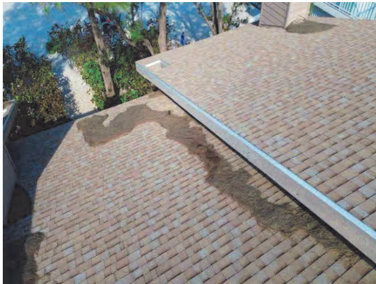
117 Clogged Gutters and Debris on Roof
