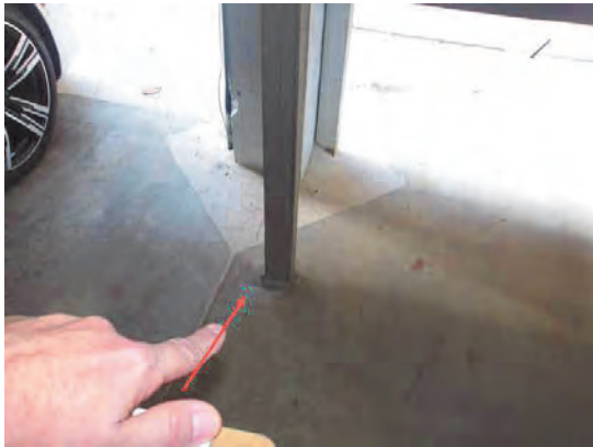
109 Left Front Stairs 4x4 Posts Not Secured to Slab
