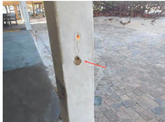
46 Rear Garage Pier Cracks and Exposed Re-Bar
