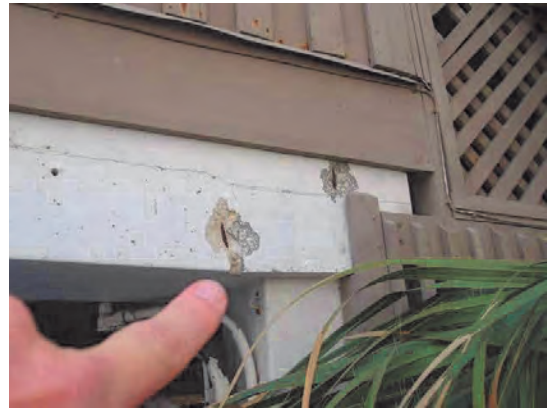
62 Right Front Garage Exposed Re-Bar
