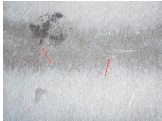
78 Garage Slab Cracks
