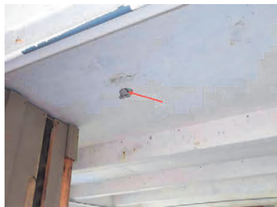
40 Right Rear Garage Cracking and exposed Re-Bar
