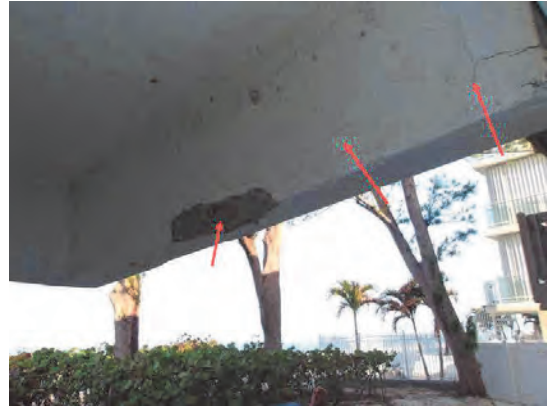
44 Left Rear Garage Cracking and exposed Re-Bar
