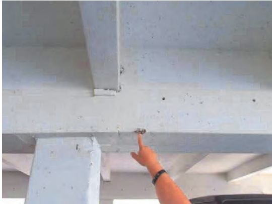
51 Middle Garage exposed re-Bar
