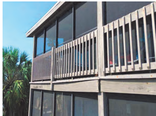
88 Wood Trim Peeling and Buckling
