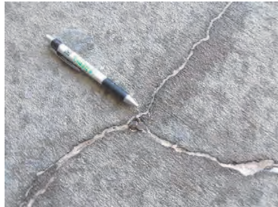
80 Garage Slab Cracks
