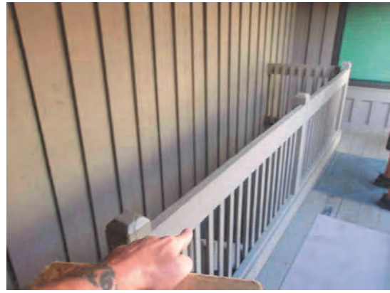
74 Loose Handrail Unit 5
