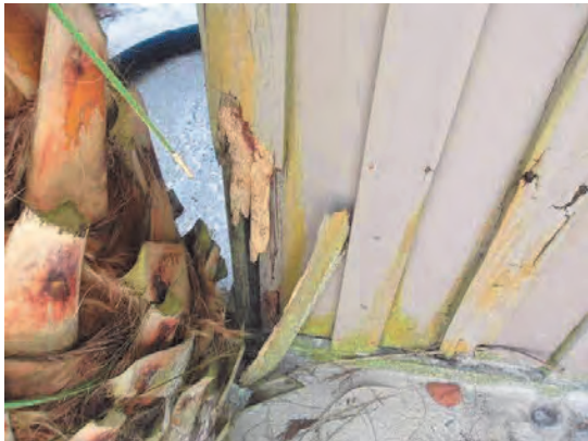
93 Wood Siding Deterioration
