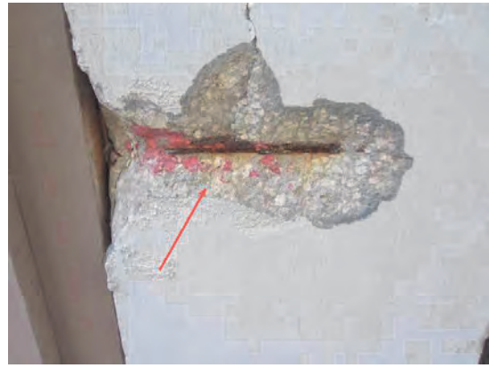
66 Right Front Garage Exposed Re-Bar
