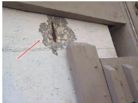
64 Right Front Garage Exposed Re-Bar
