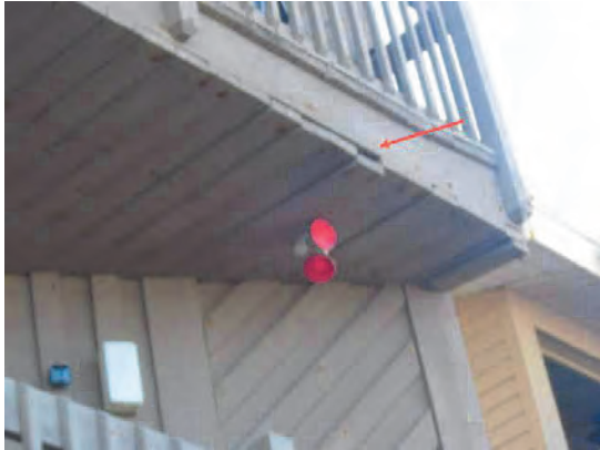
91 Rear Soffit Buckling
