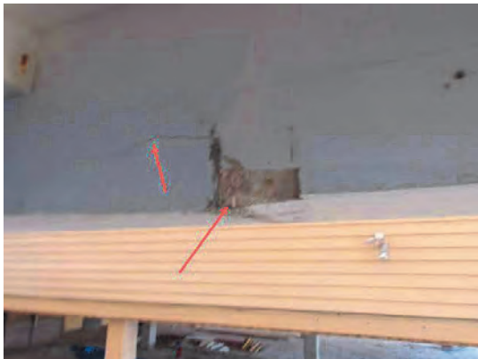
37 Damage to Left Rear Garage Beam From Flood Wall
