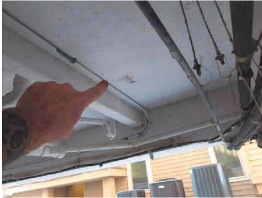
59 Left Side Garage Exposed Re-Bar
