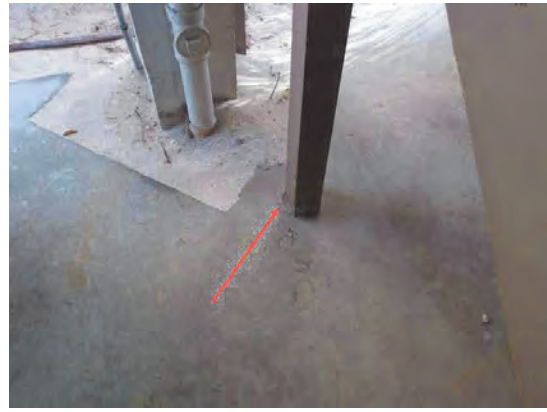
106 Right Front Stairs 4x4 Posts Not Secured to Slab
