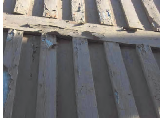
84 Wood Siding Peeling and Buckling
