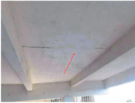
33 Rear Garage Ceiling Cracks Repairs
