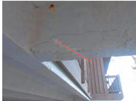
54 Rear Garage Beam Cracks
