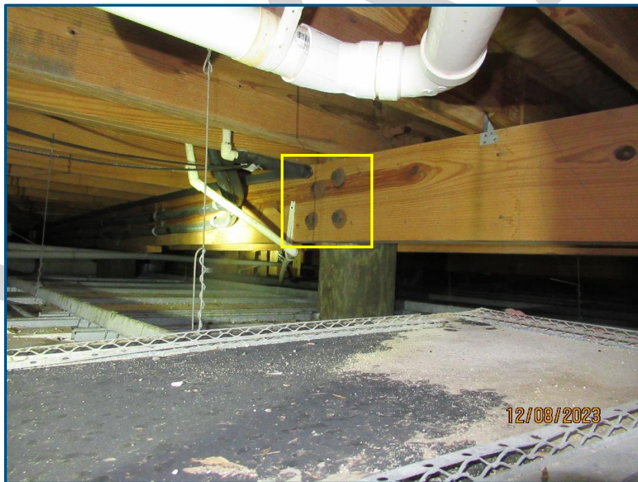
Photograph No. 26: View of corroded bolts in the wood beam to column connection located in the attic space above the parking area.
