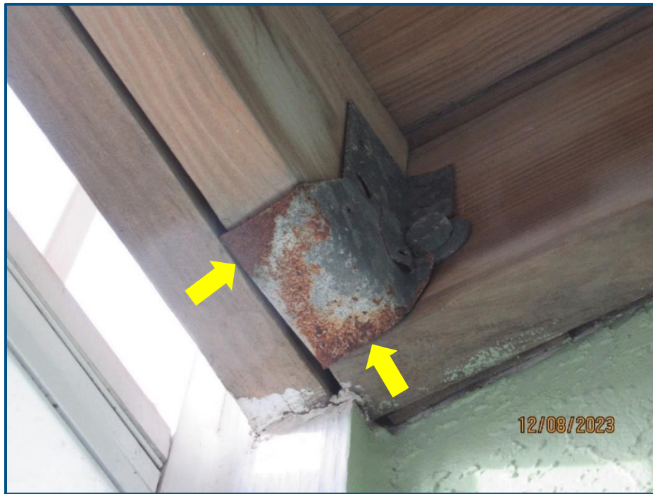
Photograph No. 15: View of corroded metal hanger beneath the stair landing on the east elevation.
