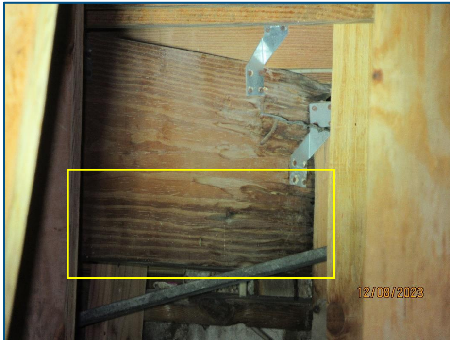
Photograph No. 25: View of moisture damage in the wood beam located in the attic space above the parking area (same beam shown in Photograph No. 14).
