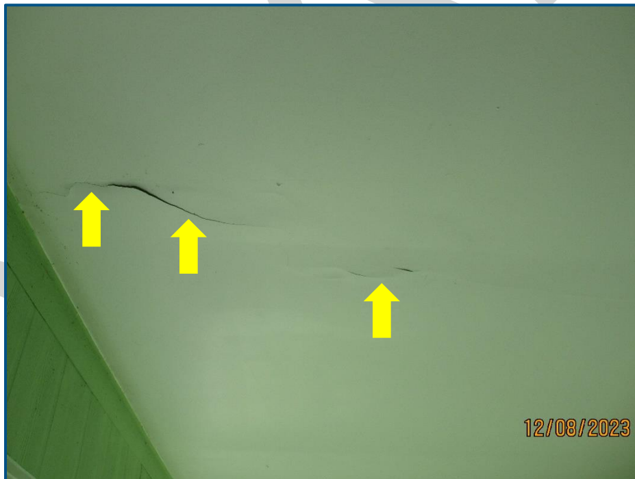
Photograph No. 18: View of paint delamination in the ceiling of the 3 rd floor landing area on the east elevation.
