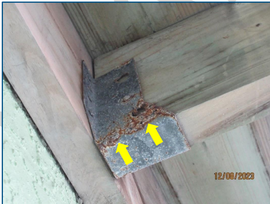
Photograph No. 20: View of a corroded metal hanger beneath the 3 rd floor landing on the west elevation.
