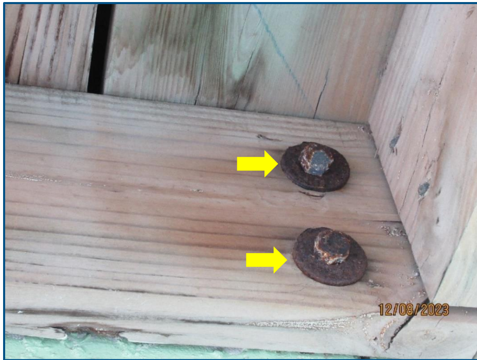
Photograph No. 21: View of corroded bolts under the 3 rd floor landing on the west elevation.
