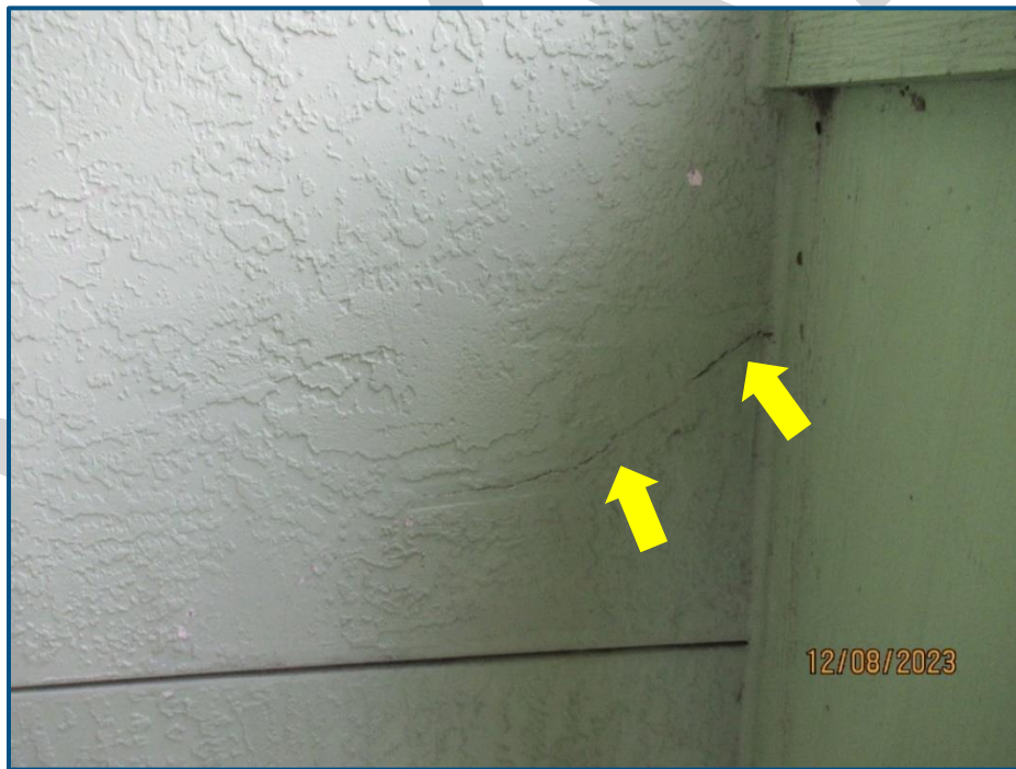
Photograph No. 22: View of a crack in the exterior stucco finish on the west elevation.
