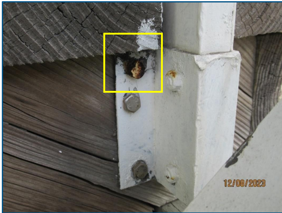
Photograph No. 17: View of a corroded fastener in a metal handrail located on the 2 nd floor stairs on the east elevation.
