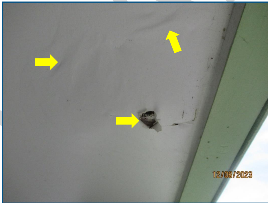
Photograph No. 10: View of bubbling paint and damage to the drywall ceiling located in the parking area.
