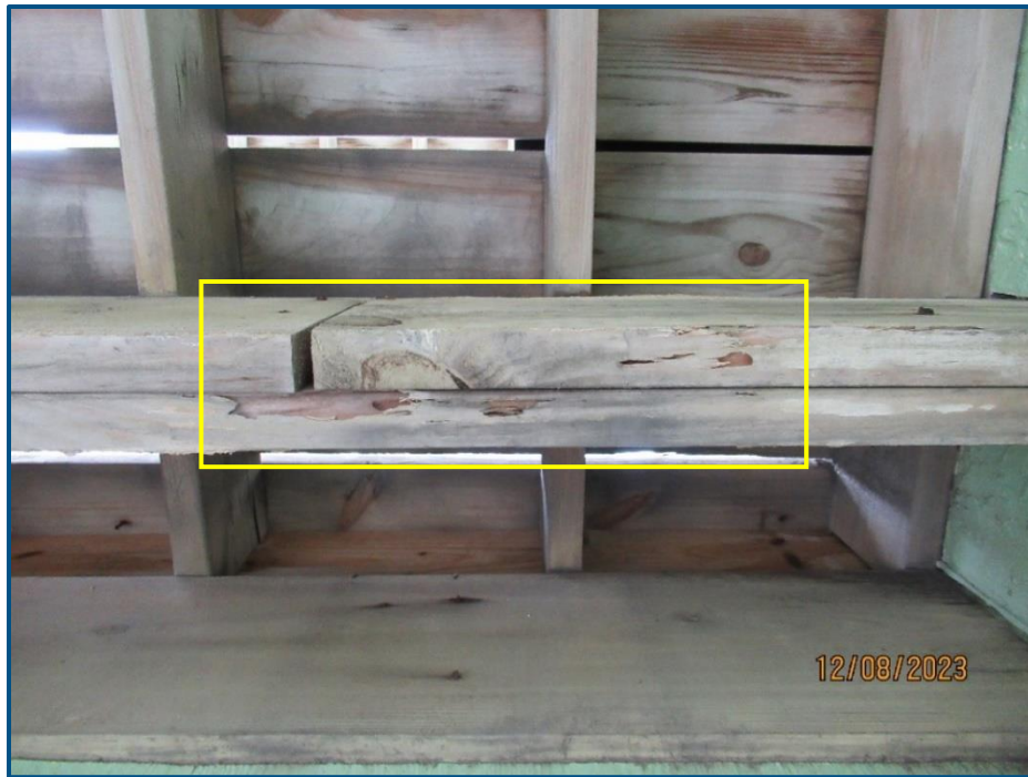
Photograph No. 19: View of termite damage in a wood beam located under the 2 nd floor landing on the west elevation.
