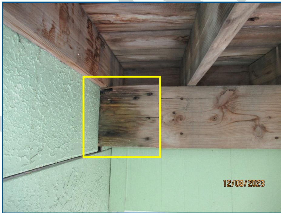
Photograph No. 14: View of moisture damage to a wood beam located below the 2 nd floor stair landing on the east elevation.
