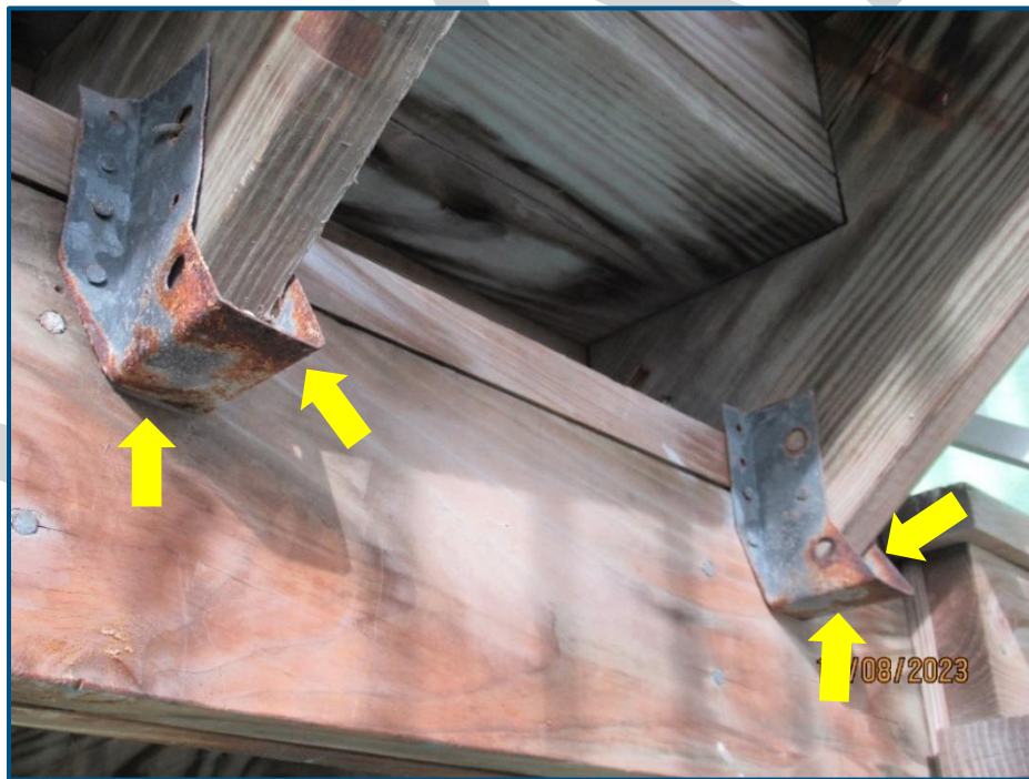
Photograph No. 16: View of corroded metal hangers under the stairs on the east elevation.
