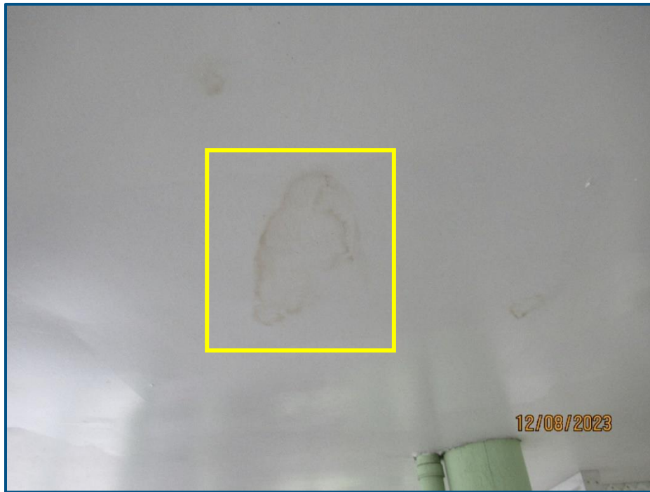
Photograph No. 9: View of a moisture stain in the drywall ceiling located in the parking area.
