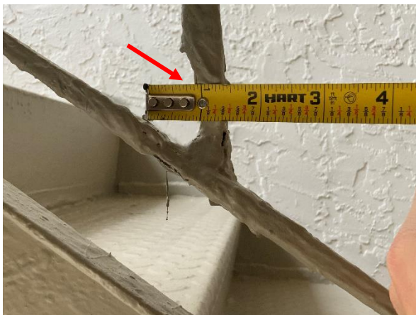
Photo 27 East Building - North Elevation – 2 nd Floor - Overall view of corroded staircase baluster.
