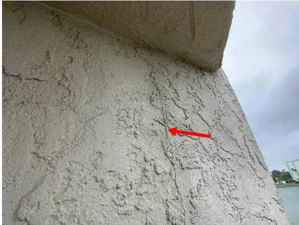
Photo 43 East Building – Unit 303 – Overall view of cracking cement plaster.
