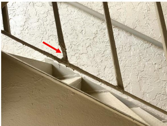
Photo 26 East Building - North Elevation – 2 nd Floor - Overall view of corroded staircase baluster.
