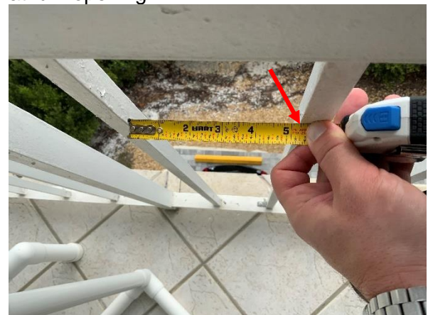
Photo 18 East Building – Unit 301 - Overall view of the guard rail picket spacing over 4 inches.
