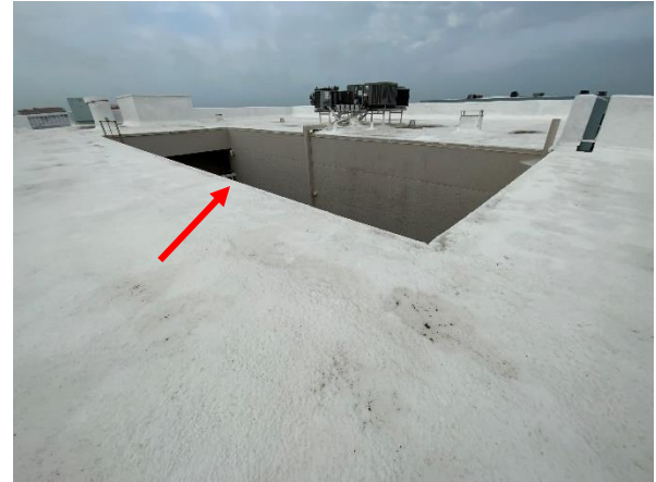
Photo 16 East Building - West Elevation – Roof - Overall view of no guard rails installed at the atrium opening.
