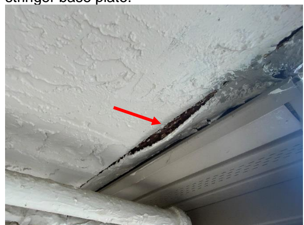
Photo 24 East Building - North Elevation – 1 st Floor - Overall view of corrosion at the staircase landing.
