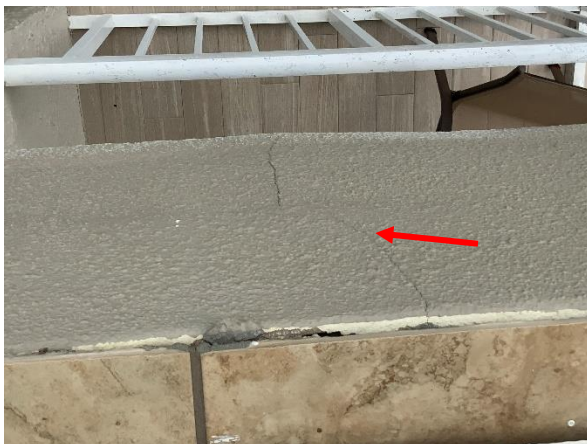
Photo 39 West Building – Unit 402 – Overall view of cracking cement plaster.
