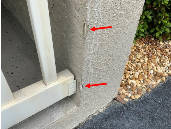
Photo 37 West Building – West Elevation – Ground Floor - Overall view of damaged cement plaster.
