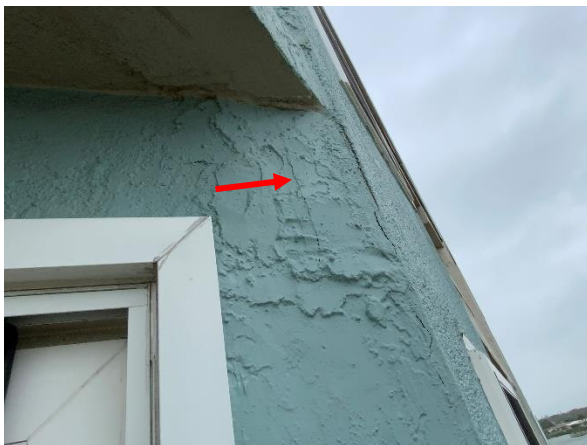
Photo 44 East Building – Unit 305 – Overall view of cracking cement plaster.
