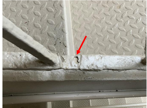
Photo 22 West Building - South Elevation – 2 nd Floor - Overall view of corroded staircase base rail.
