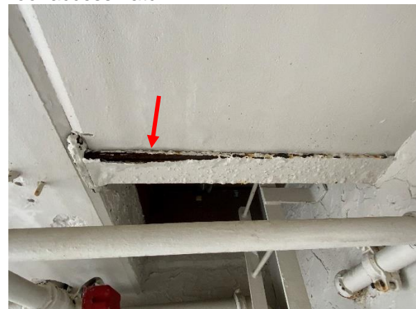
Photo 30 West Building - North Elevation – 5 th Floor - Overall view of corroded metal framing at the roof access hatch.
