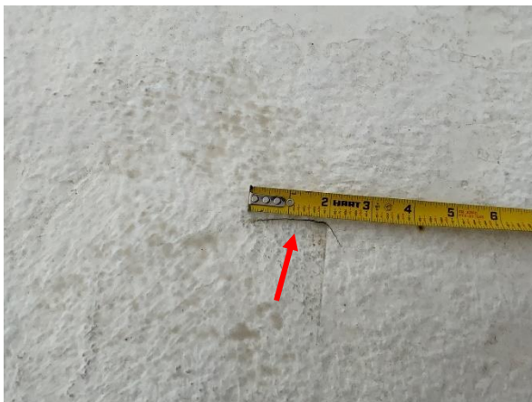
Photo 33 East Building - Roof – Overall view of punctures in the roof coating.
