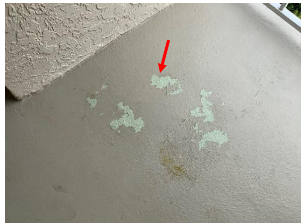
Photo 54 East Building – 4 th Floor – Overall view of delaminated walkway traffic coating.
