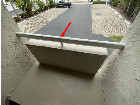
Photo 13 West Building - West Elevation – 1 st Floor - Overall view of loose-fitting guard rail.
