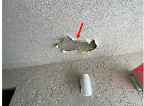
Photo 52 East Building – Unit 301 – Overall view of delaminated exterior coating.
