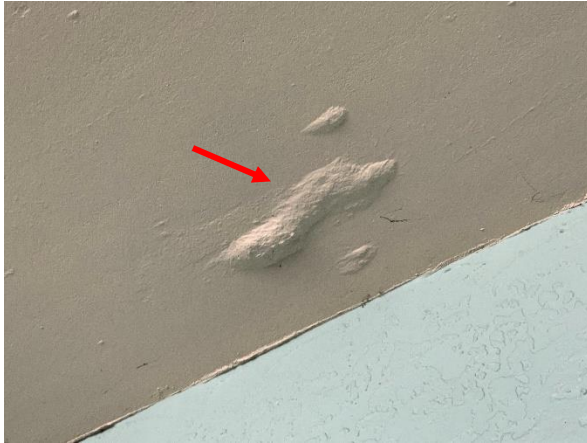
Photo 49 East Building – Ground Parking – Overall view of delaminated exterior coating.
