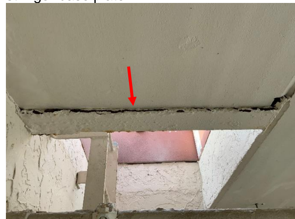
Photo 29 West Building - South Elevation – 5 th Floor - Overall view of corroded metal framing at the roof access hatch.
