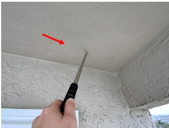
Photo 51 East Building – Unit 301 – Overall view of delaminated exterior coating.
