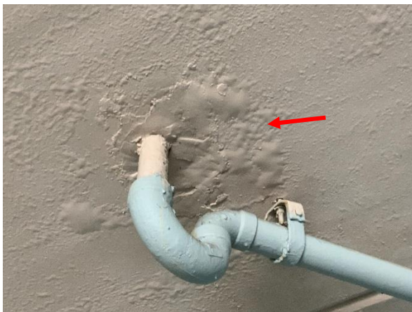
Photo 50 East Building – Ground Parking – Overall view of delaminated exterior coating.
