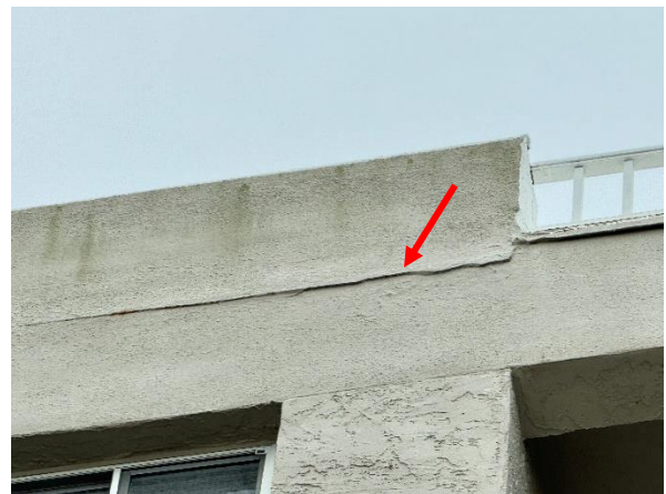
Photo 35 West Building – North Elevation – Roof - Overall view of cracking cement plaster.
