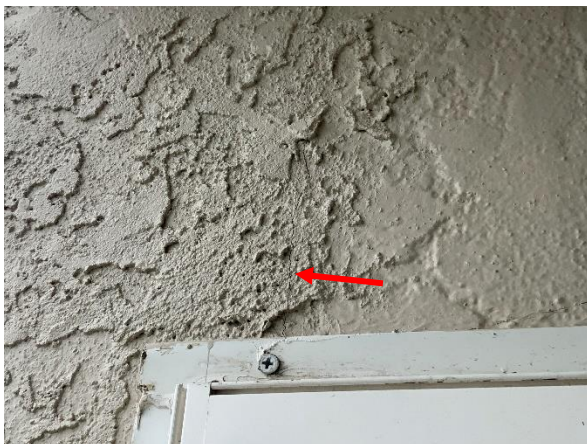
Photo 45 East Building – Unit 401 – Overall view of cracking cement plaster.
