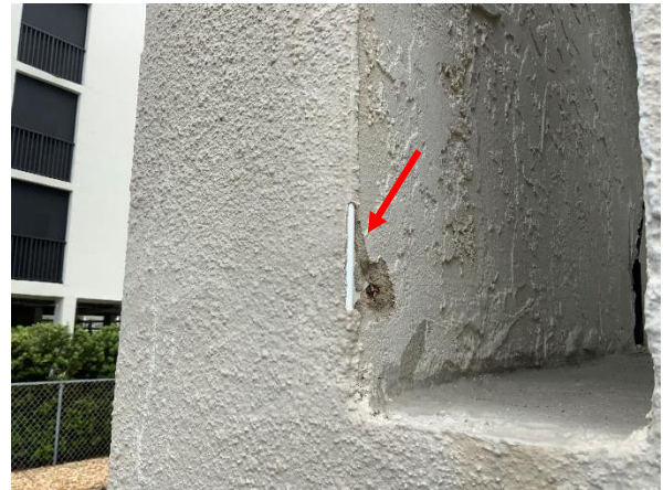
Photo 36 West Building – West Elevation – Ground Floor - Overall view of damaged cement plaster.
