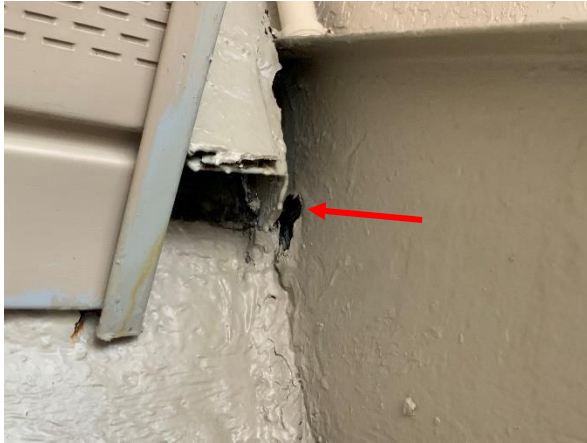
Photo 25 East Building - North Elevation – 1 st Floor - Overall view of corroded staircase stringer.
