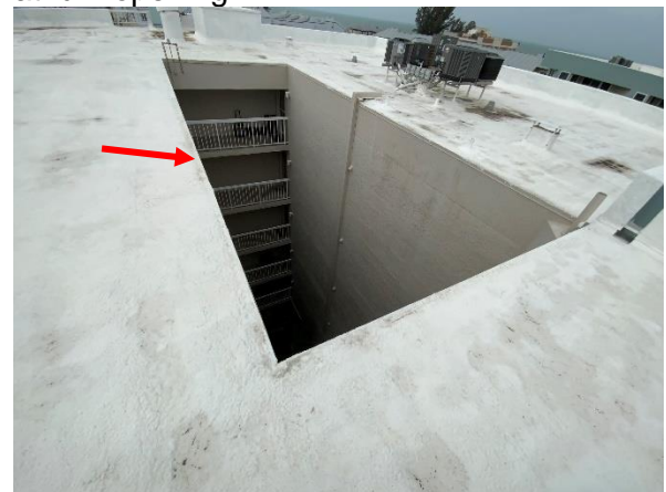
Photo 17 East Building - West Elevation – Roof - Overall view of no guard rails installed at the atrium opening.
