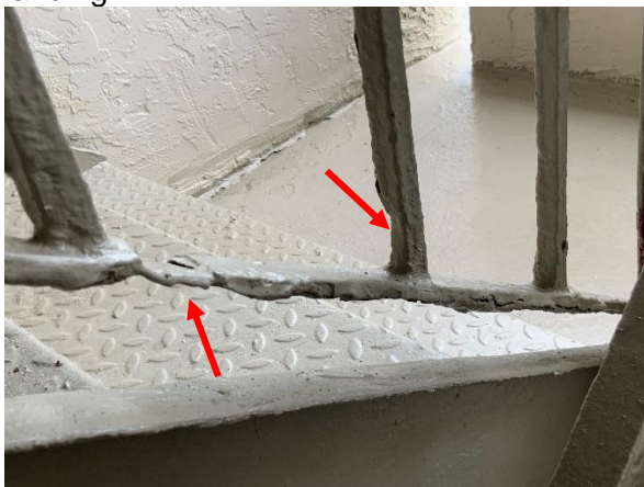
Photo 21 West Building - South Elevation – 2 nd Floor - Overall view of corroded staircase base rail and baluster.
