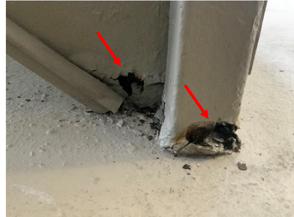
Photo 28 East Building - South Elevation – Ground Floor - Overall view of corroded staircase stringer base plate.
