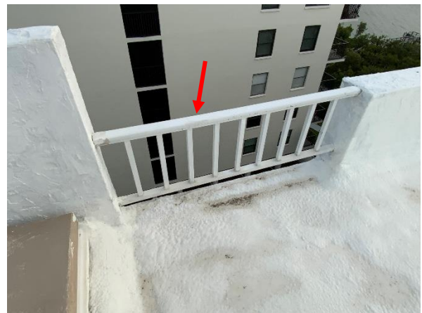
Photo 11 West Building - North Elevation – Roof - Overall view of loose-fitting guard rail.
