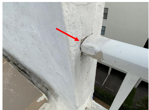
Photo 12 West Building - North Elevation – Roof - Overall view of loose-fitting guard rail.
