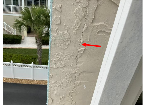
Photo 40 West Building – Unit 306 – Overall view of cracking cement plaster.
