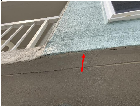
Photo 38 West Building – East Elevation – 1 st Floor - Overall view of cracking cement plaster.
