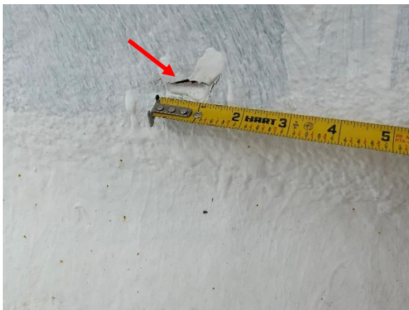
Photo 32 West Building - Roof – Overall view of punctures in the roof coating.
