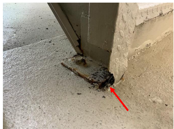
Photo 23 West Building - South Elevation – Ground Floor - Overall view of corroded staircase stringer base plate.
