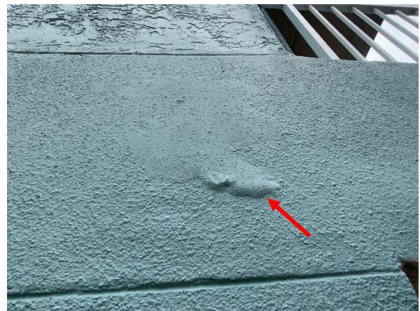
Photo 48 East Building – South Elevation – 1 st Floor – Overall view of delaminated exterior coating.
