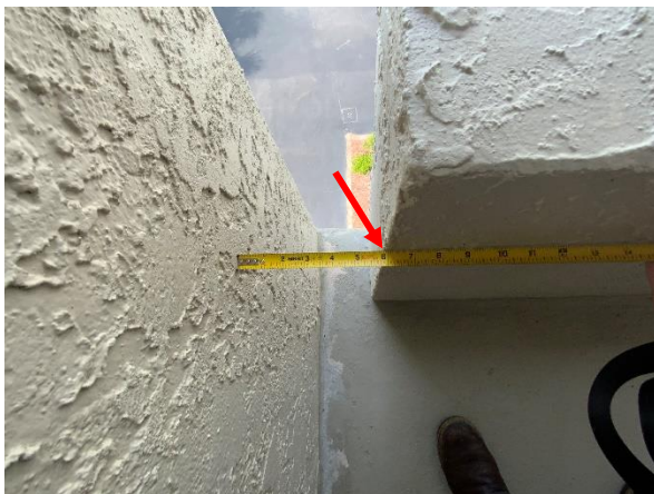
Photo 15 East Building - South Elevation – 4 th Floor - Overall view of the stair well landing parapet wall spacing over 4 inches.
