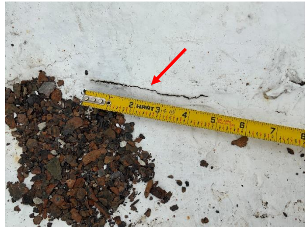
Photo 34 East Building - Roof – Overall view of punctures in the roof coating.
