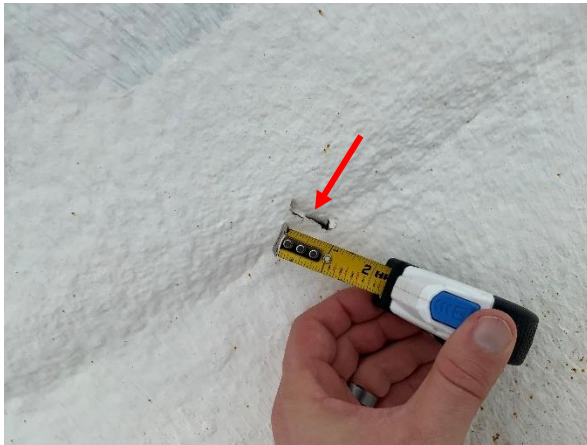
Photo 31 West Building - Roof – Overall view of punctures in the roof coating.
