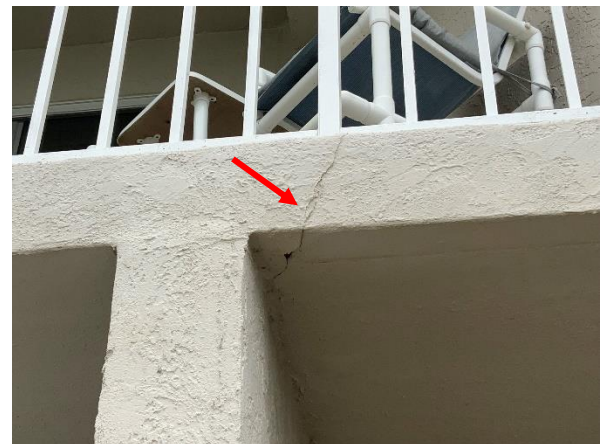
Photo 42 East Building – East Elevation – 1 st Floor - Overall view of cracking cement plaster.
