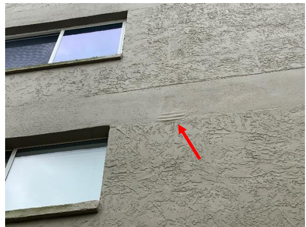
Photo 47 West Building – North Elevation – 2 nd Floor – Overall view of delaminated exterior coating.
