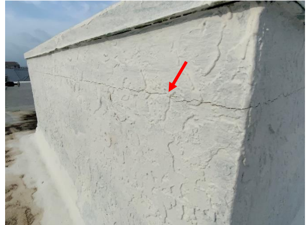
Photo 46 East Building – Roof – Overall view of cracking cement plaster.
