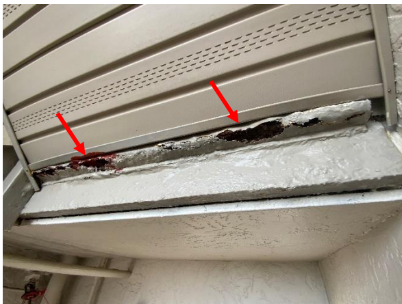
Photo 20 West Building - North Elevation – 3 rd Floor - Overall view of corrosion at the staircase landing.
