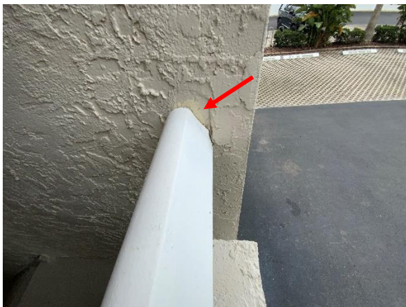
Photo 14 West Building - West Elevation – 1 st Floor - Overall view of loose-fitting guard rail.
