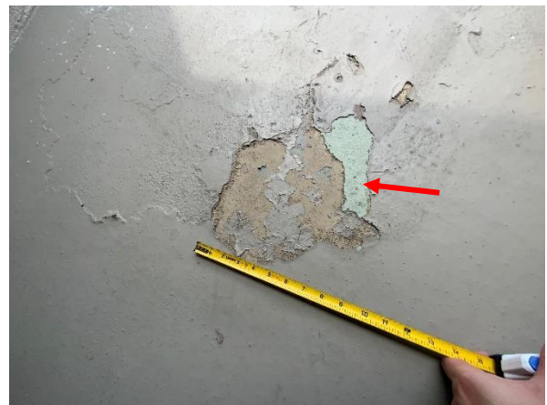
Photo 53 West Building – 1 st Floor – Overall view of delaminated walkway traffic coating.
