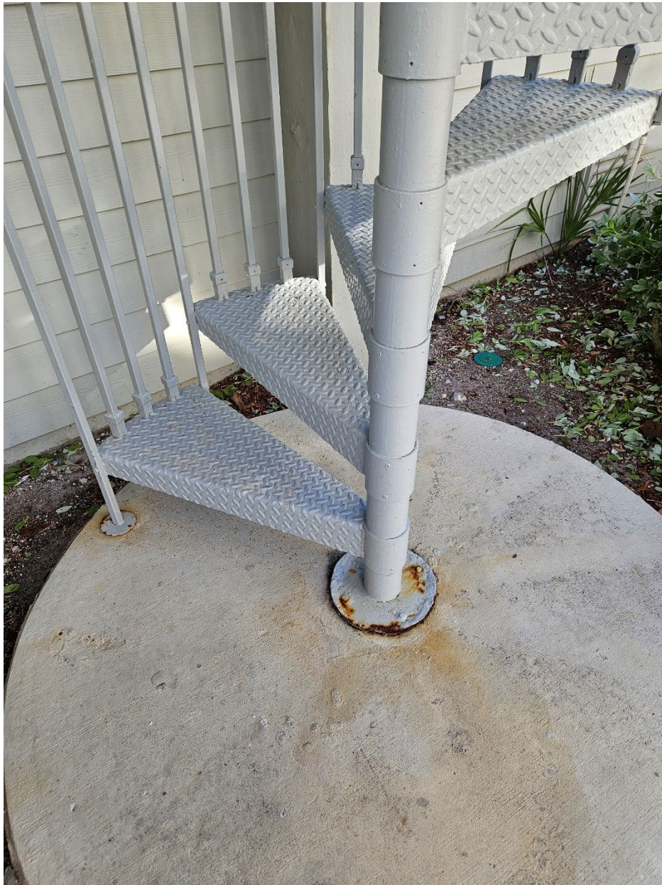
SPIRAL STAIR BASE PLATE DETERIORATION - COMMON AT ALL BUILDINGS
