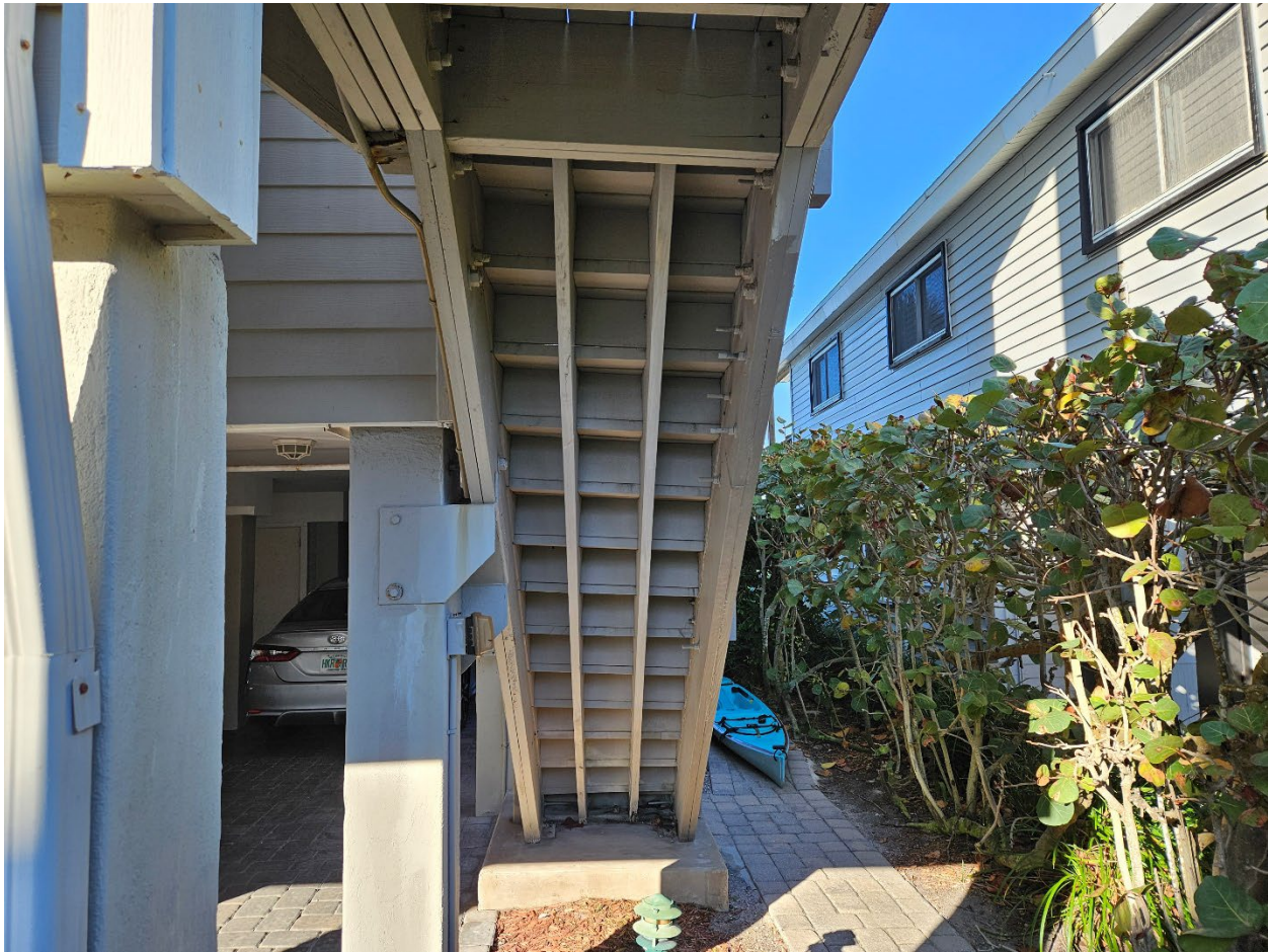
DEFLECTED STAIR FRAMING RUN
