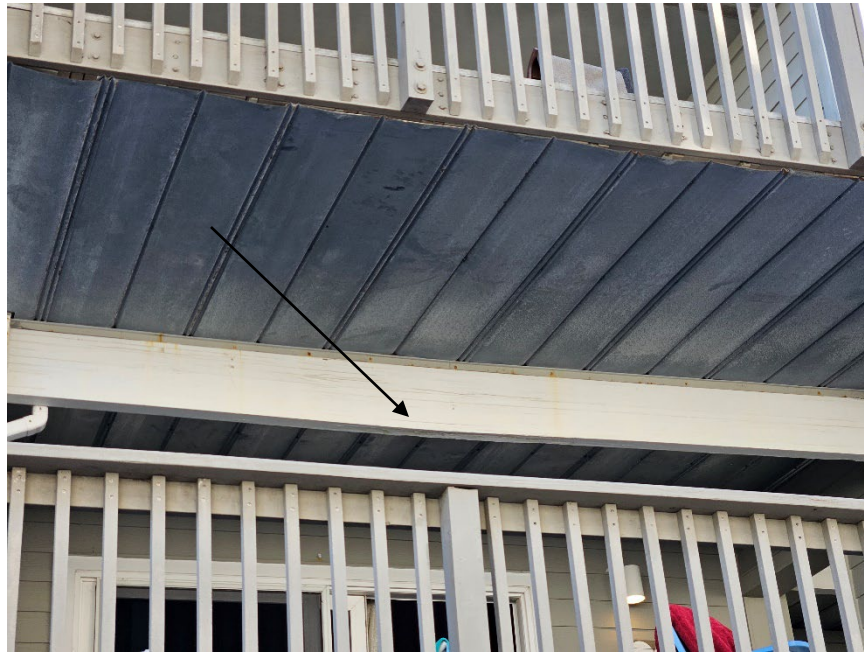
METAL SHEET PANS INSTALLED UNDER 3 RD FL FRAMING 2" DEFLECTION NOTED IN BEAM
