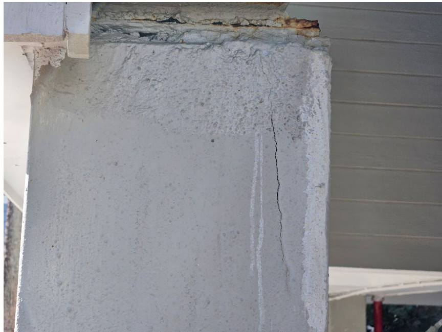
NE COLUMN DELAMINATION AND PLATE DAMAGE
