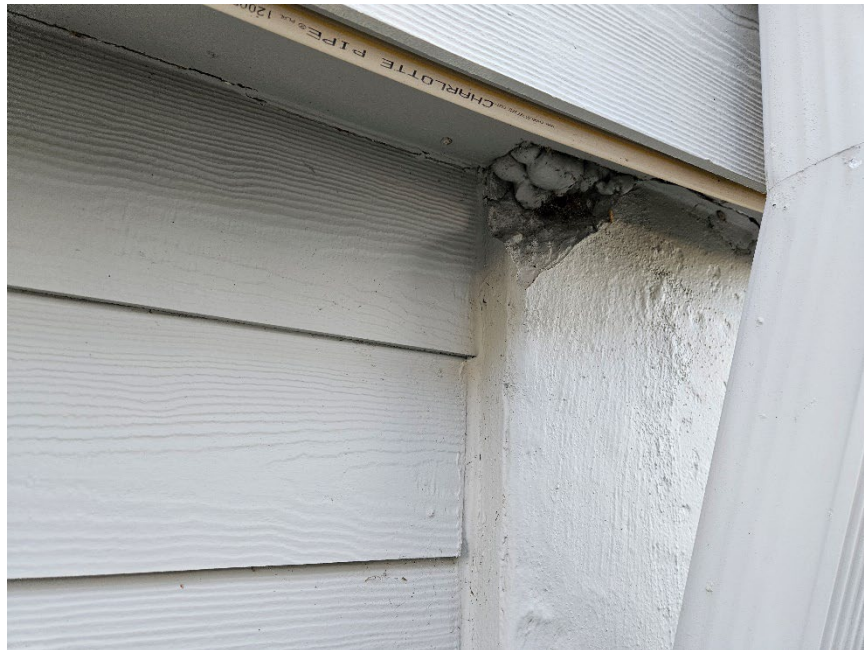
DAMAGED COLUMN CORNER
