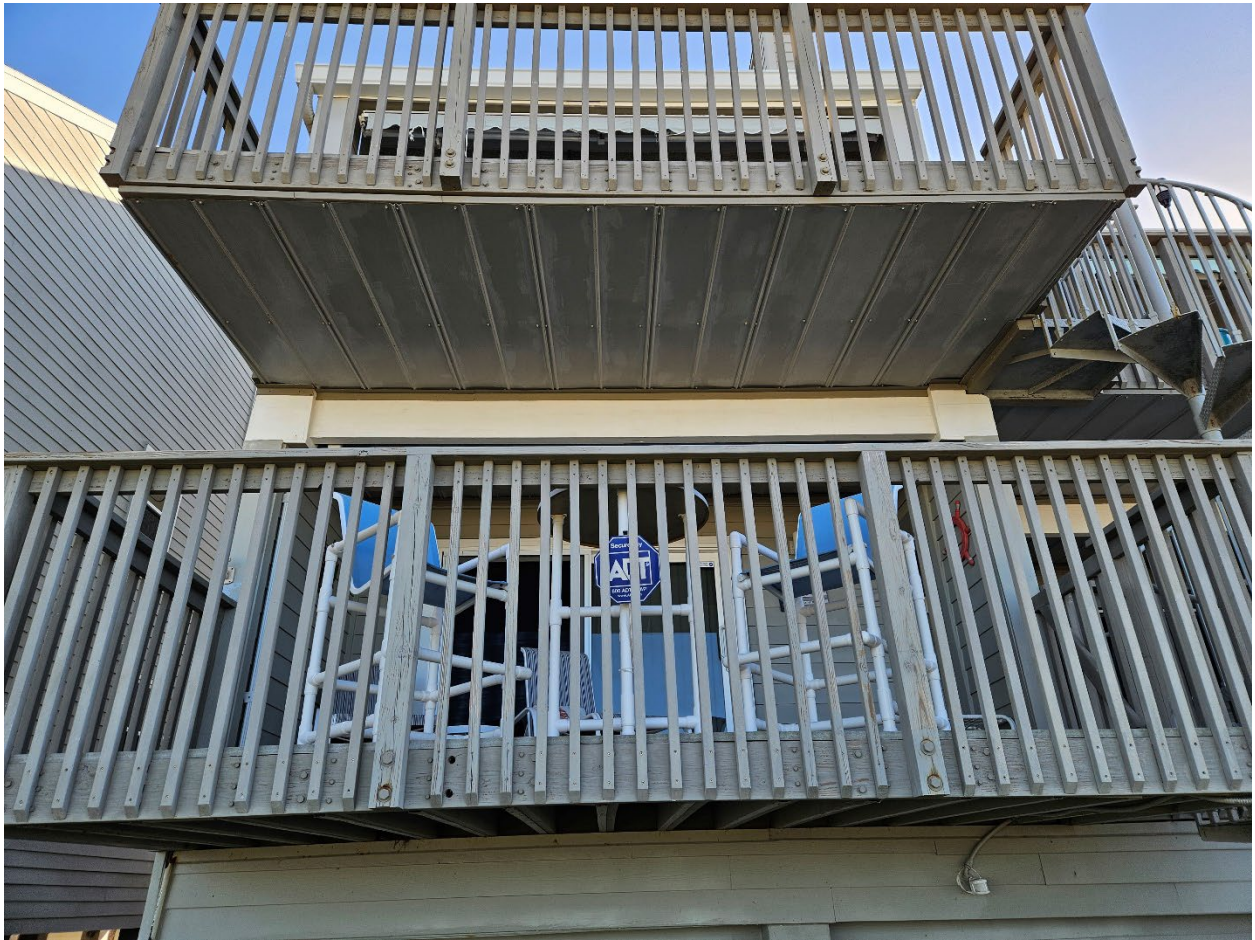
METAL PAN SHEETING - RECOMMEND REMOVING ALL LOCATIONS
