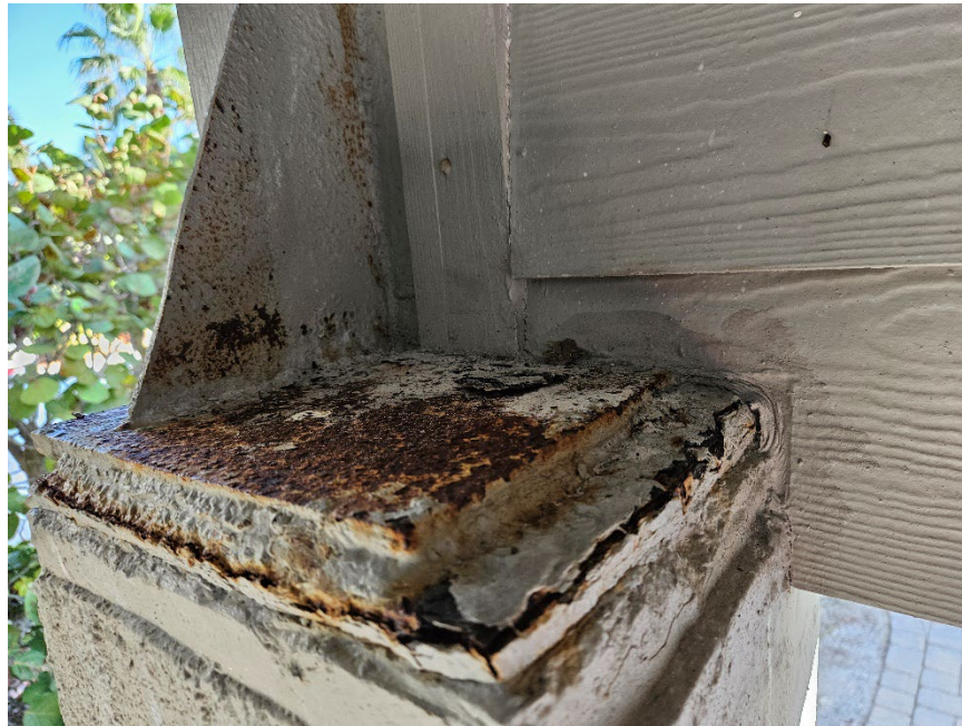
DAMAGED PLATE / BEAM CONNECTION
