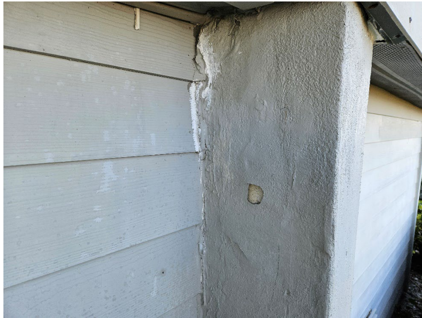
DELAMINATING STUCCO ON WEST SIDE OF BUILDING.
