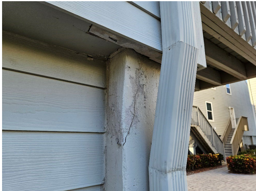
CONCRETE COLUMN DAMAGE
