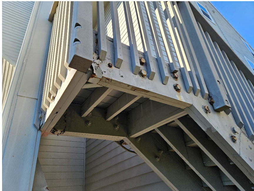
DAMAGED STAIR CONNECTIONS
