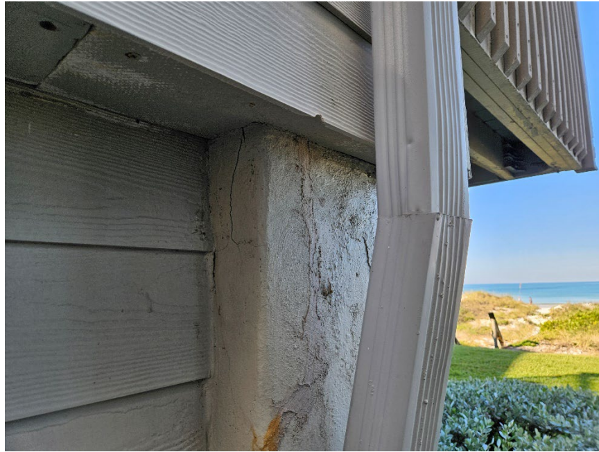
DAMAGE AND DELAMINATION AT NW COLUMN
