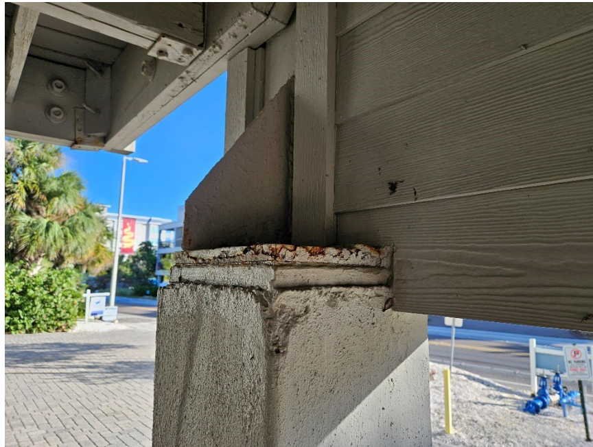
PLATE DAMAGE -BLDG #1
