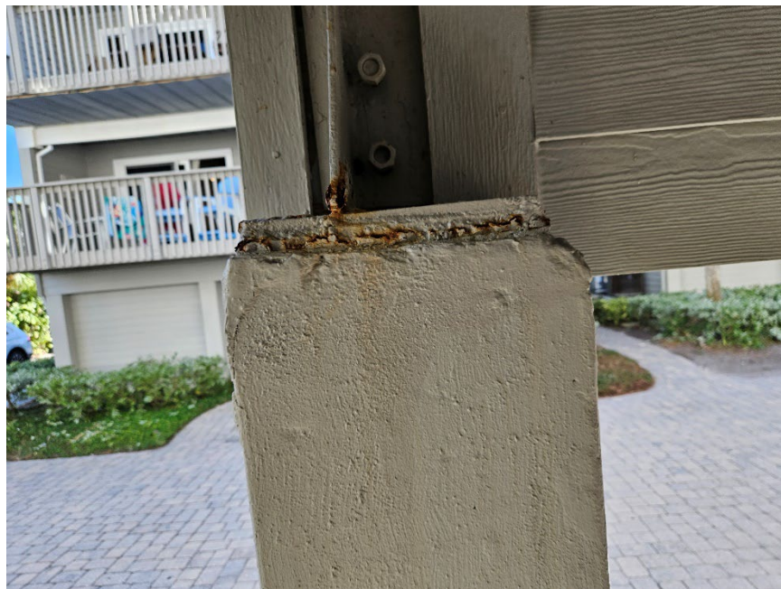
DAMAGED PLATE CONNECTION
