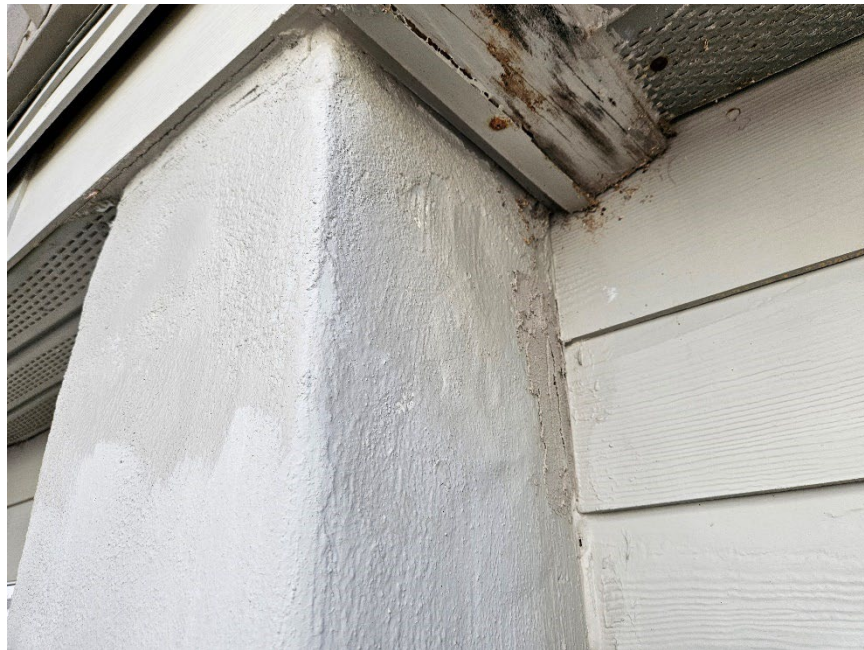
CONCRETE COLUMN PREVIOUSLY REPAIRED
