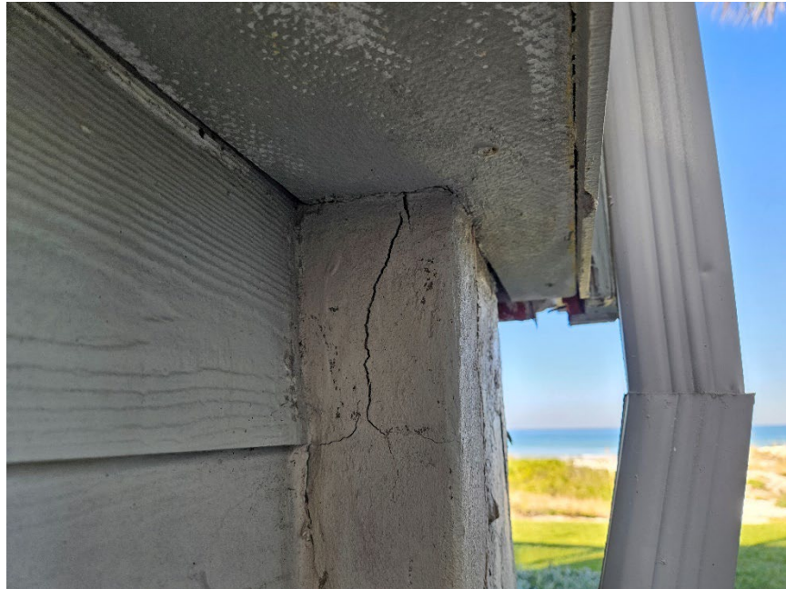
NW COLUMN DAMAGE
