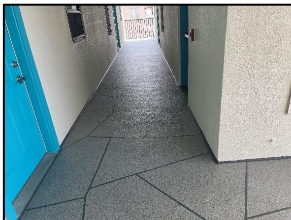
Fig.5 – Typical Gemstone Waterproofing Coating at Walkways.
