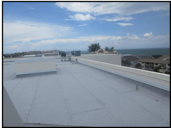
Fig.8 – Overview of New Modified Bitumen Roofing System.
