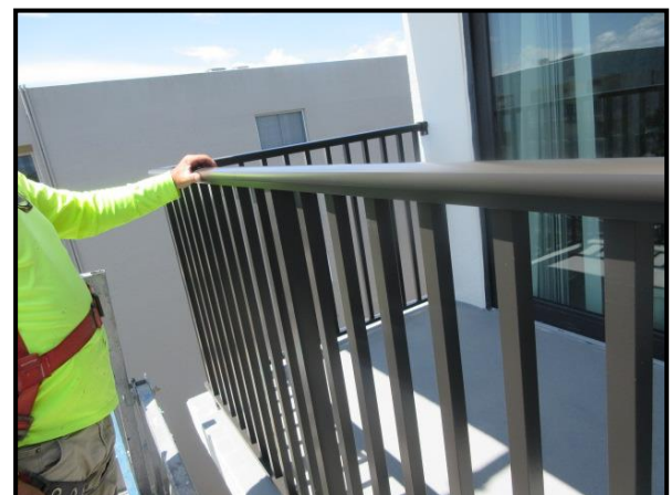
Fig.6 – New Railing System Installed at Balconies (42" Height – 4" Picket Spacing).
