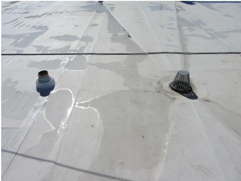
Photo #10 – Close Up Of Roof Drain and Vent Stack with TPO Boot.
