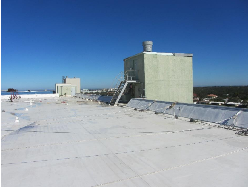
Photo #9 – Overview of TPO Roof, Has Been Installed for Approximately 2 Years.
