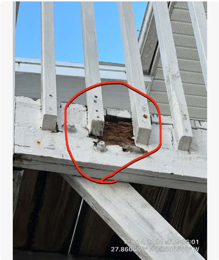
Unit 34, Center stairs. This location requires a repair to beam at top landing.
