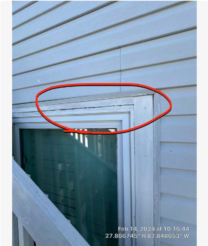
Open joints at window perimeter need resealing, located on the stairs to unit 10.
