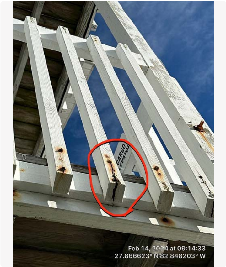
East stairs, South side of building. The wood framing is in fair condition. Rusting fasteners and split wood framing observed.
