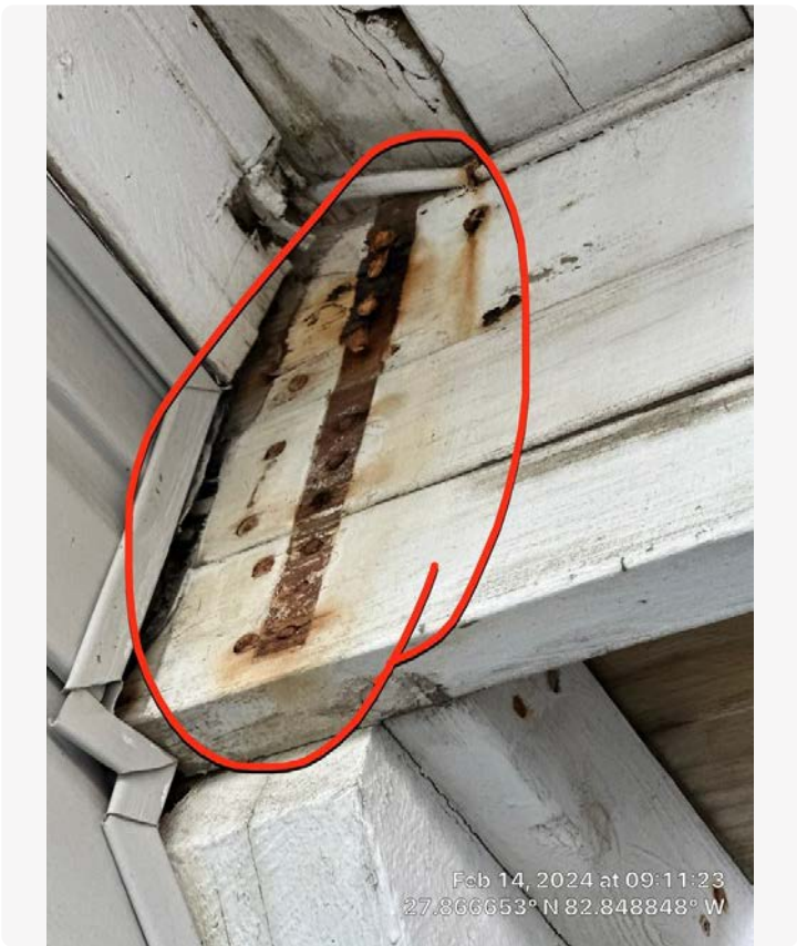
Rusting and missing fasteners West stairwell, North side of building. These locations will require repair and/or replacement of the fasteners.
