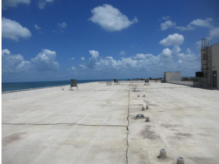
Photo #13 – Overview of Roof System - Modified Bitumen Coated with VFI Liquid Applied #990 Silicone.
