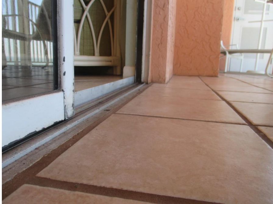
Photo #11 – SGD's Track Installed per Manufacturer's Recommendations. (TYP.)
