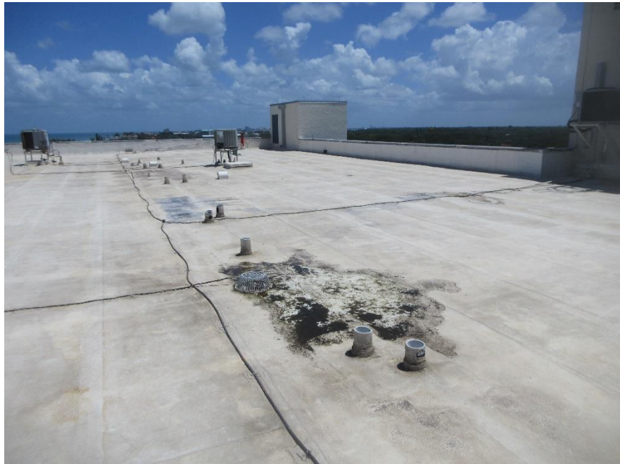
Photo #14 – Overview of Some Ponding Water Areas Observed at All Roof Levels.
