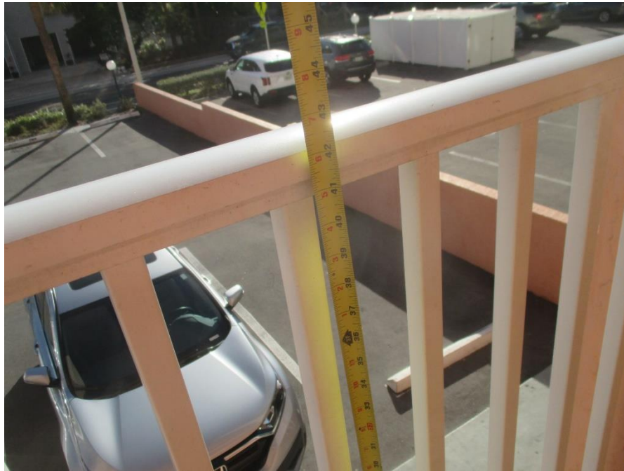
Photo #7 – Railing Height Appears to Be per Code ( \geq 42'' ).
