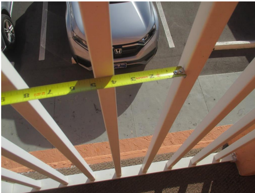
Photo #8 – Picket Spacing Appears to Be per Code ( \leq 4'' )
