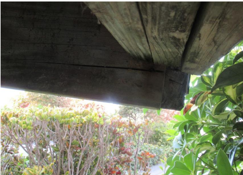
PHOTO 4: Observed cracked main perimeter carry beam.
