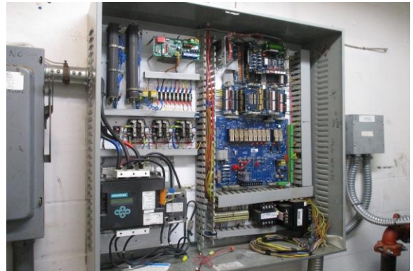
26 Elevator Control Board
