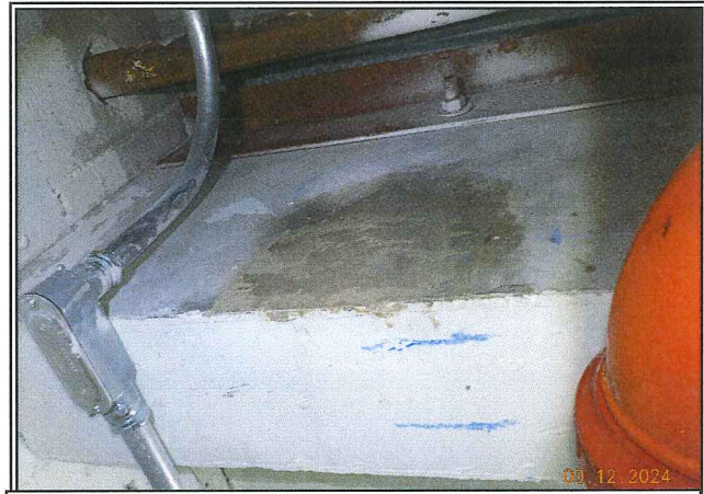
Area of Beam where Steel was Exposed; after Patching
