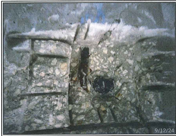
Area of Beam where Steel was Exposed
